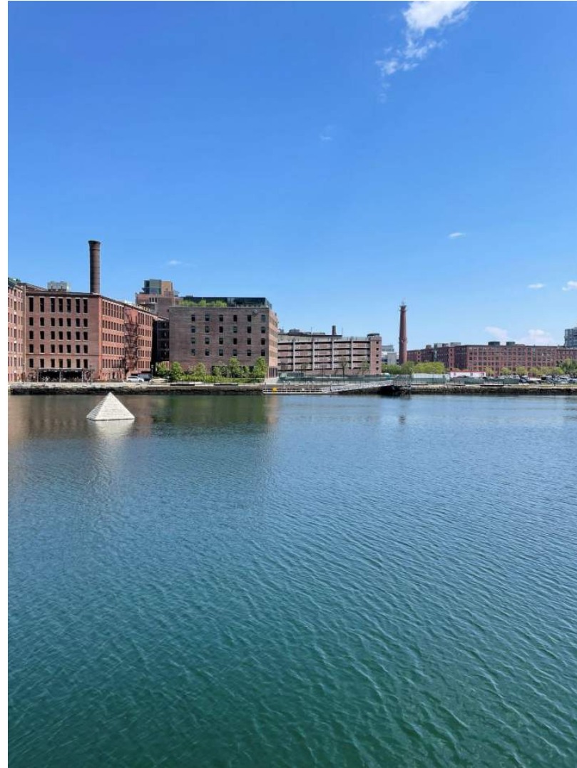
Proposed Location View from Summer Street Bridge
