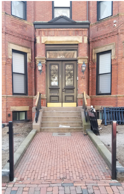
Main Brick Walk and Front Stoop
