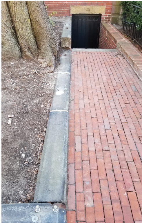
Side Brick Walk to Basement
