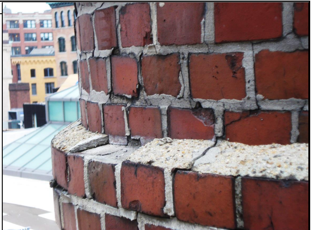
Deteriorated Wash and Bricks at Top of Stack
