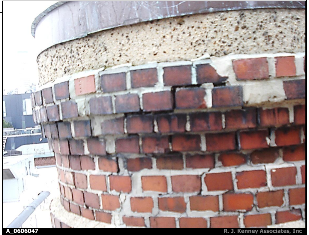
Top of Stack Cracked and Displaced
