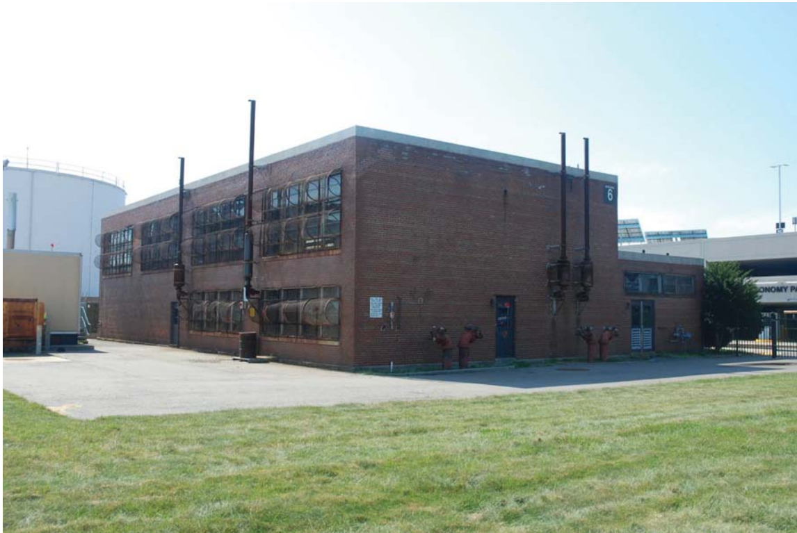
6. Former Logan Airport Water Pumping Station, 161 Prescott Street, Boston, MA. View of rear (E) and north elevations, photographer facing SW, August 2019.
