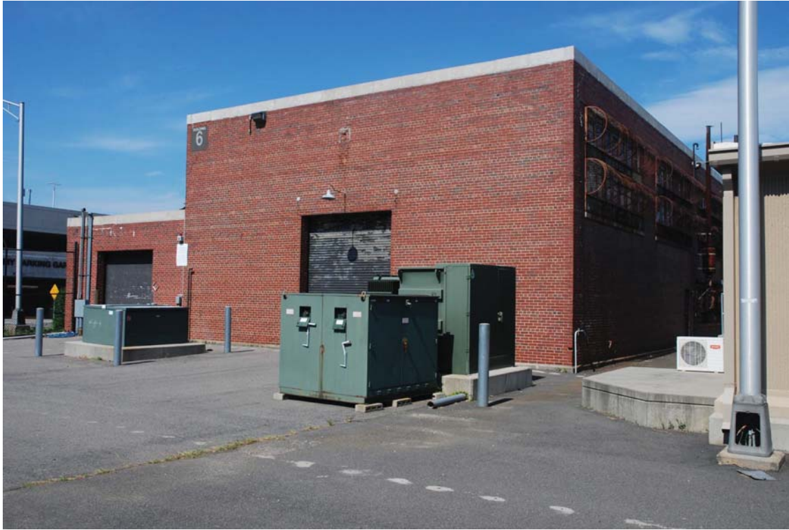
5. Former Logan Airport Water Pumping Station, 161 Prescott Street, Boston, MA. View of S elevation, photographer facing NW, August 2019.
