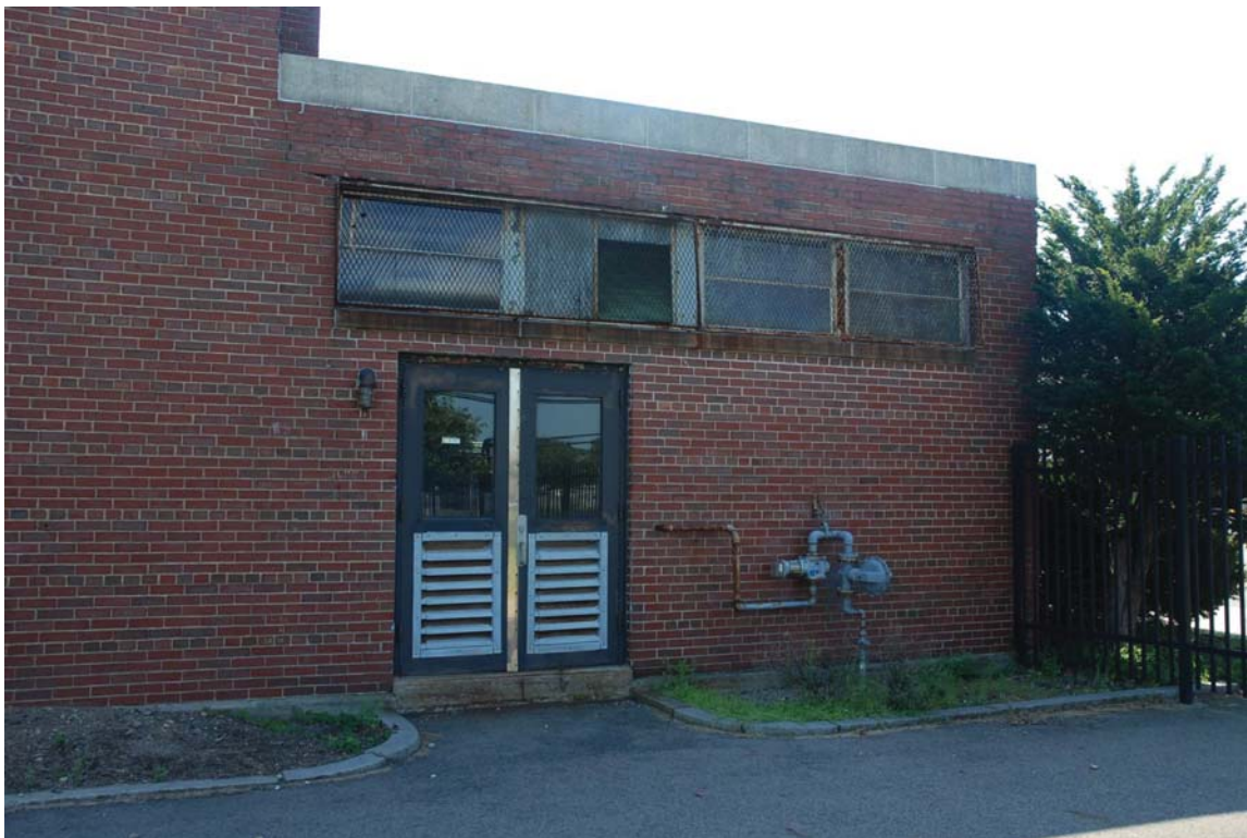
8. Former Logan Airport Pumping Station, 161 Prescott Street, Boston, MA. View of N elevation, entrance detail, photographer facing S, August 2019.
