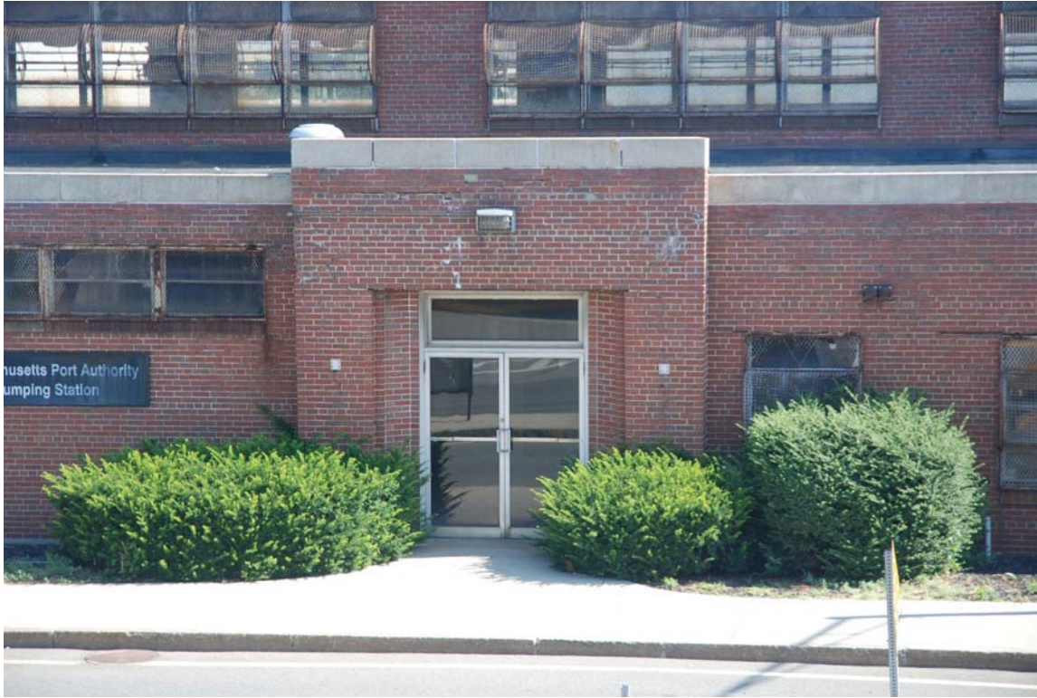
3. Former Logan Airport Water Pumping Station, 161 Prescott Street, Boston, MA. View of front (W) elevation, main entrance detail, photographer facing E, August 2019.
