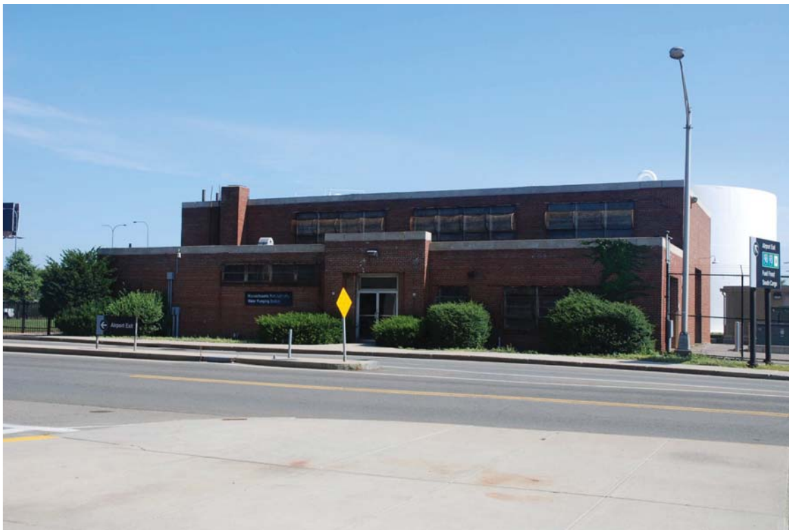
2. Former Logan Airport Water Pumping Station, 161 Prescott Street, Boston, MA. View of front (W) elevation, photographer facing E, August 2019.
