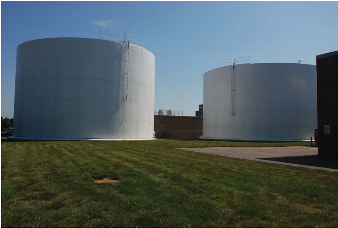
9. Project parcel, 161 Prescott Street, Boston, MA. View of reservoir water tanks on the east side of the Logan Airport Pumping Station, photographer facing E, August 2019.
