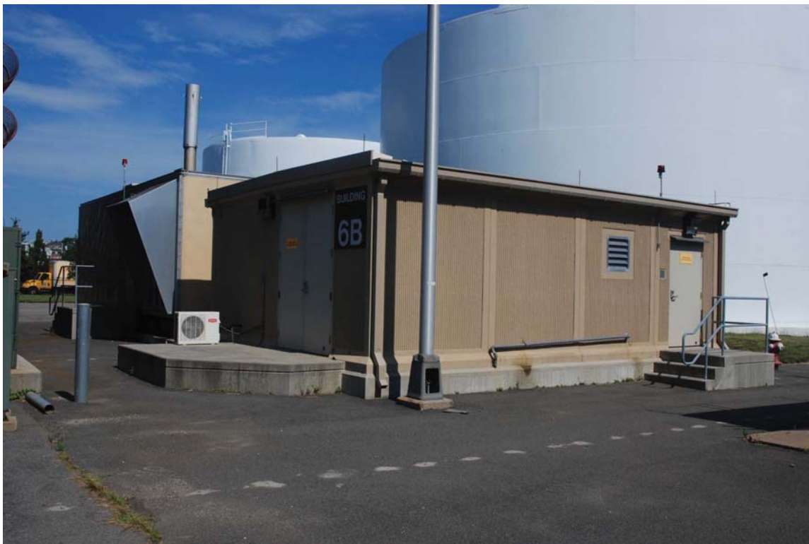
10. Project parcel, 161 Prescott Street, Boston, MA. View of electrical communications building and backup generator, photographer facing NW, August 2019.
