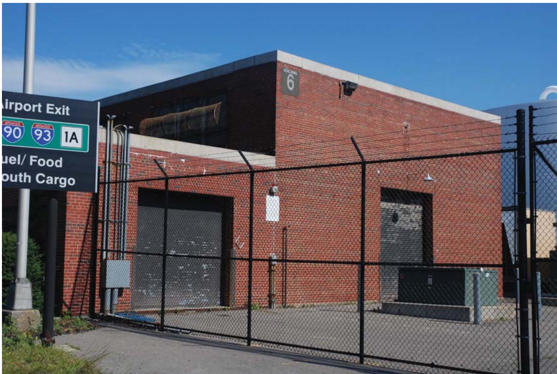
4. Former Logan Airport Water Pumping Station, 161 Prescott Street, Boston, MA. View of S elevation, photographer facing NE, August 2019.
