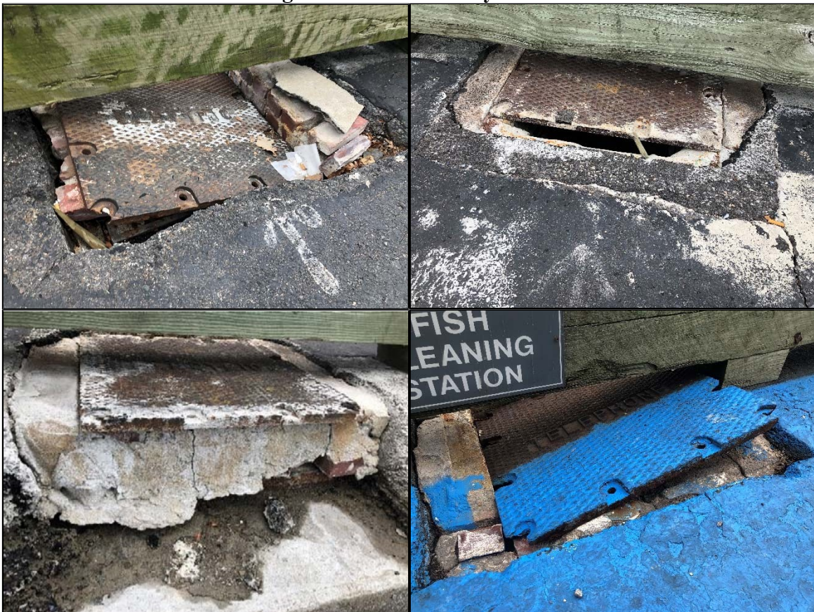
Below: Existing Conditions of Utility Access Hand-Hole
