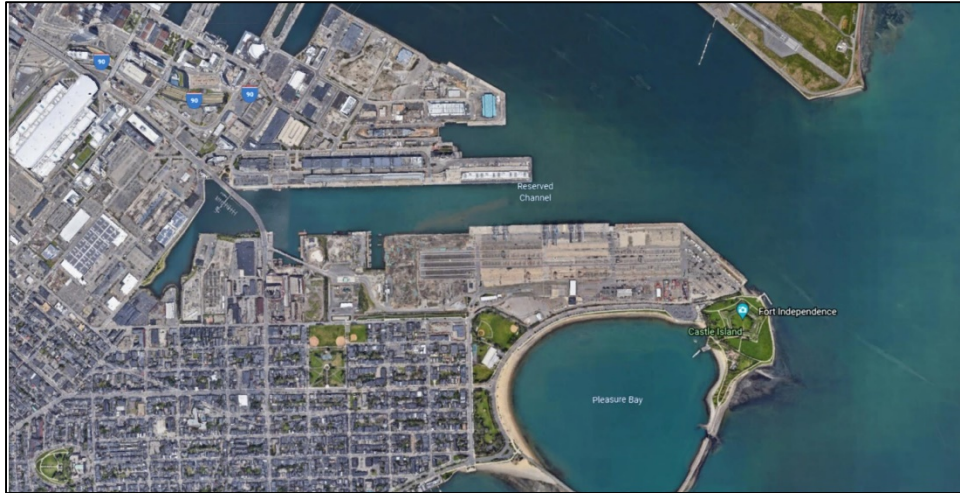
Site Overview (Image Source: Google Earth)
