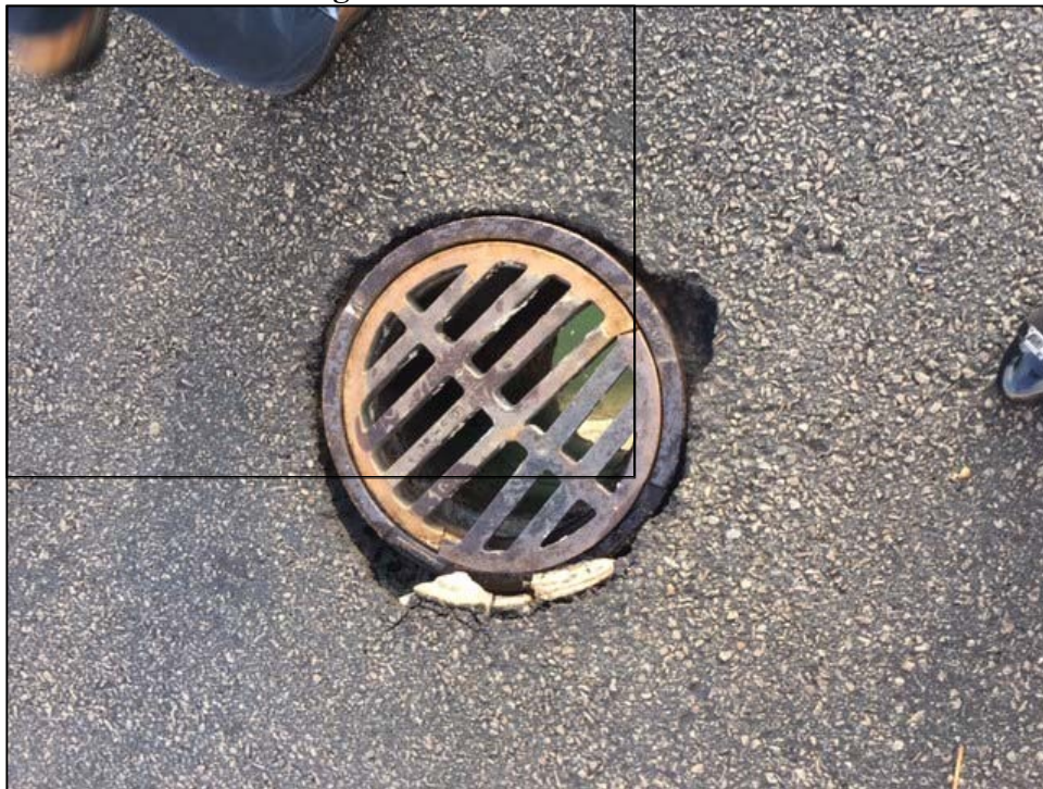
Above: Heaved Pavement Section Below: Drainage Hole within Heaved Pavement Section
