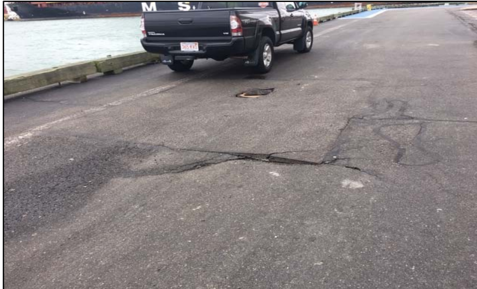
Above: Heaved Pavement Section Below: Drainage Hole within Heaved Pavement Section
