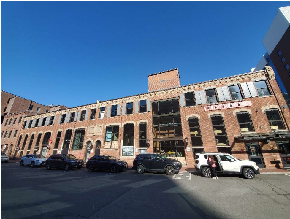
1. General view of 44 Thomson Place looking West.
