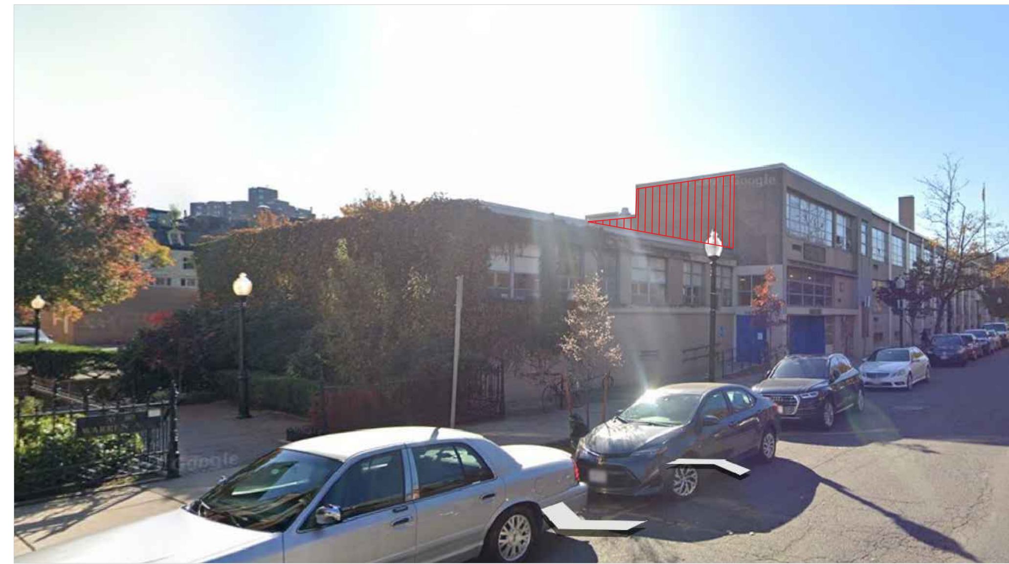
2 STREET VIEW FROM NORTHEAST ( WARREN AVE)
