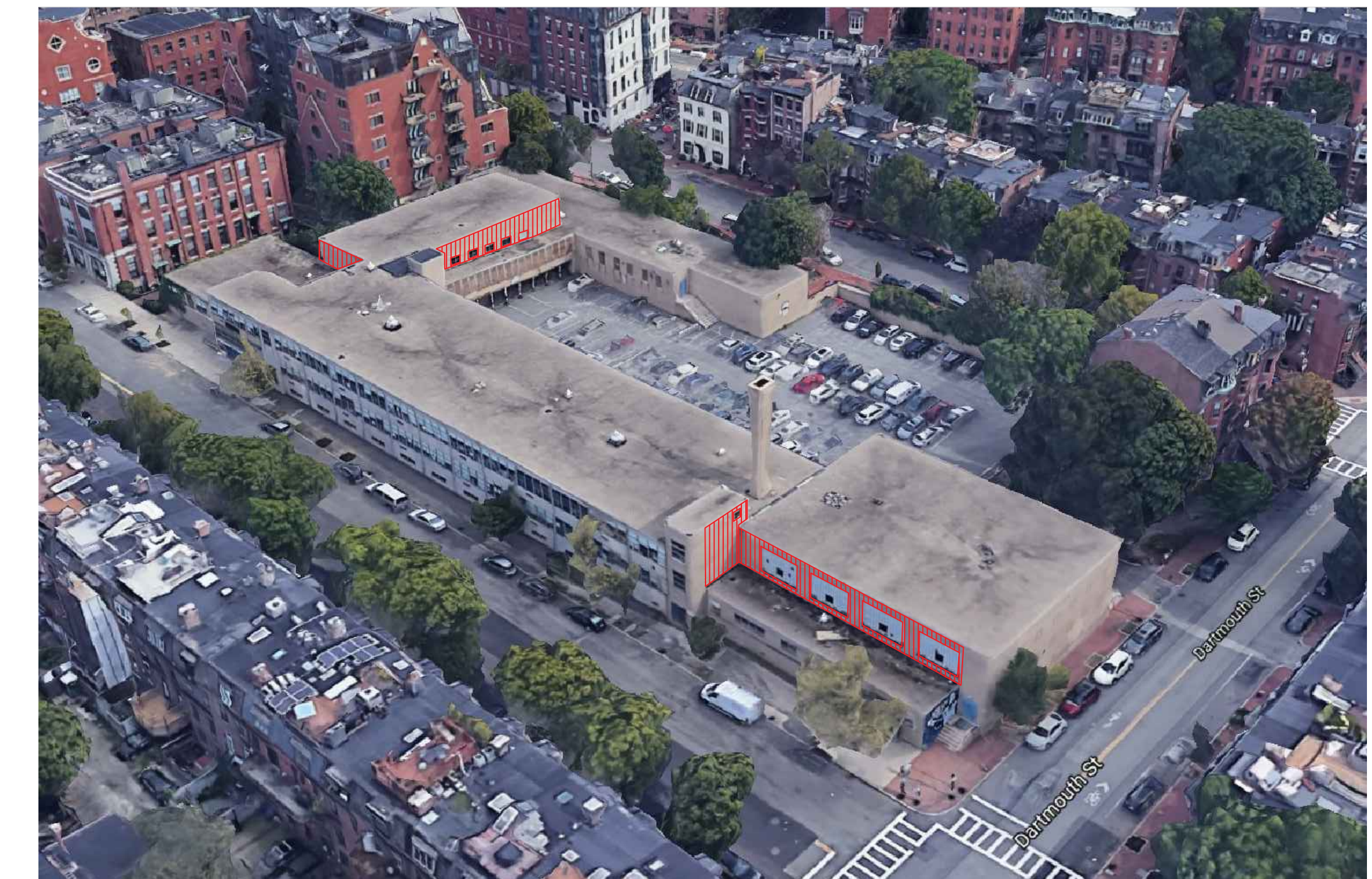
7 AERIAL VIEW FROM NORTHWEST (WARREN AVE & DARTMOUTH ST)
