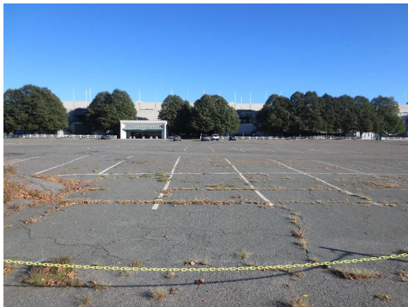
View of grandstand building from surface parking lot in one of the locations where surcharging is proposed; grandstand building to remain
