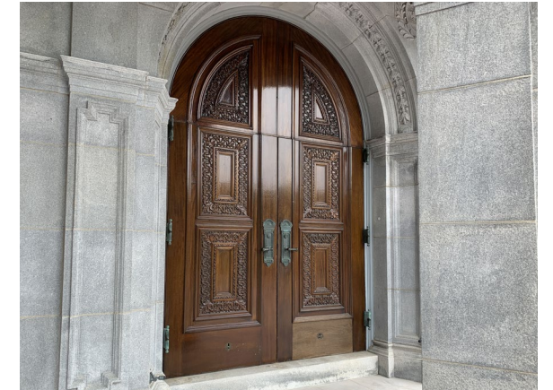
Existing Wood Doors at Vestibule
