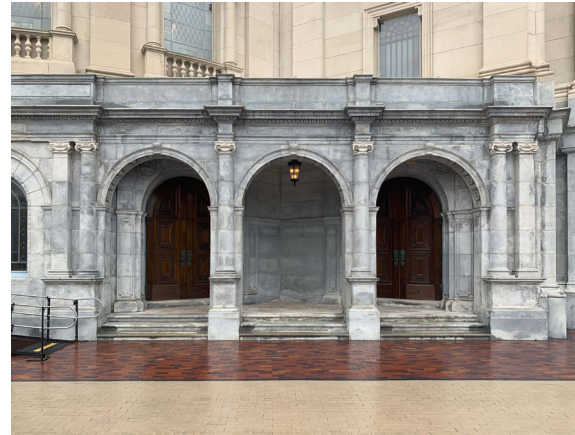
Proposed Elevator – left, Existing Vestibule – right
