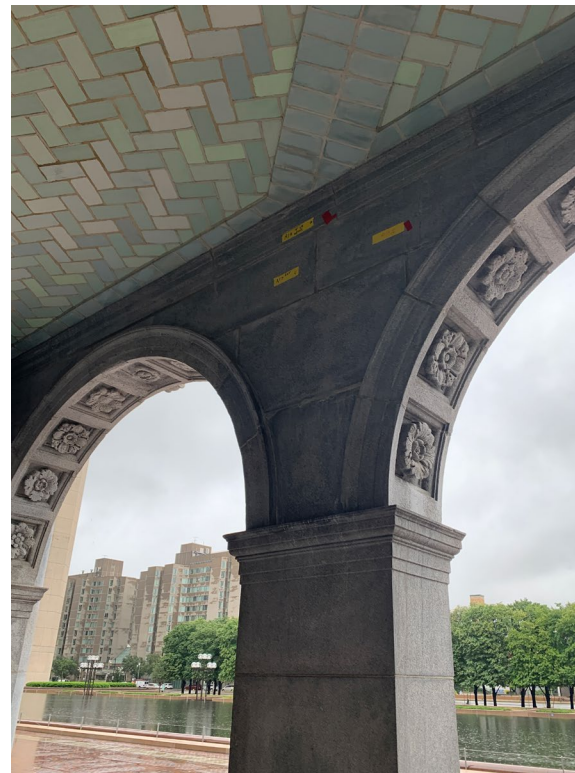
Stone Detail and Guastavino Tiled Ceiling
