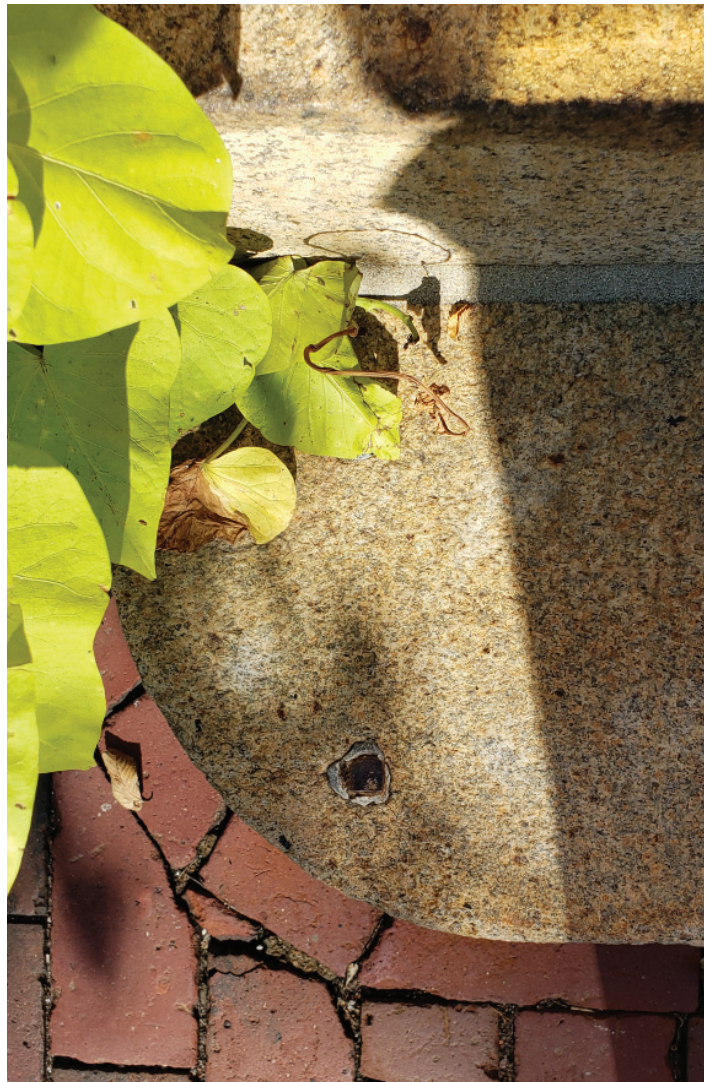
EXIST STAIRS - IRON POST CUT OFF
