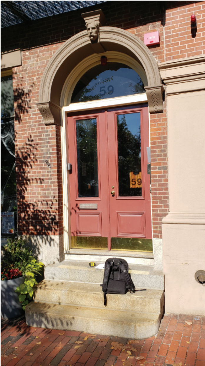
EXISTING STAIRS - FRONT
