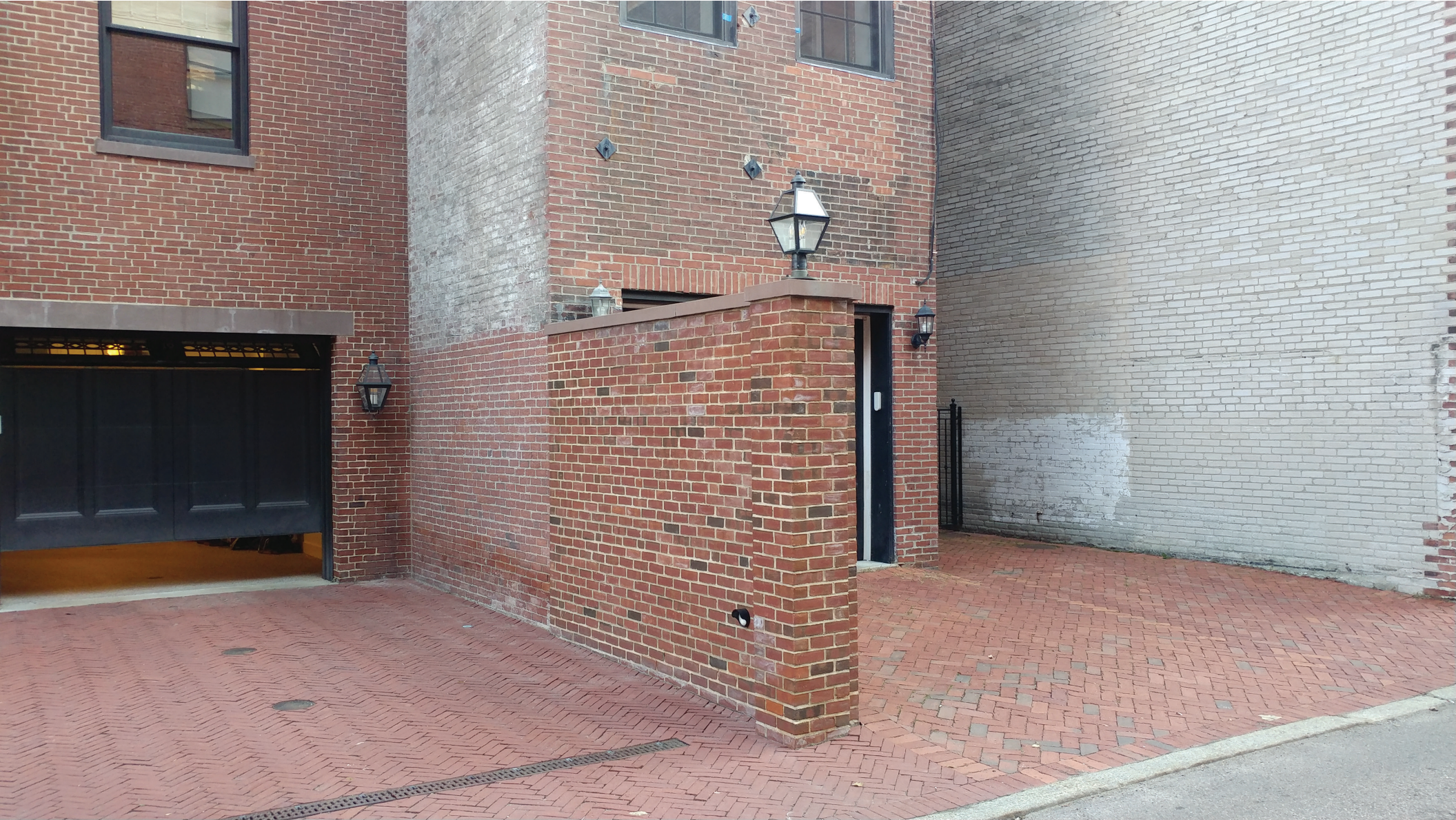
REAR WALL @ EAST PROPERTY LINE / GARAGE DOOR
