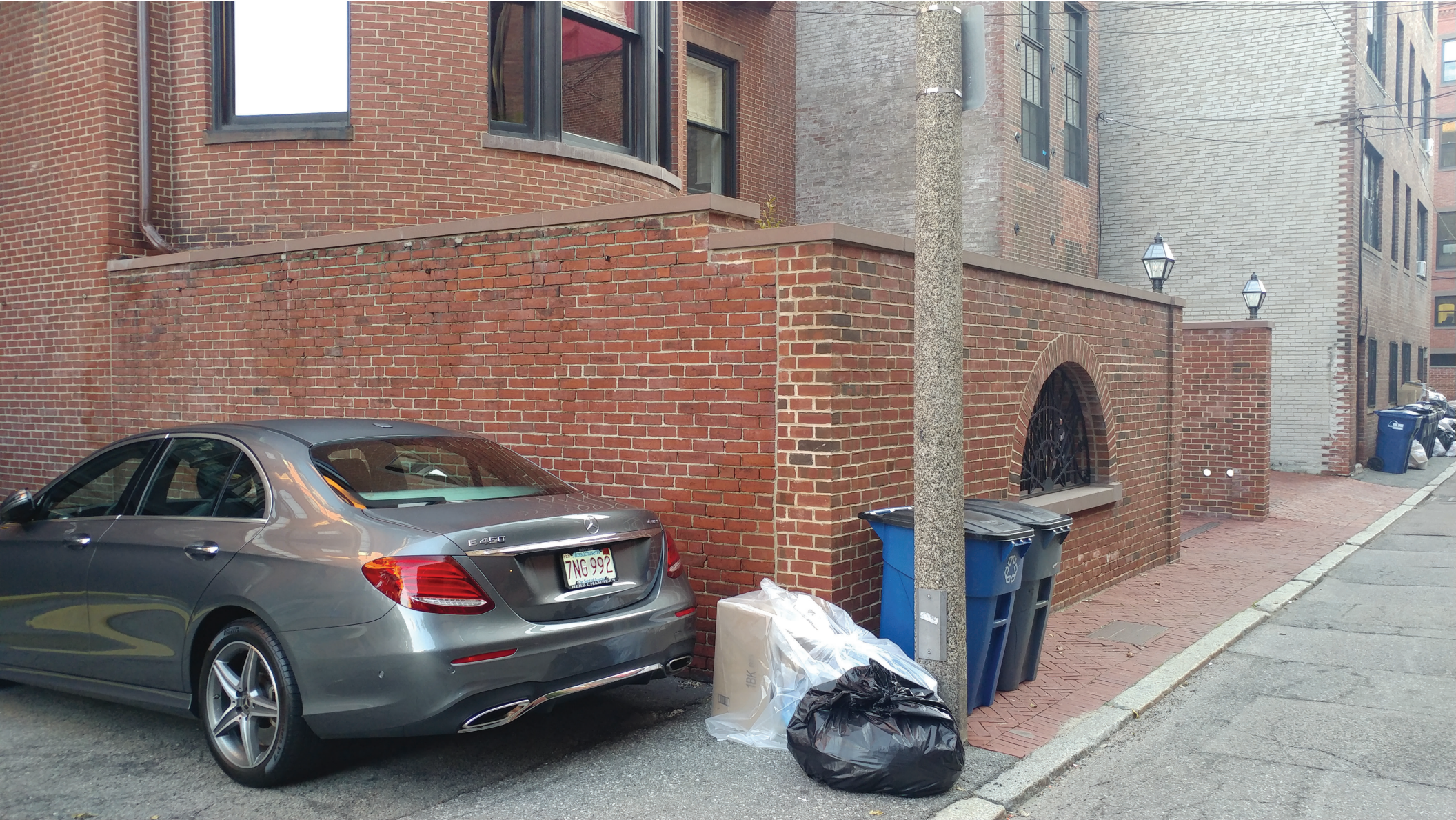
REAR WALL LOOKING EAST & #12 PARKING AREA
