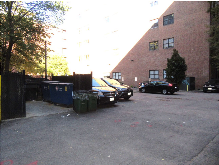
4. 11 Sleeper Street parcel, transformer at far right, view northwest
