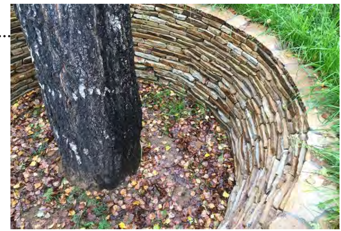
Retaining Wall to Protect Tree
