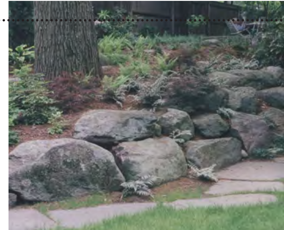
Boulder Retaining Walls
