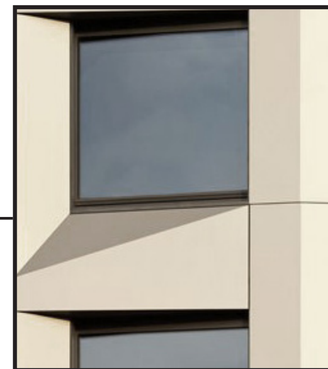
METAL PANEL CLADDING
