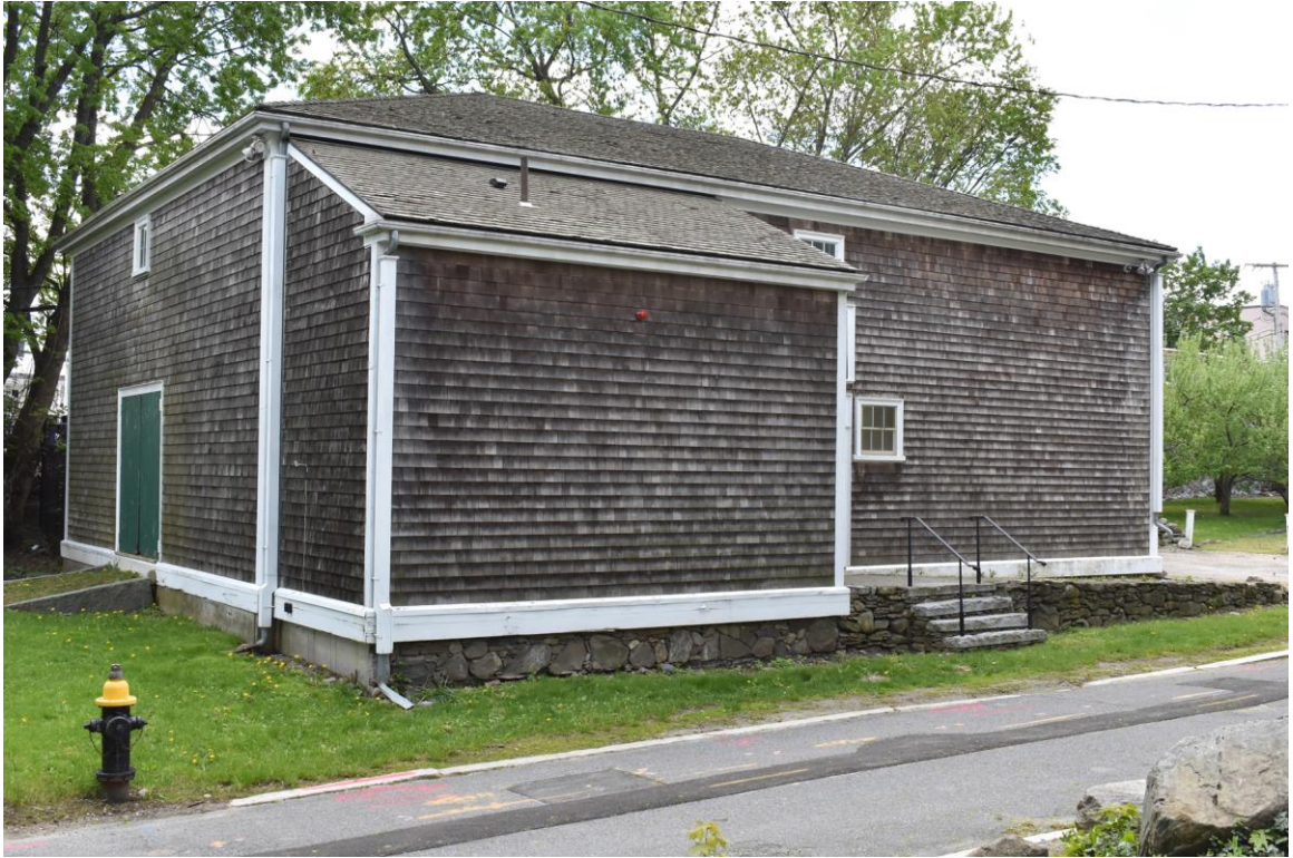
Photo 25. Ingersoll-Gardner Carriage House, northeast and northwest elevations.
