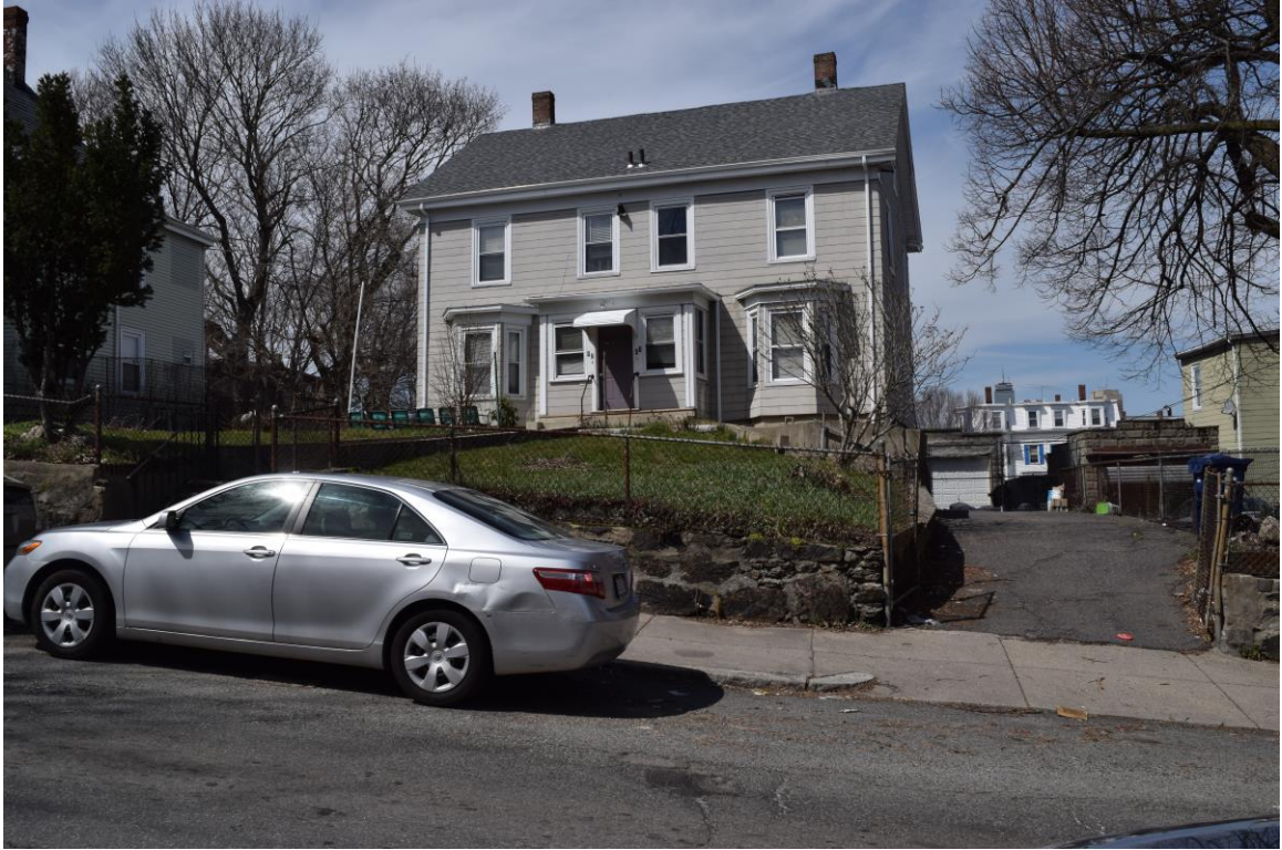
Photo 16. 42–44 Shirley Street, front (southeast) and side (northeast) elevations.
