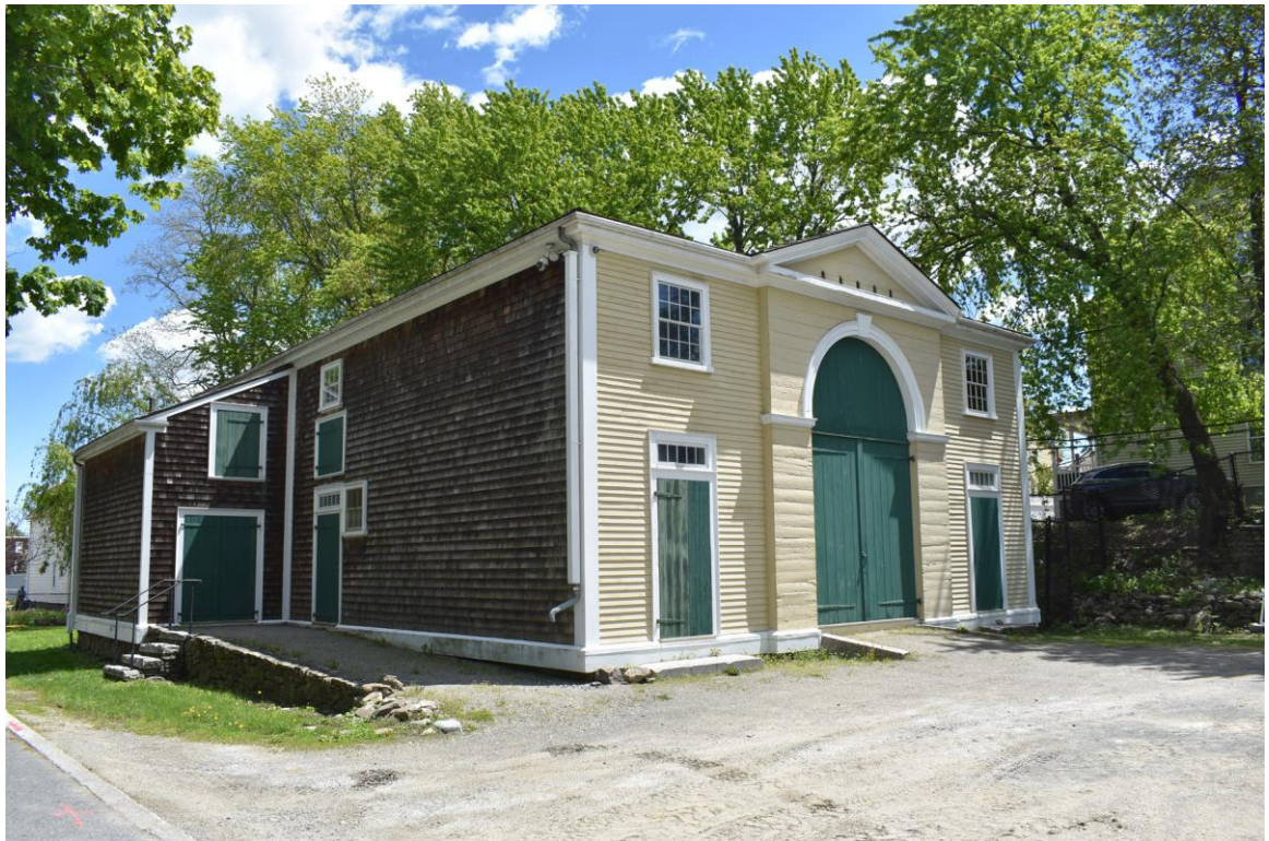
Photo 24. Ingersoll-Gardner Carriage House, front (southwest) and northwest elevations.
