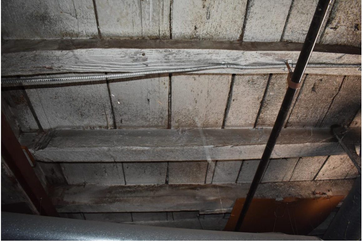
Photo 21. 44 Shirley Street interior, basement, showing lime washed ceiling framing.
