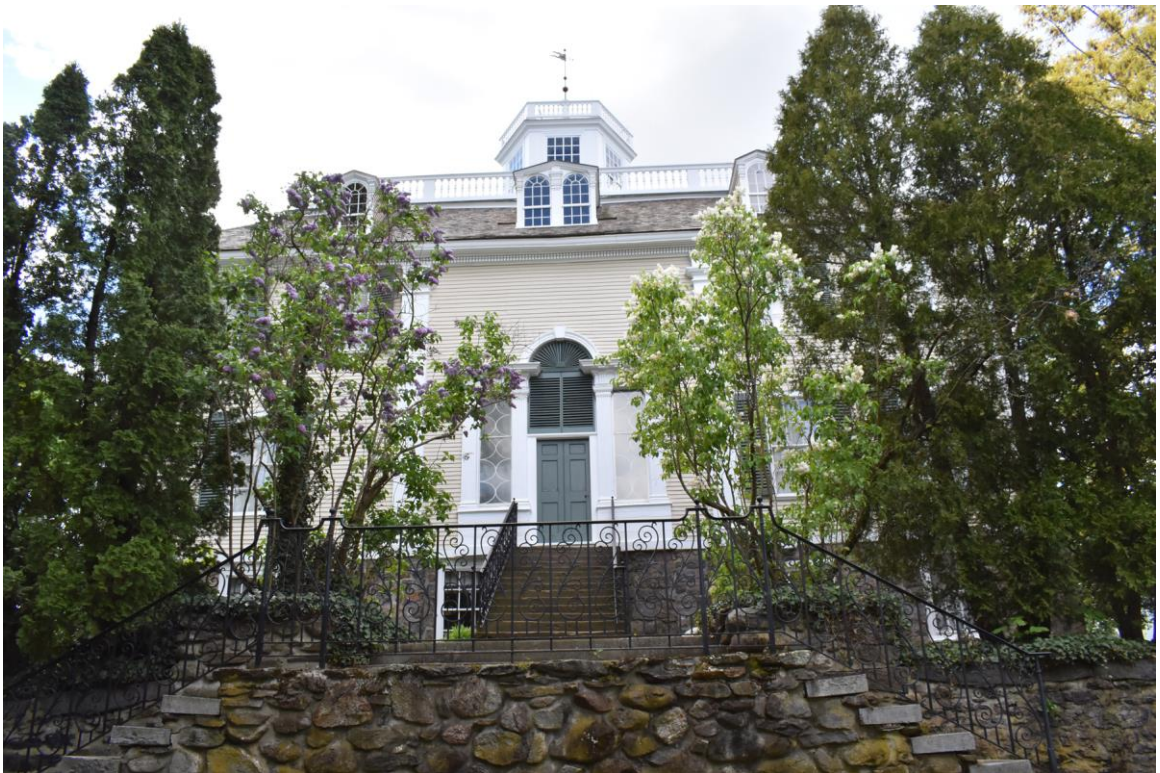
Photo 12. Shirley-Eustis House, rear (northeast) elevation.
