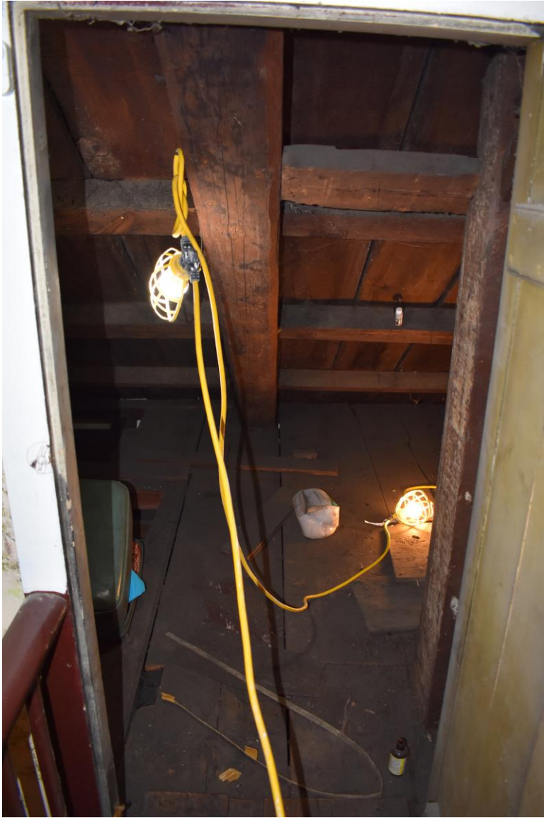
Photo 20. 42 Shirley Street interior, attic framing.
