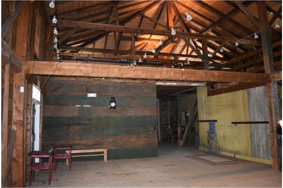
Photo 27. Ingersoll-Gardner Carriage House interior, first story.
