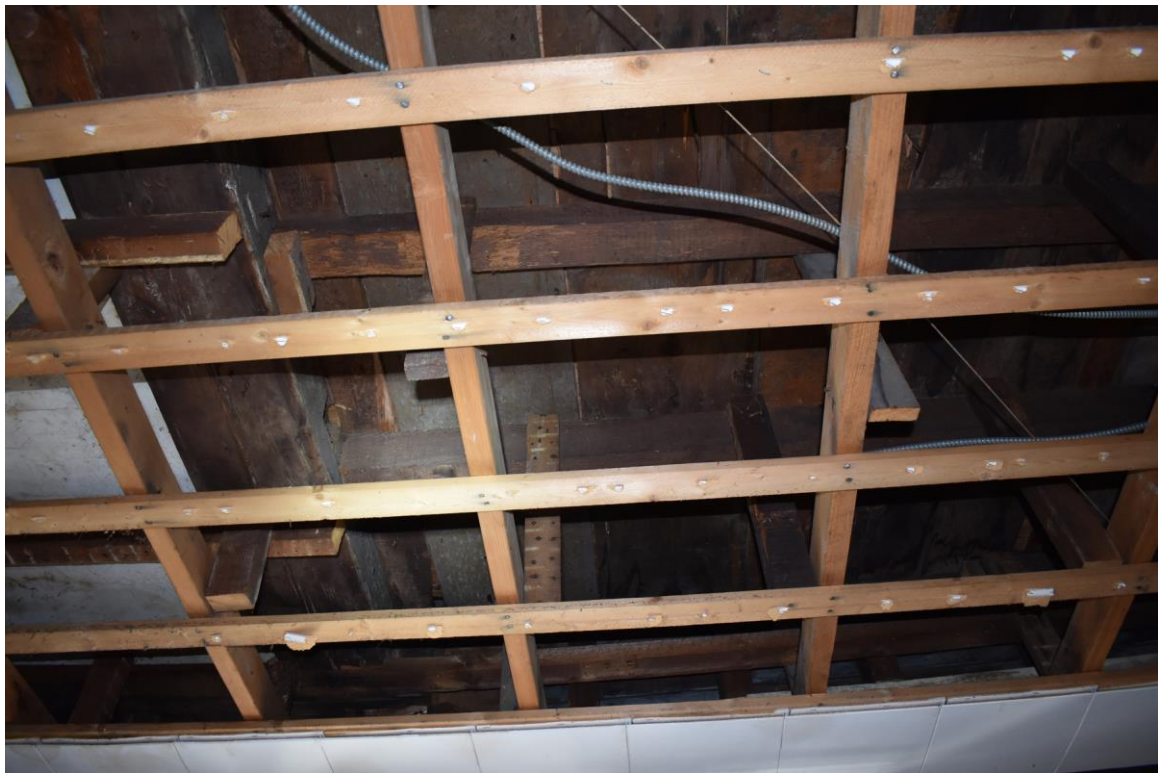
Photo 19. 42 Shirley Street interior, first floor ceiling framing and plaster (at left).
