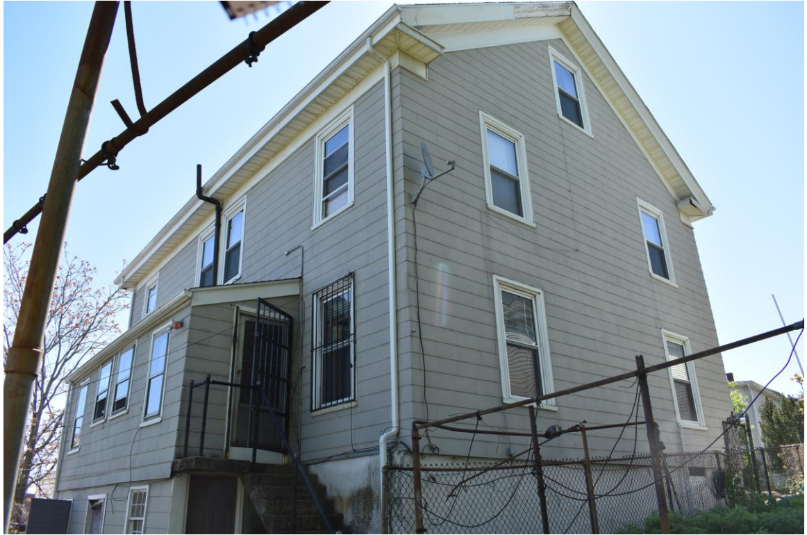
Photo 18. 42–44 Shirley Street, rear (northwest) and southwest elevation.
