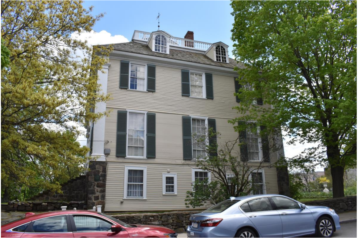
Photo 11. Shirley-Eustis House, northwest elevation.
