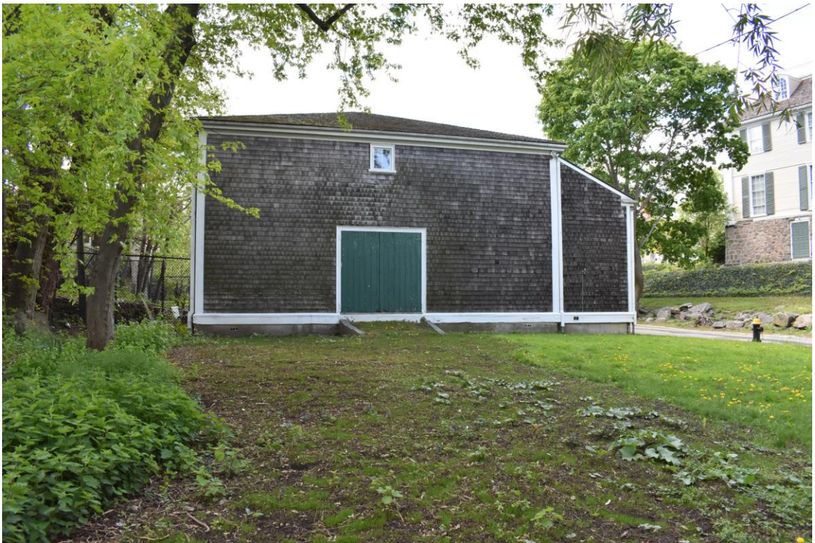
Photo 26. Ingersoll-Gardner Carriage House, rear (northeast) elevation.
