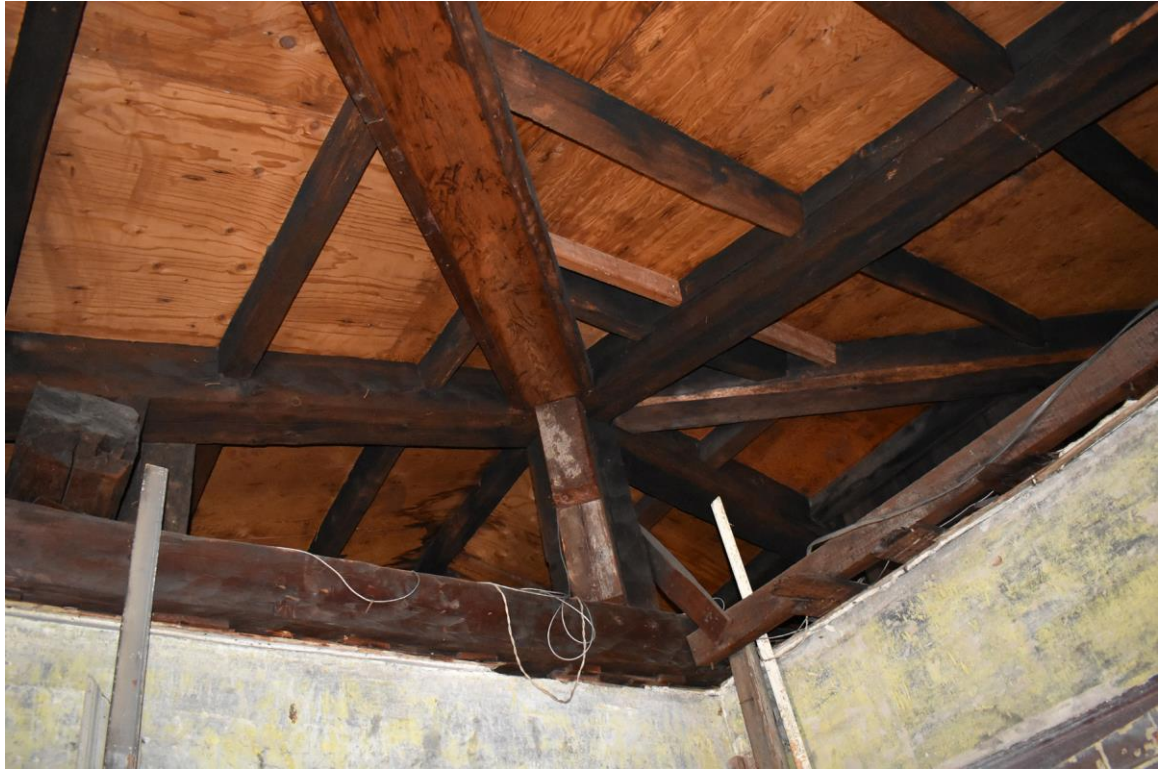
Photo 13. Shirley-Eustis House interior, roof framing.
