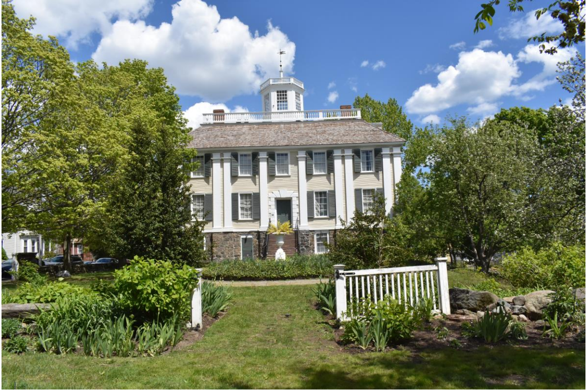
Photo 9. Shirley-Eustis House and Grounds, looking northeast at the front (southwest) façade.
