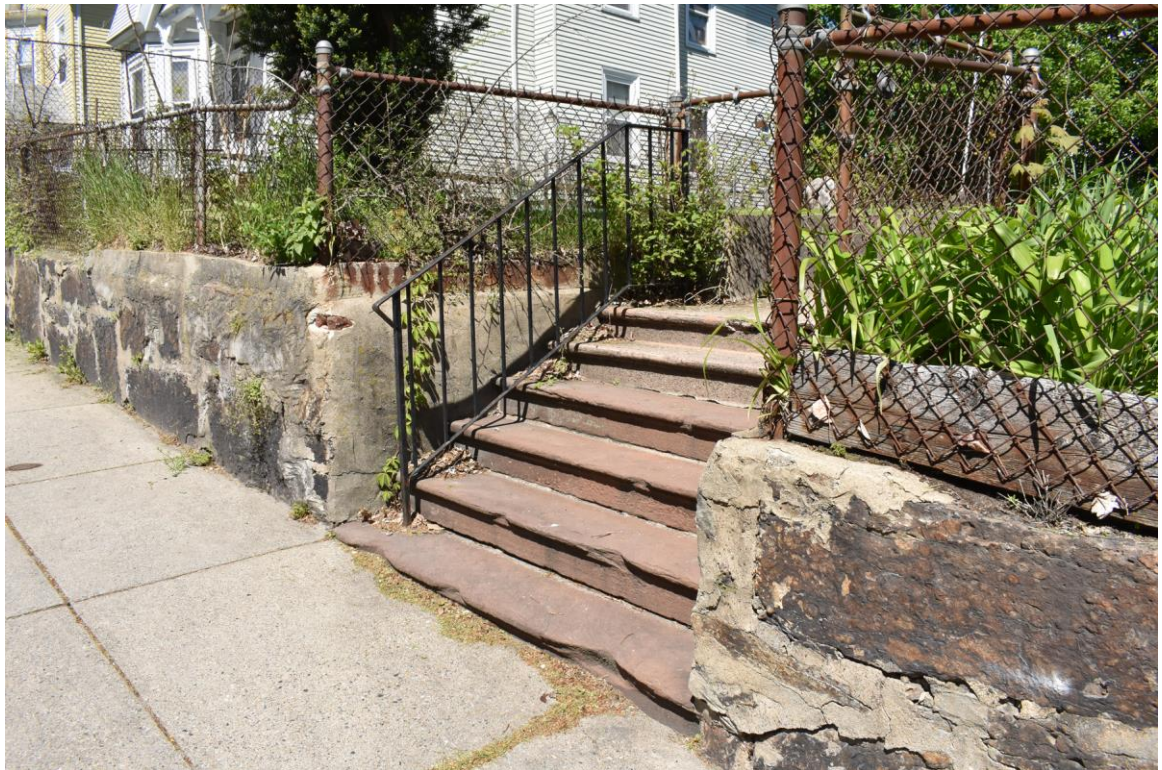
Photo 6. 42-44 Shirley Street, retaining wall and brownstone stairs, looking northwest.
