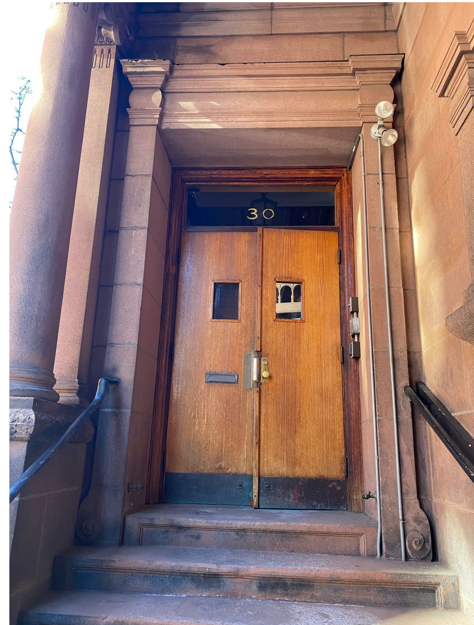
VIEW OF 30 FAIRFIELD STREET ENTRANCE PORCH WITH FLUSH WOOD EXTERIOR DOORS
