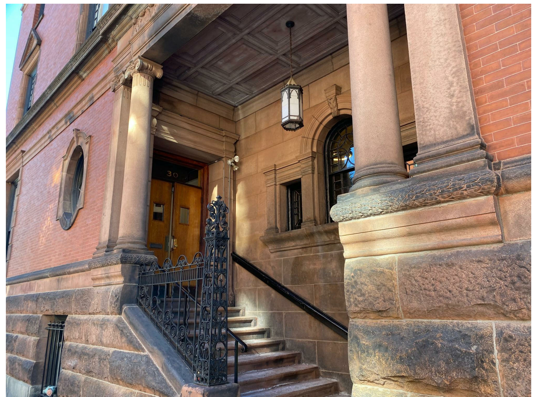
VIEW OF 30 FAIRFIELD STREET ENTRANCE PORCH WITH FLUSH WOOD EXTERIOR DOORS
