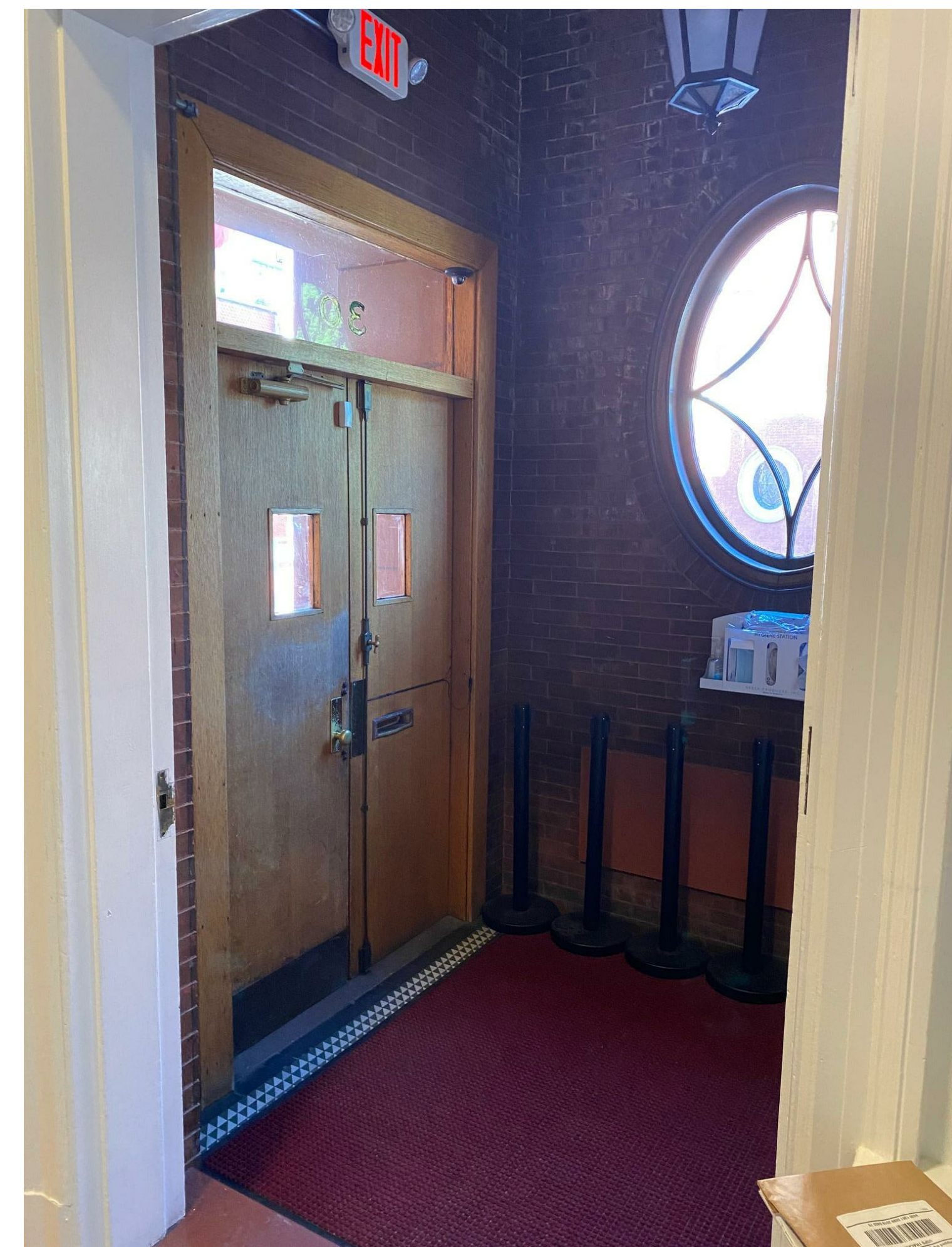
VIEW OF 30 FAIRFIELD STREET ENTRANCE VESTIBULE WITH FLUSH WOOD EXTERIOR DOORS
