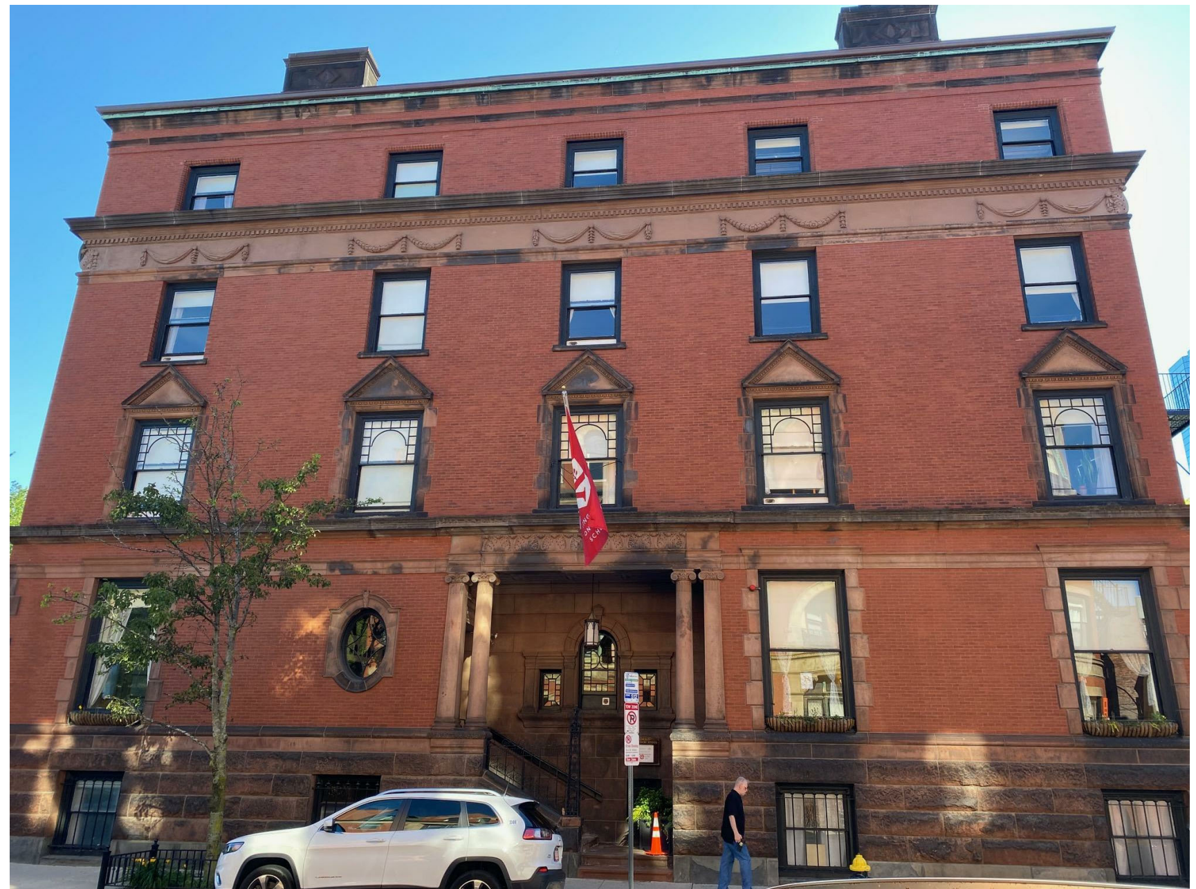
VIEW OF 30 FAIRFIELD STREET WITH ENTRANCE PORCH
