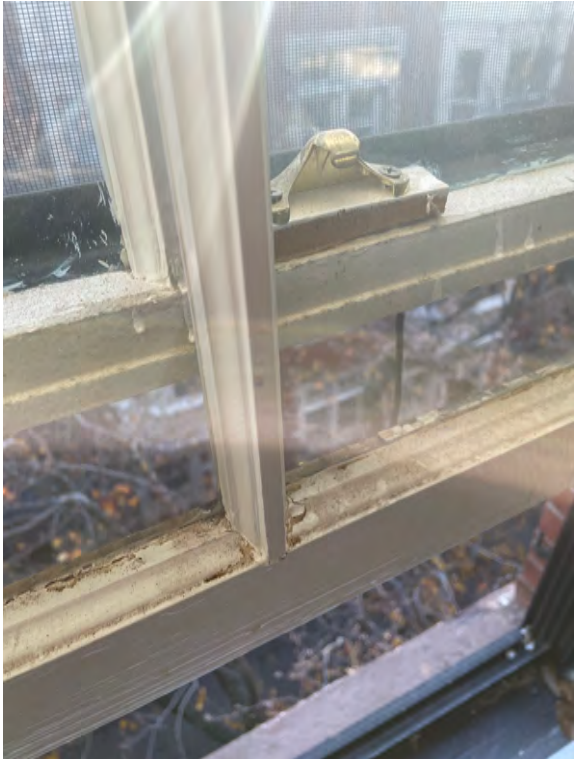
Example of 4 th floor replacement window sash
