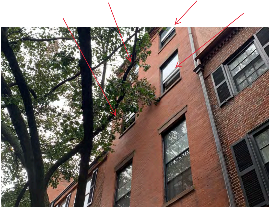
Front side of building (Pinckney Street) looking up at 3rd & 4th Floors with 2nd floor (not our unit) in bottom of picture.
