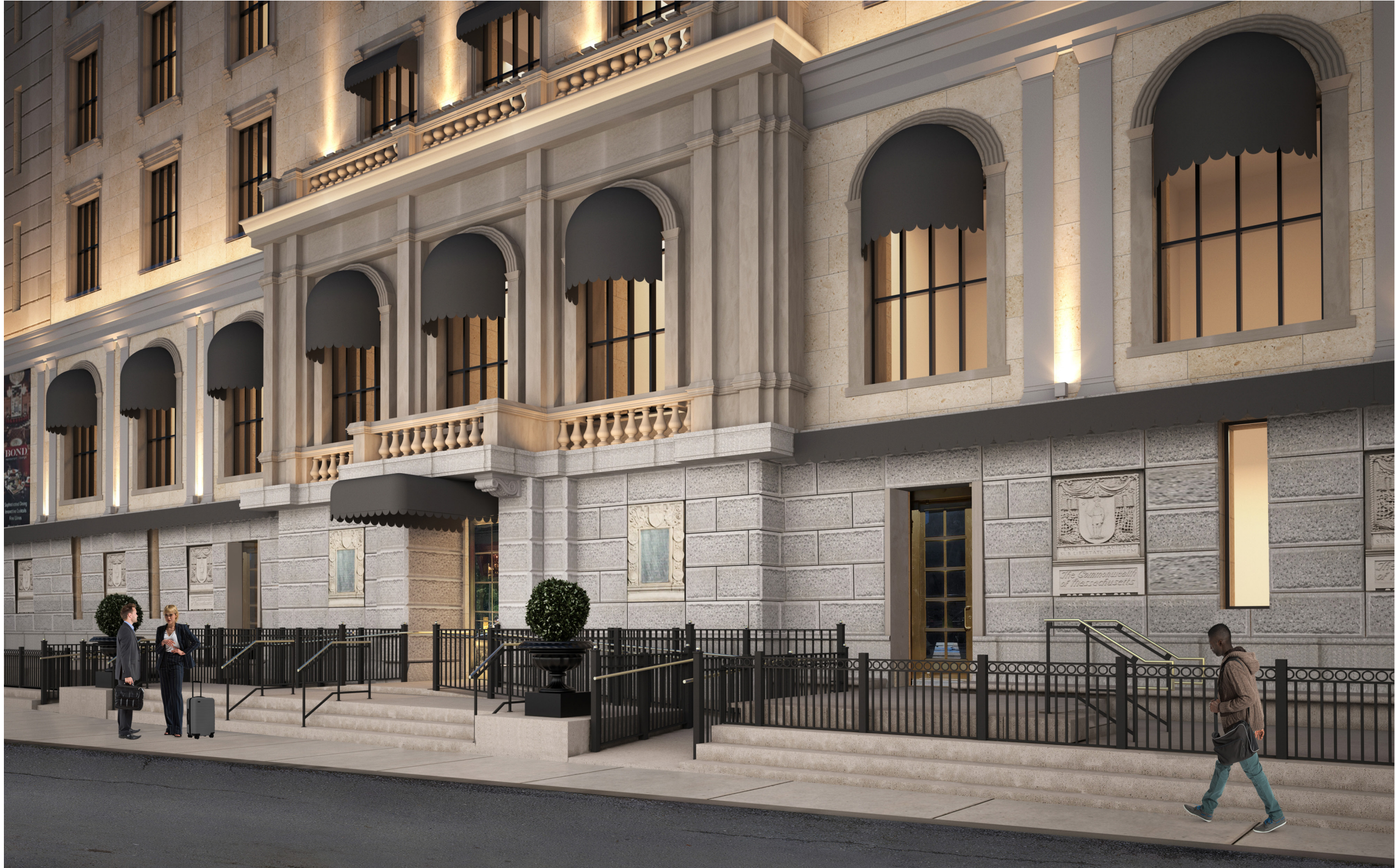
NEW PEARL STREET ENTRANCE WITH HANDRAILS AND RAMPS - STREET VIEW (PLANTERS NOT SHOWN)
