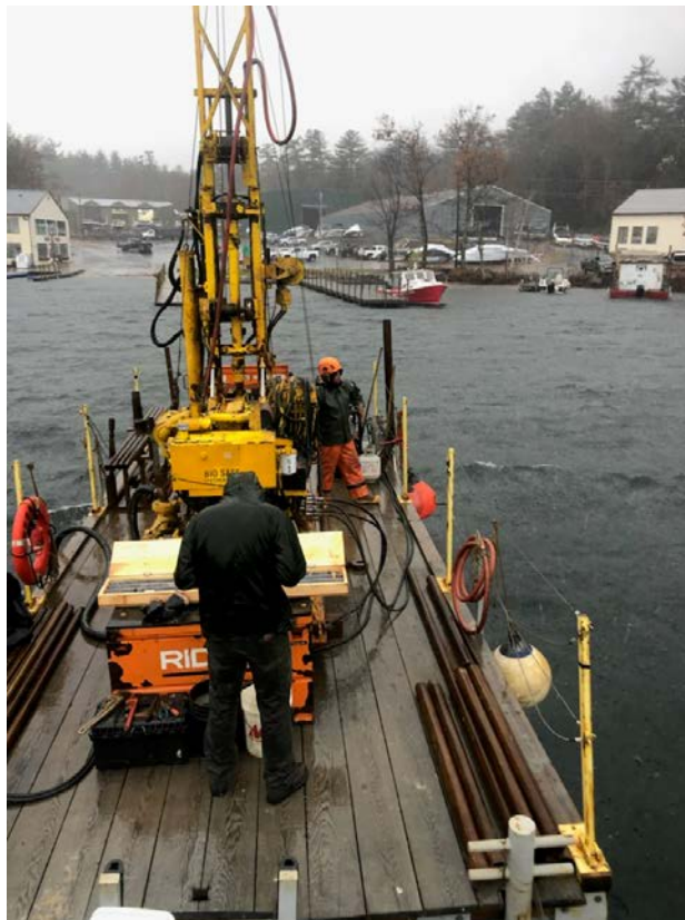
Photo 6: View of representative barge and equipment to be used during the in-water portion of the geotechnical work.
