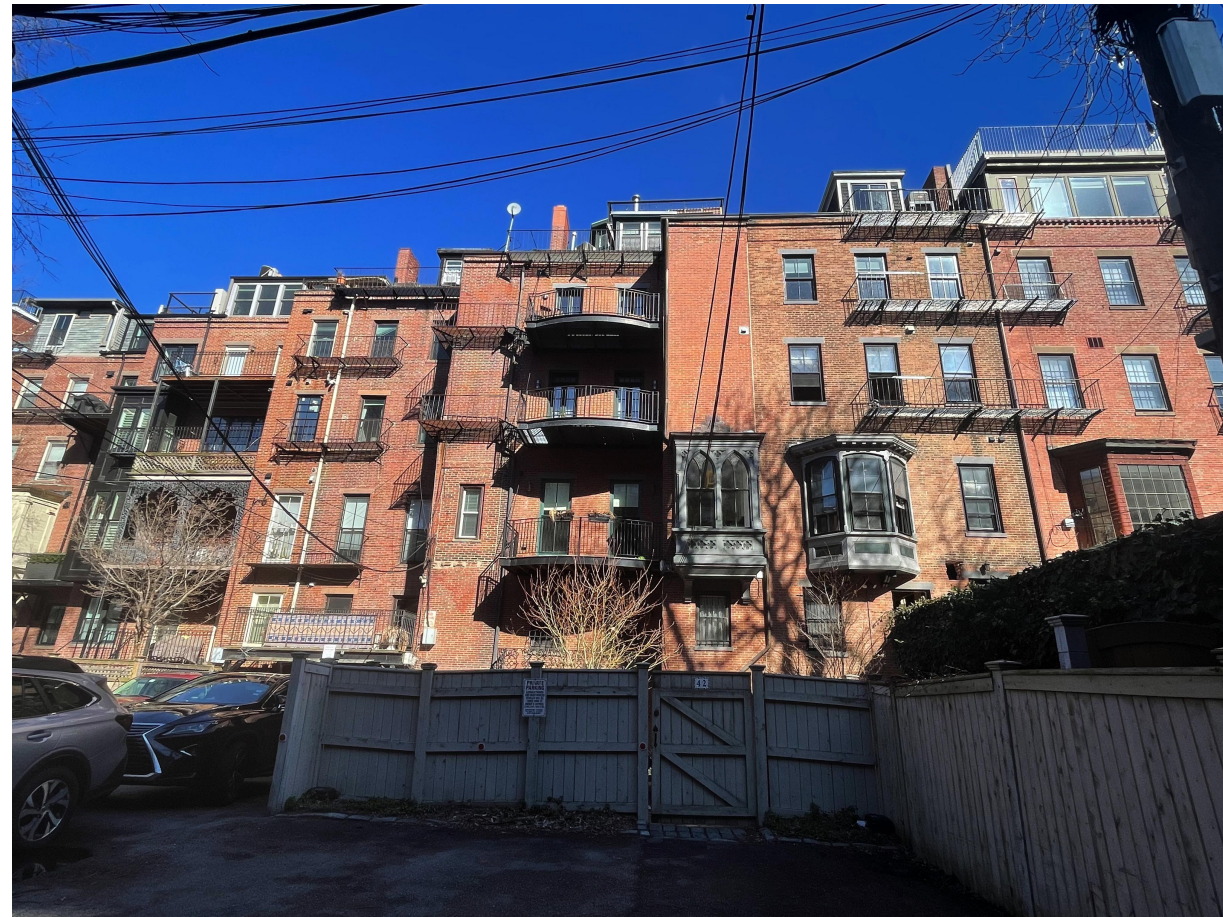
DORMER & ROOF DECK CONTEXT ALONG PUBLIC ALLEY 701 (UNITS 38-50)
