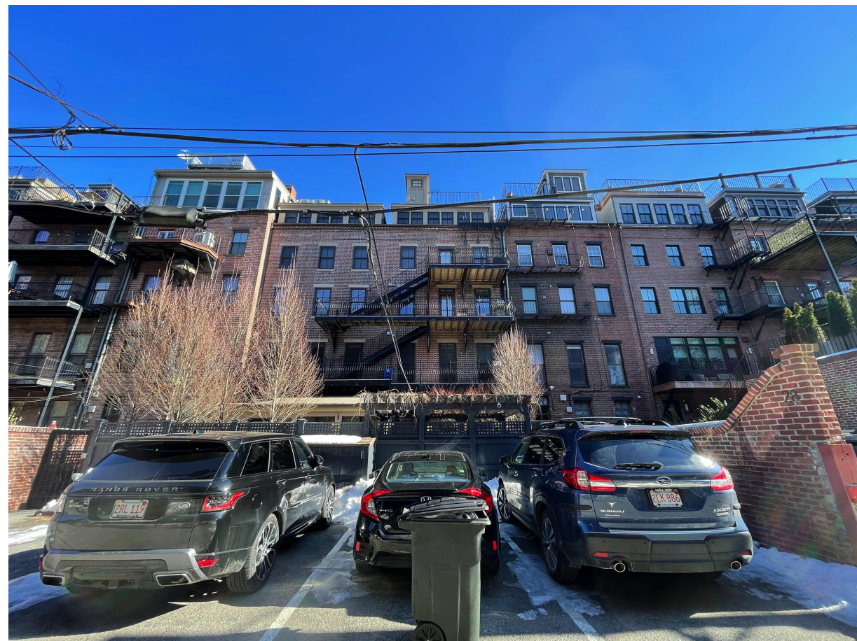
DORMER & ROOF DECK CONTEXT ALONG PUBLIC ALLEY 701 (UNITS 20-36)
