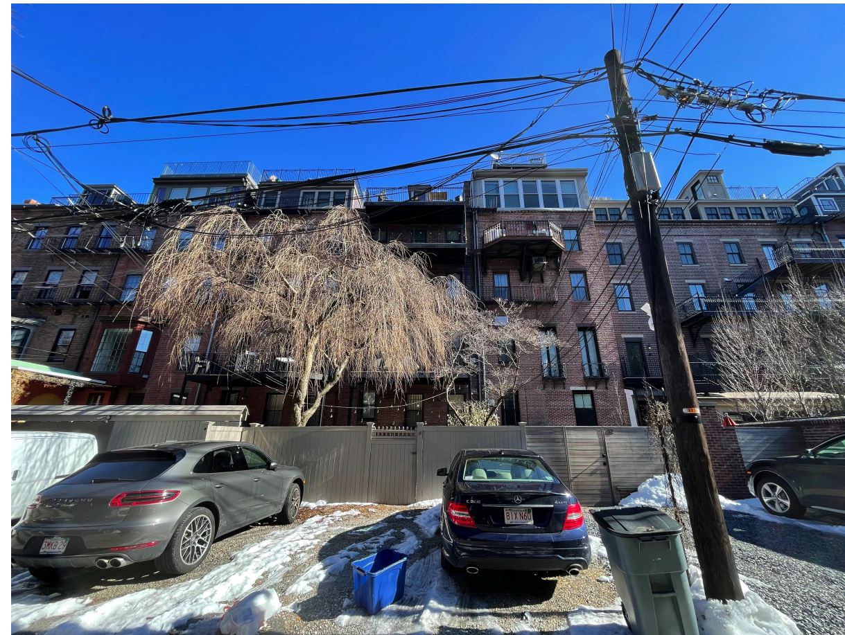
DORMER & ROOF DECK CONTEXT ALONG PUBLIC ALLEY 701 (UNITS 26-40)
