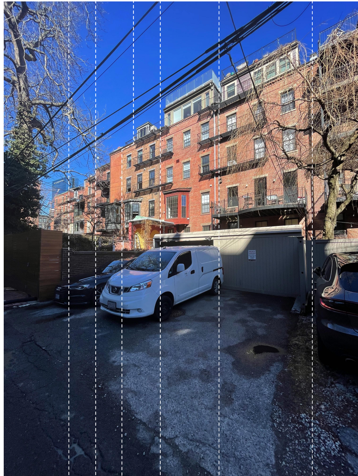
VIEW LOOKING NORTH ALONG PUBLIC ALLEY 701 (REAR ELEVATION)
