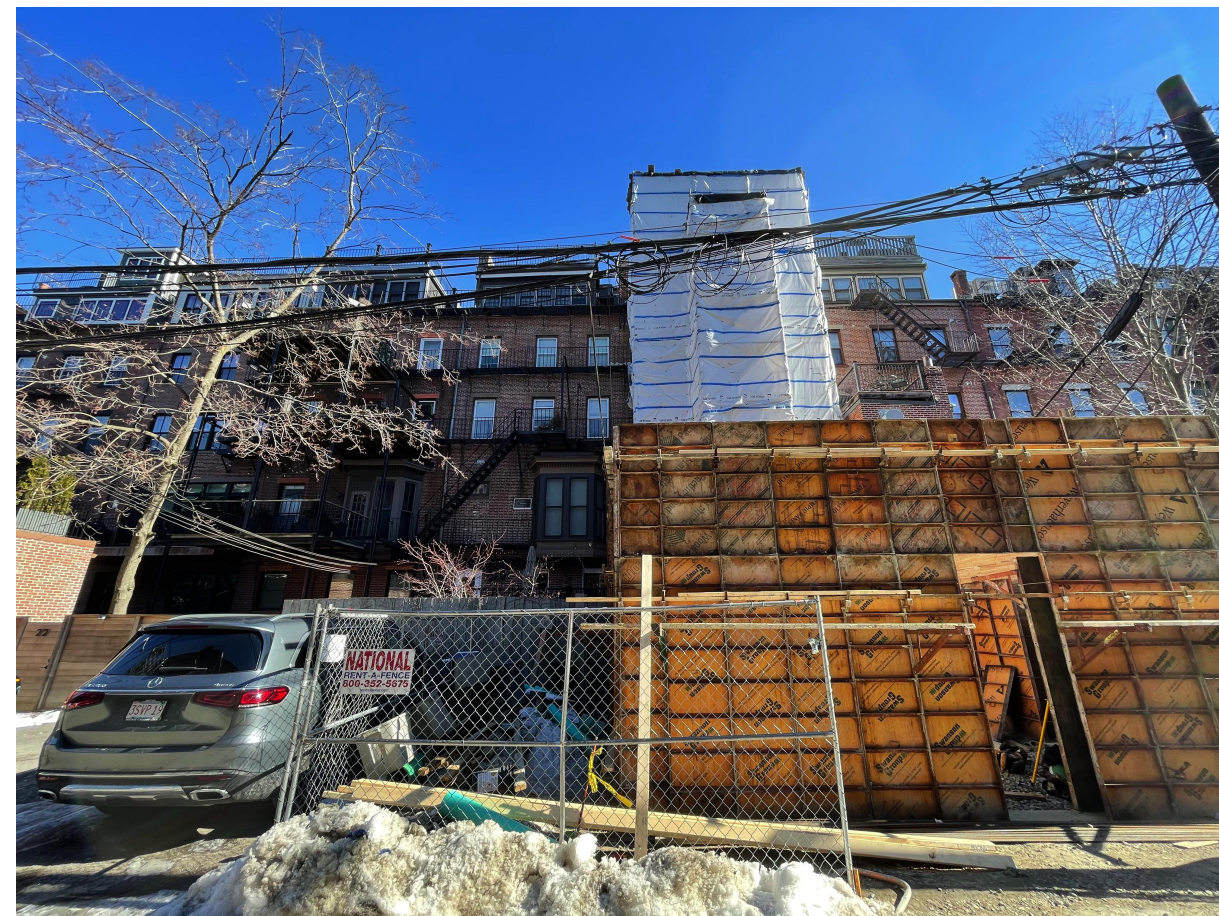
DORMER & ROOF DECK CONTEXT ALONG PUBLIC ALLEY 701 (UNITS 12-26)
