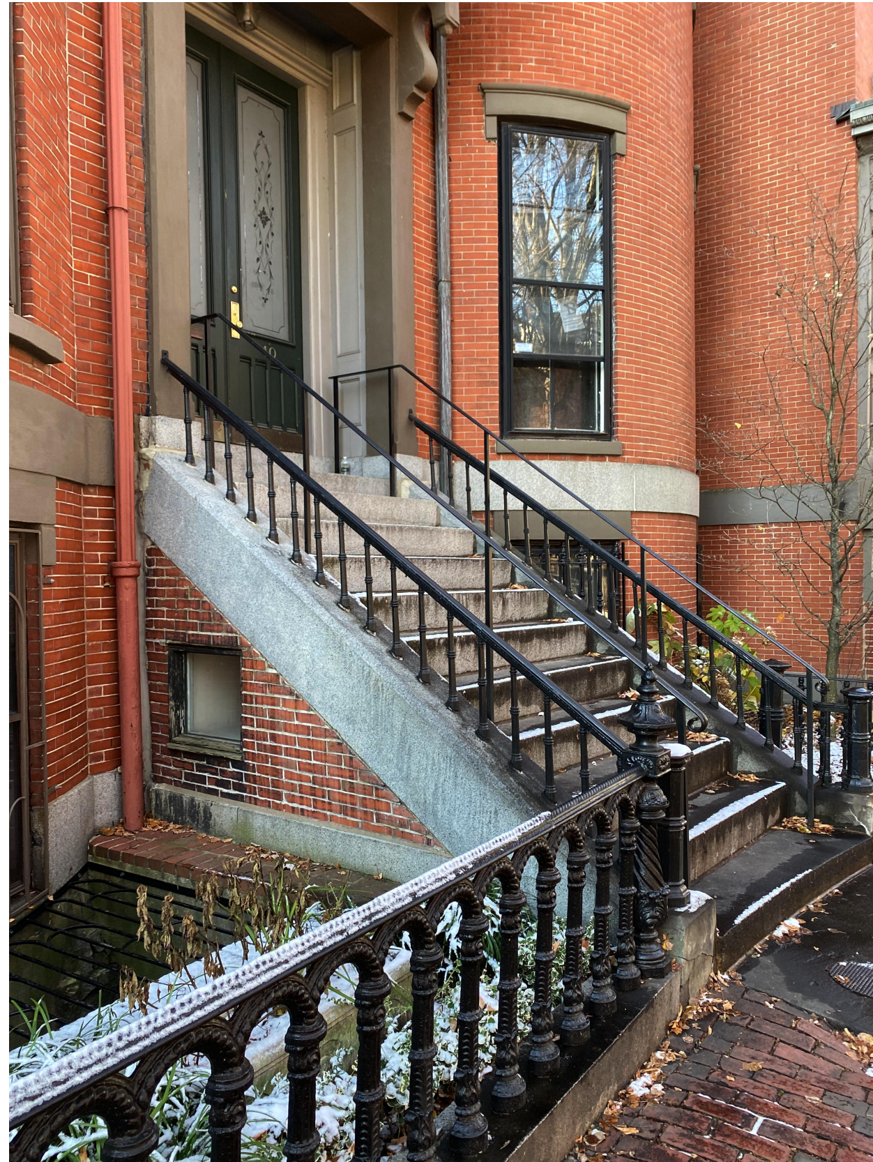
DETAIL VIEW: EXISTING STONE STOOP
