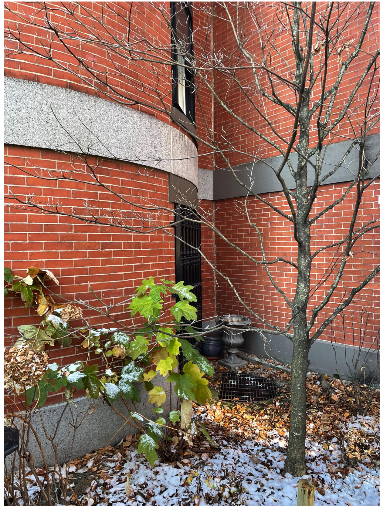
DETAIL VIEW: FRONT GARDEN WITH EXISTING WELL & GRATE
