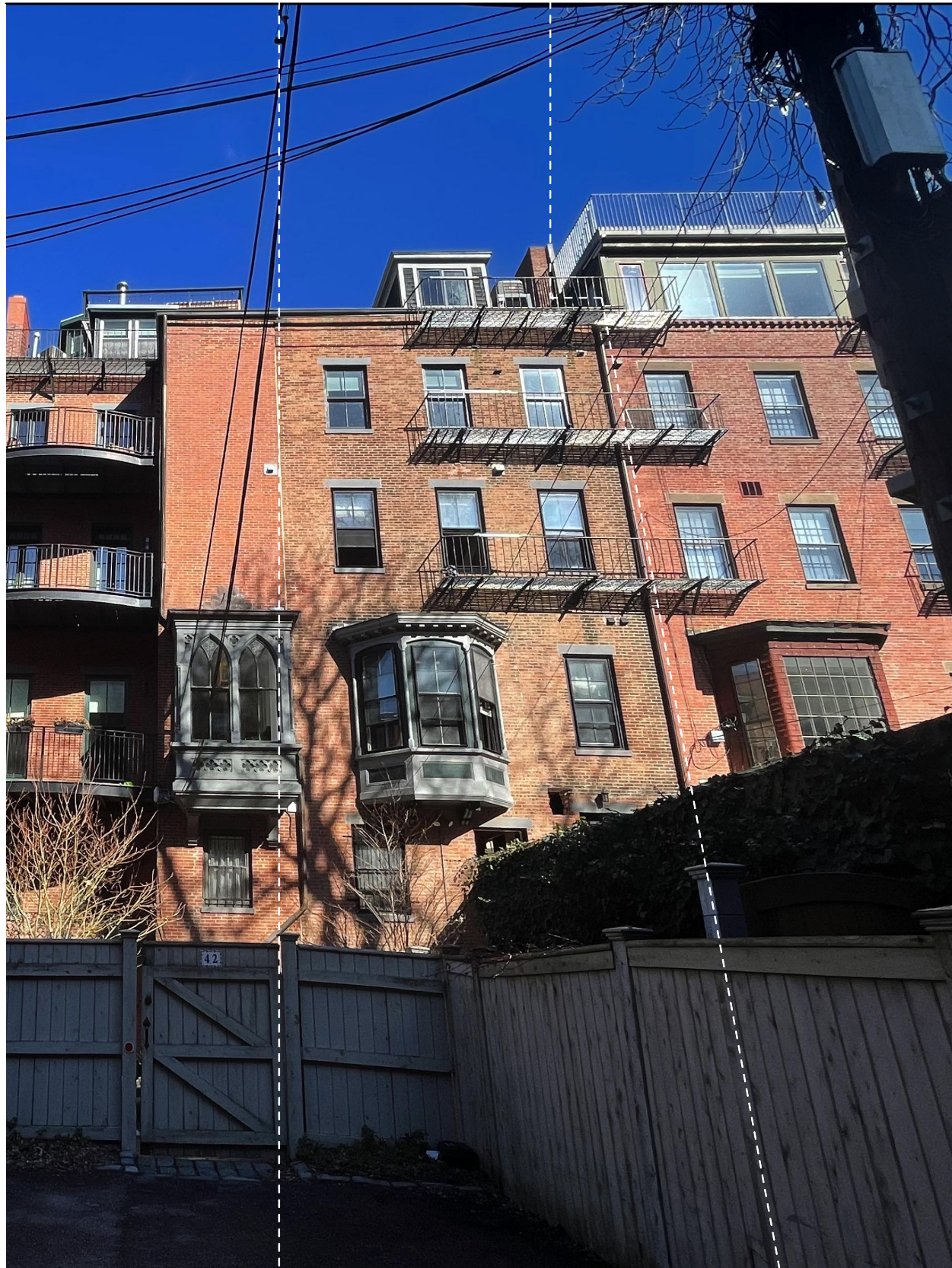
VIEW LOOKING EAST FROM PUBLIC ALLEY 701 (REAR ELEVATION)
