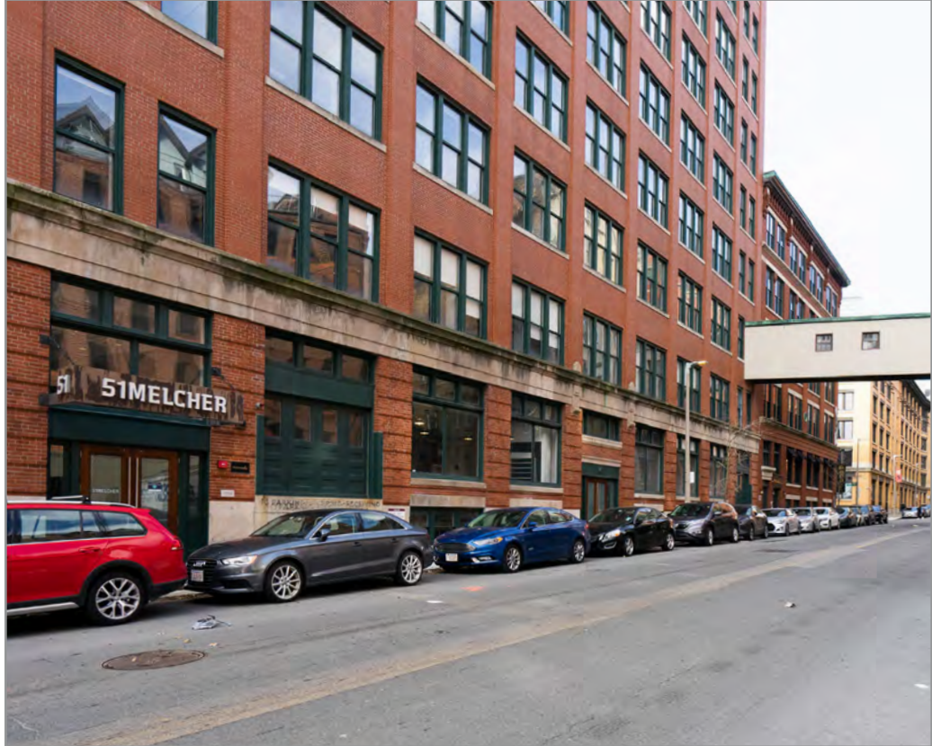
FRONT VIEW ON MELCHER ST
