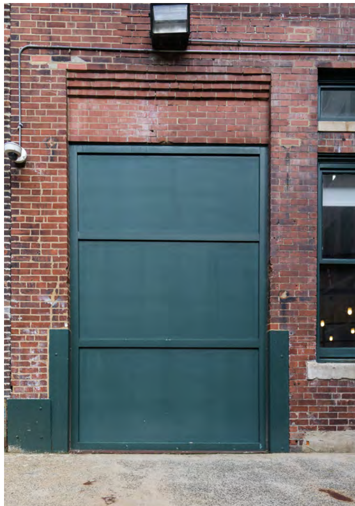
EXISTING INFILL TO BE REPLACED WITH DOOR
