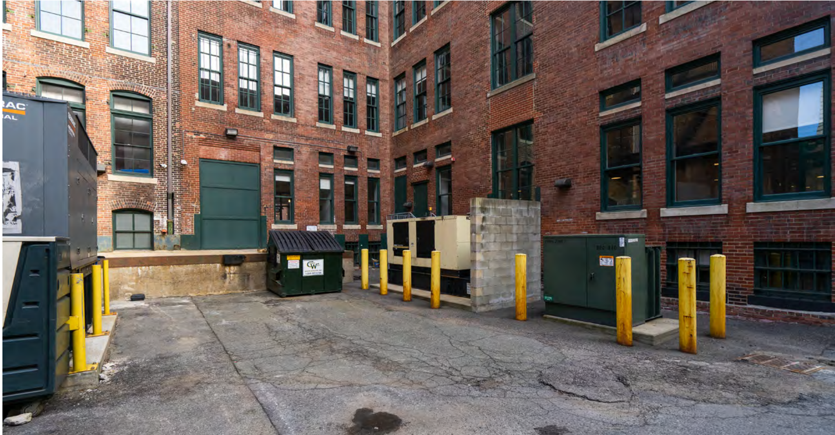
EXISTING VIEW OF 51 MELCHER FROM NECCO COURT
