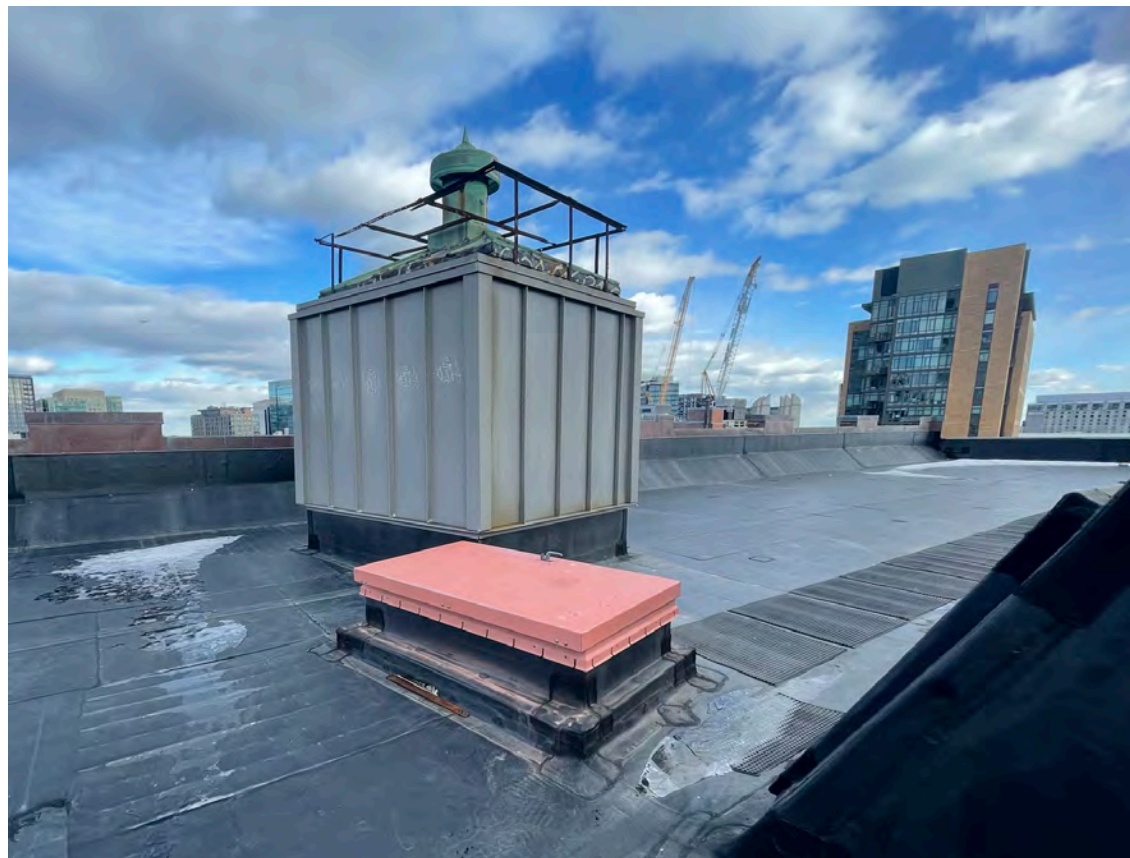
EXISTING ABONDONED LIFT HEADHOUSE AND ROOF HATCH
