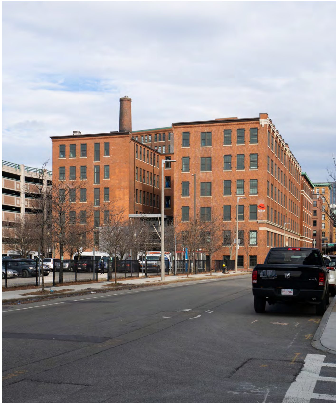
EXISTING VIEW 500' DOWN A STREET AT WORMWOOD
