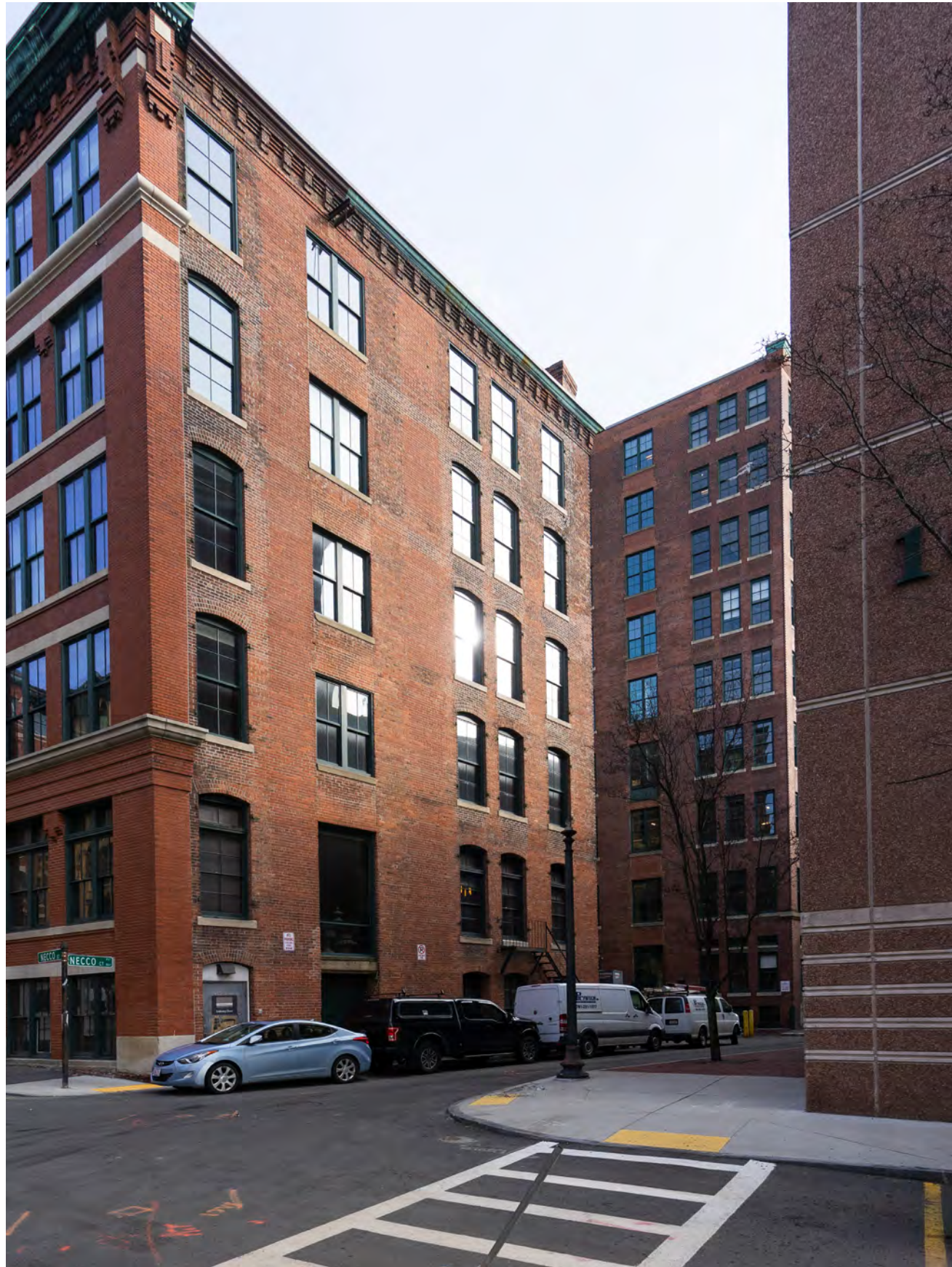
EXISTING VIEW FROM NECCO STREET
