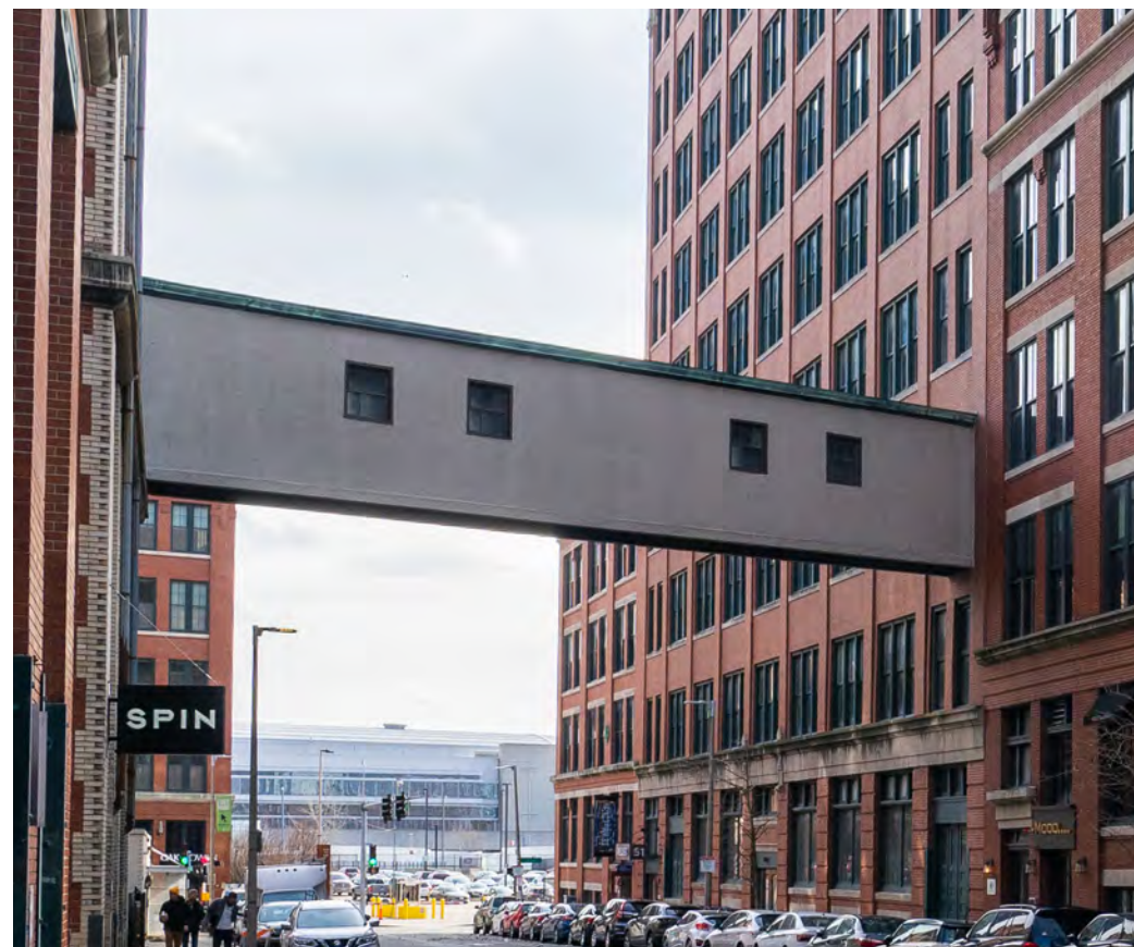
SKYBRIDGE - LOOKING TOWARDS A ST
