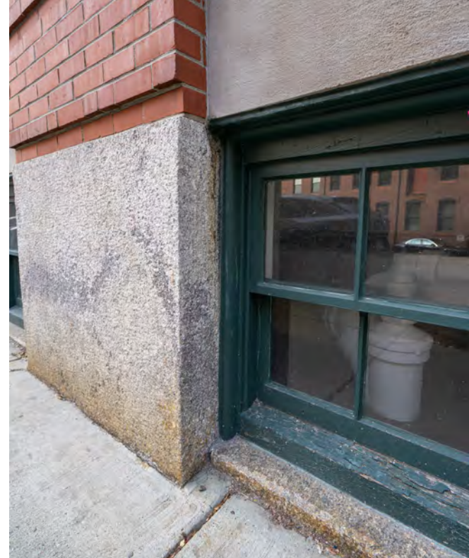
EXISTING BASEMENT WINDOWS
