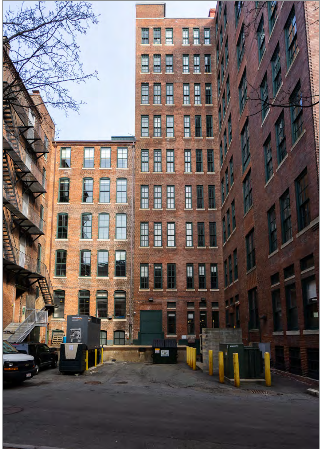
REVITALIZED LOADING DOCK
