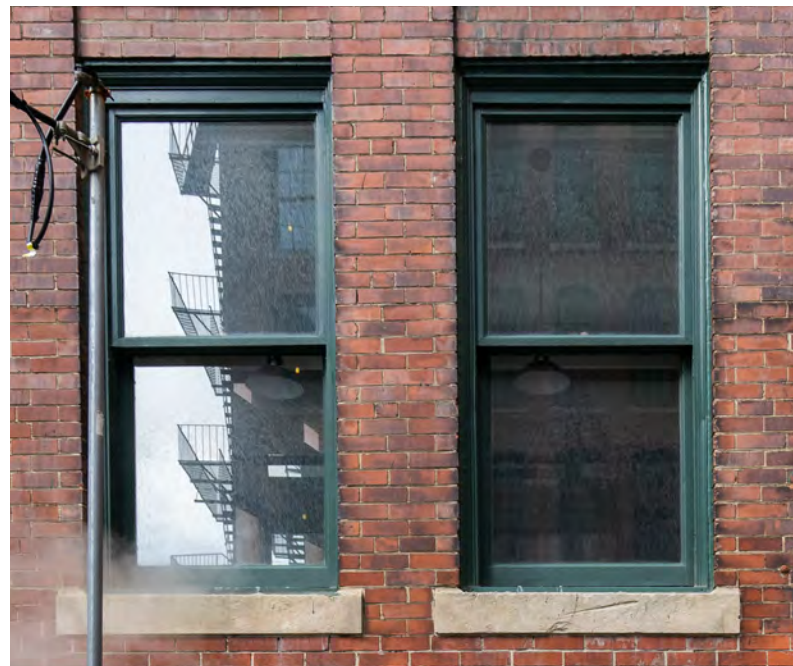
EXISTING WINDOW TO BE INFILLED
