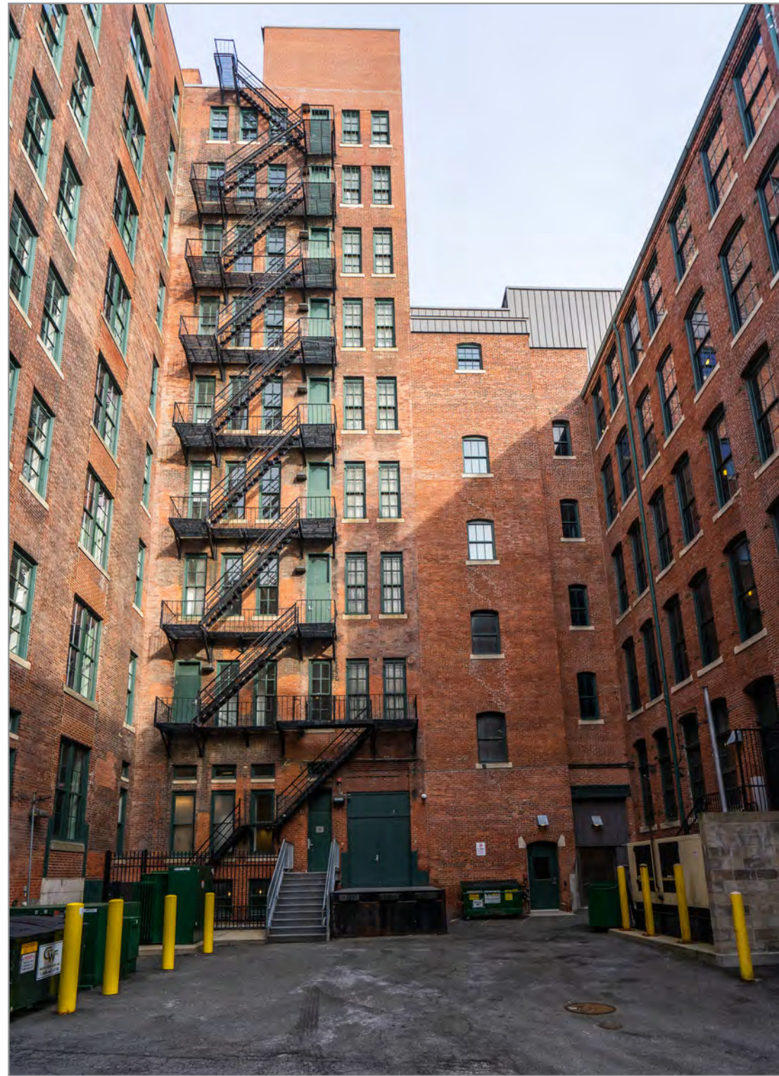
EXISTING LOADING DOCK
