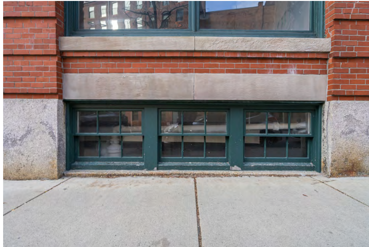
EXISTING BASEMENT WINDOWS
