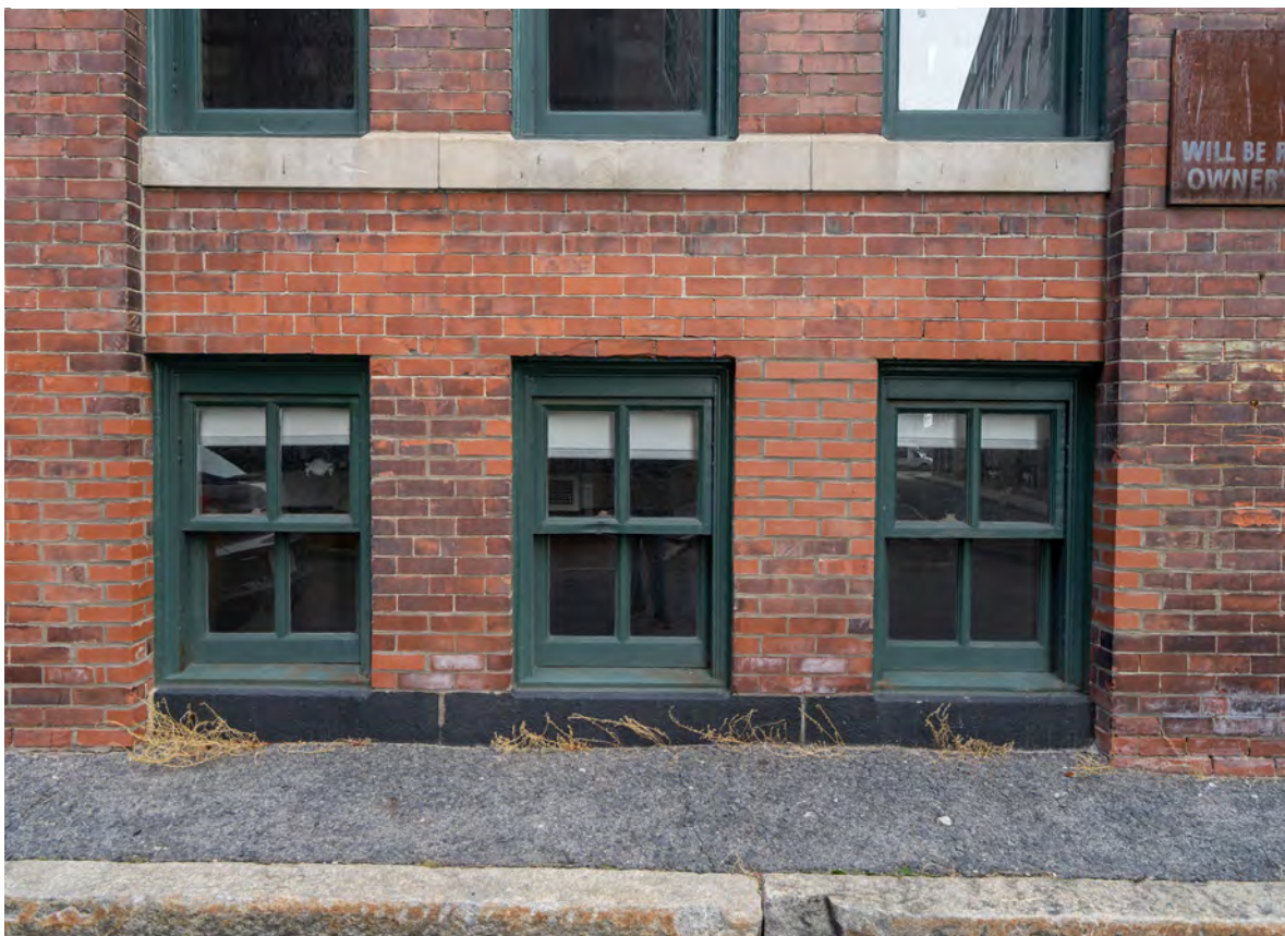
EXISTING BASEMENT WINDOWS
