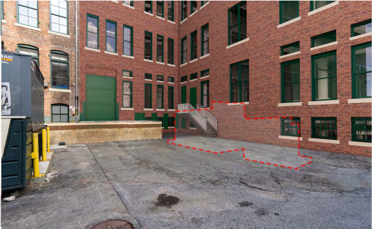
EXISTING VIEW WITH HIDDEN GENERATOR
