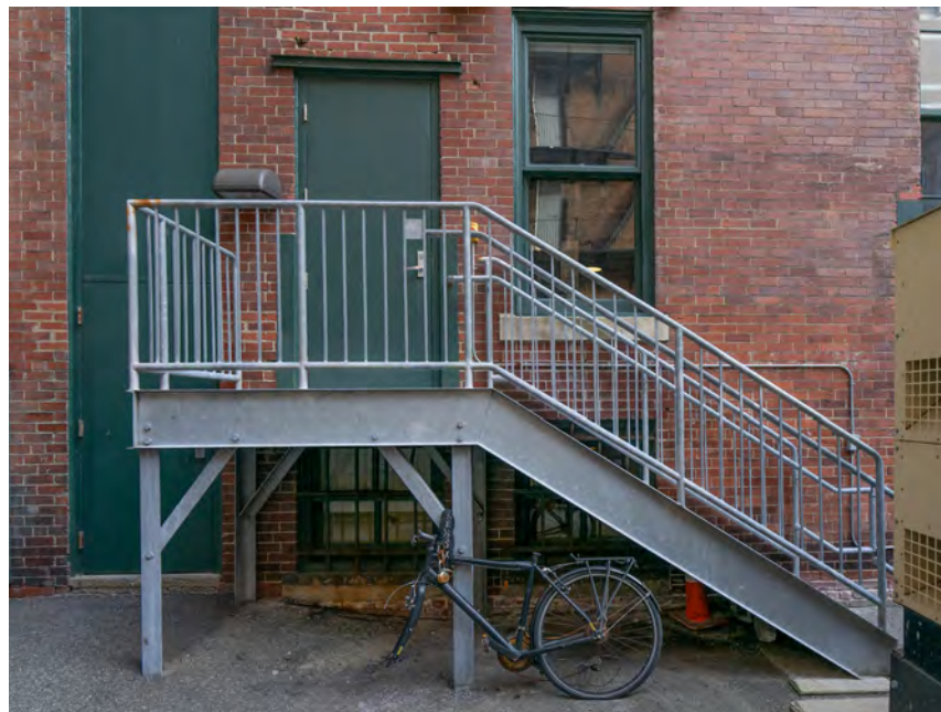
EXISTING STAIR TO BE REMOVED
