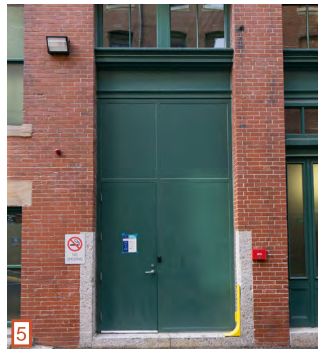
5 NECCO STREET - DOOR AND LOUVER
