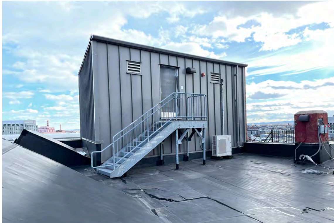
EXISTING ELEVATOR OVERRUN
