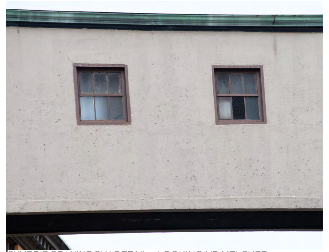
SKYBRIDGE WINDOW DETAIL - LOOKING UP MELCHER
