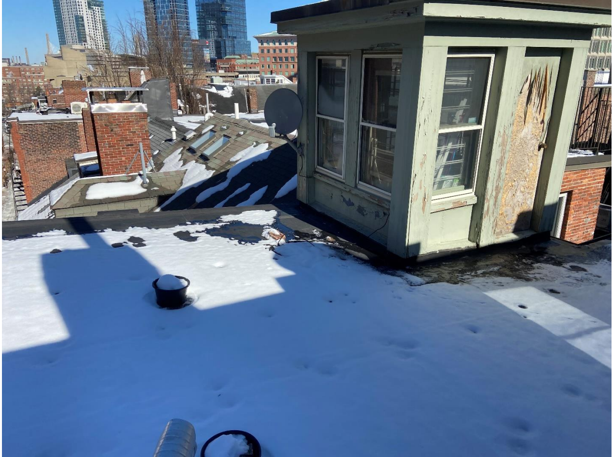
Roof and headhouse – facing North
