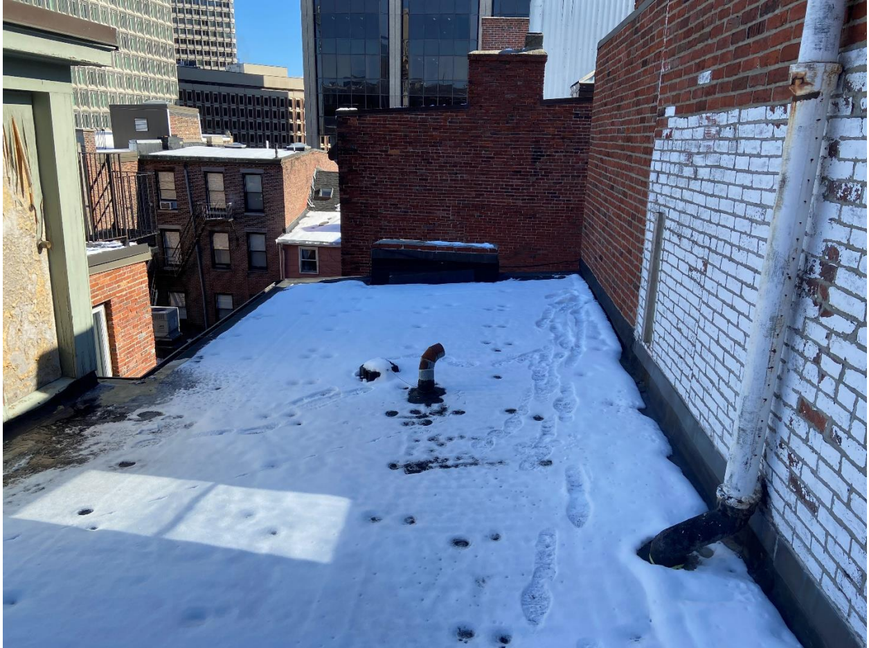
Roof and headhouse – facing East
