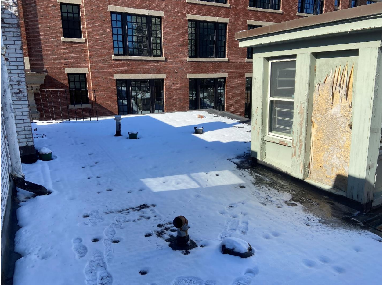
Roof and headhouse – facing West
