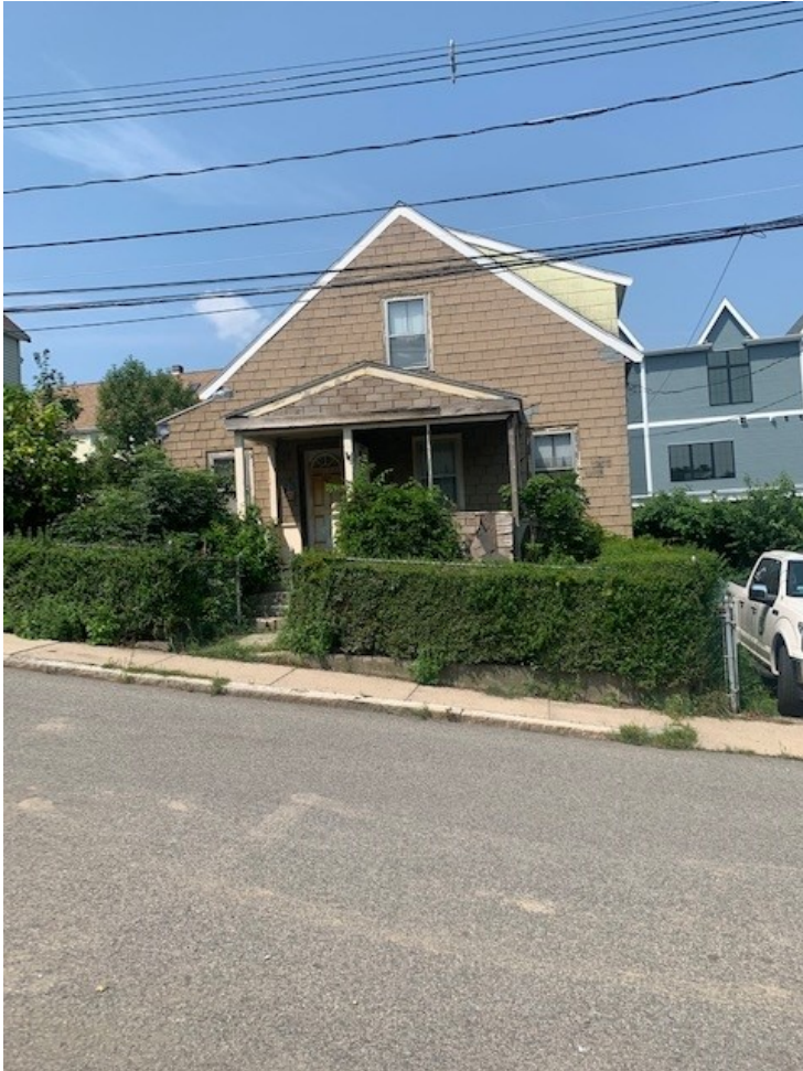
1) Front of 26 Tilesboro St
