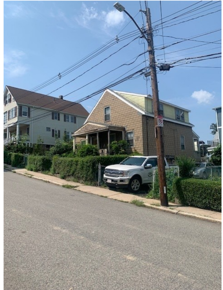
2) Front & Right Side of 26 Tilesboro St
