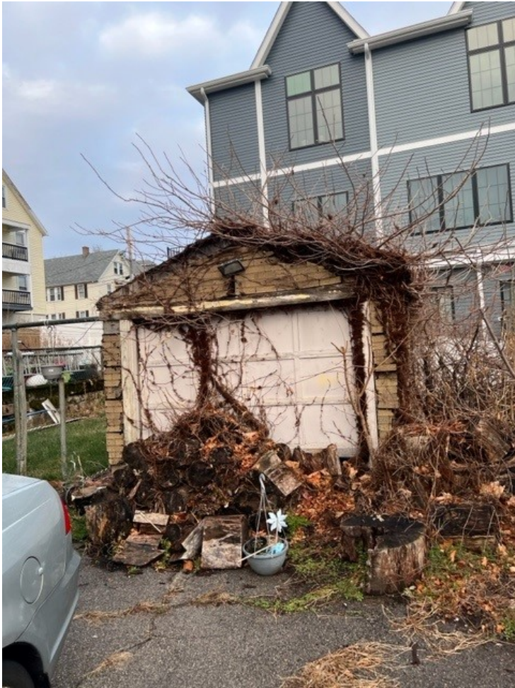
7) Front of Shed at 26 Tilesboro
