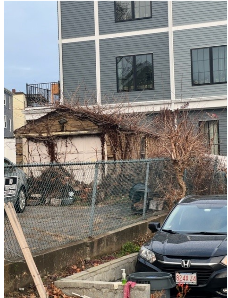
8) Front and Right Side of Shed at 26 Tilesboro
