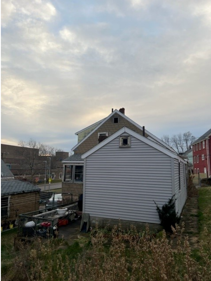
5) Rear of 26 Tilesboro St
