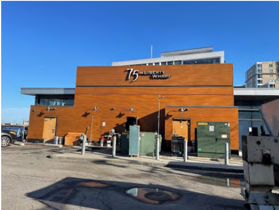
Looking East at proposed location of 20' container pads
