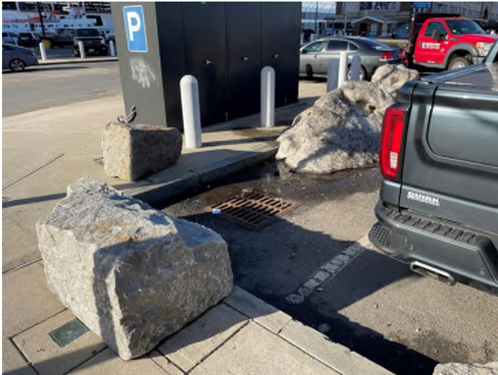
Catch Basin at west end of parking lot near proposed location of 40' container pads
