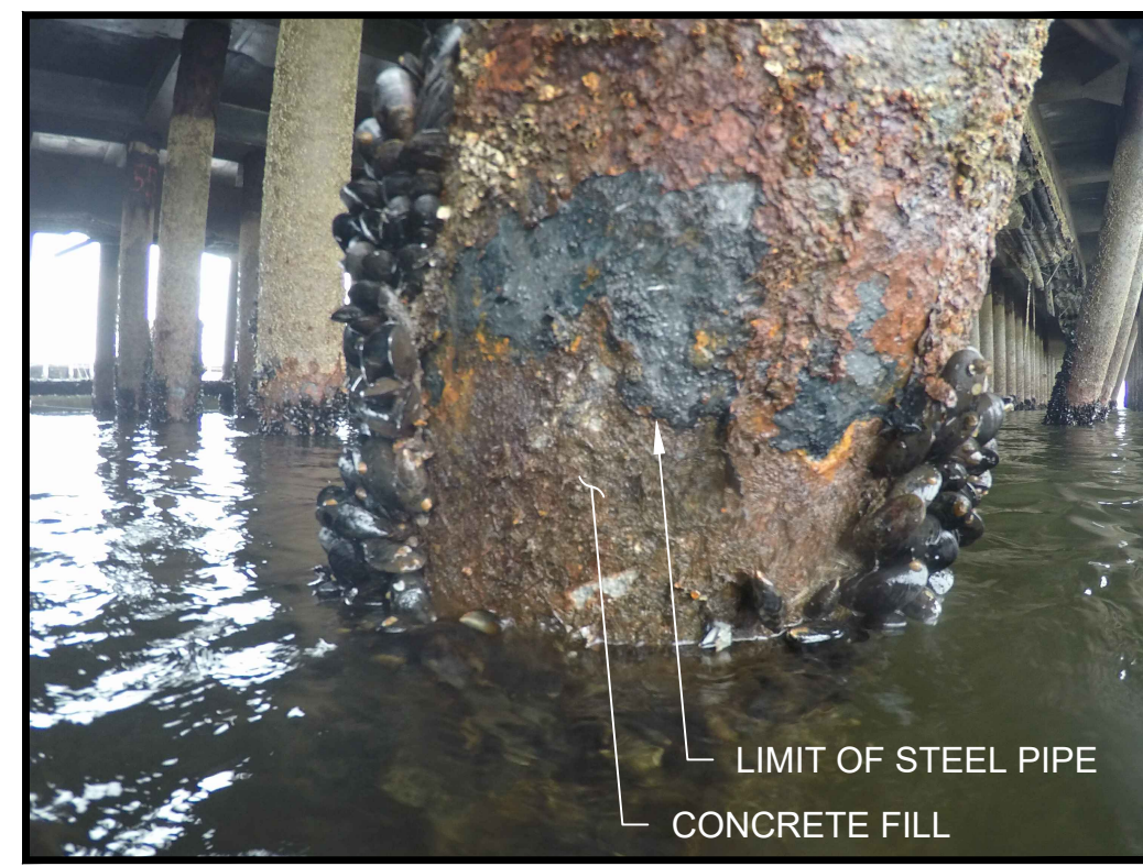
PHOTO 17 - TYPICAL PILE CONDITIONS NEAR MLW
