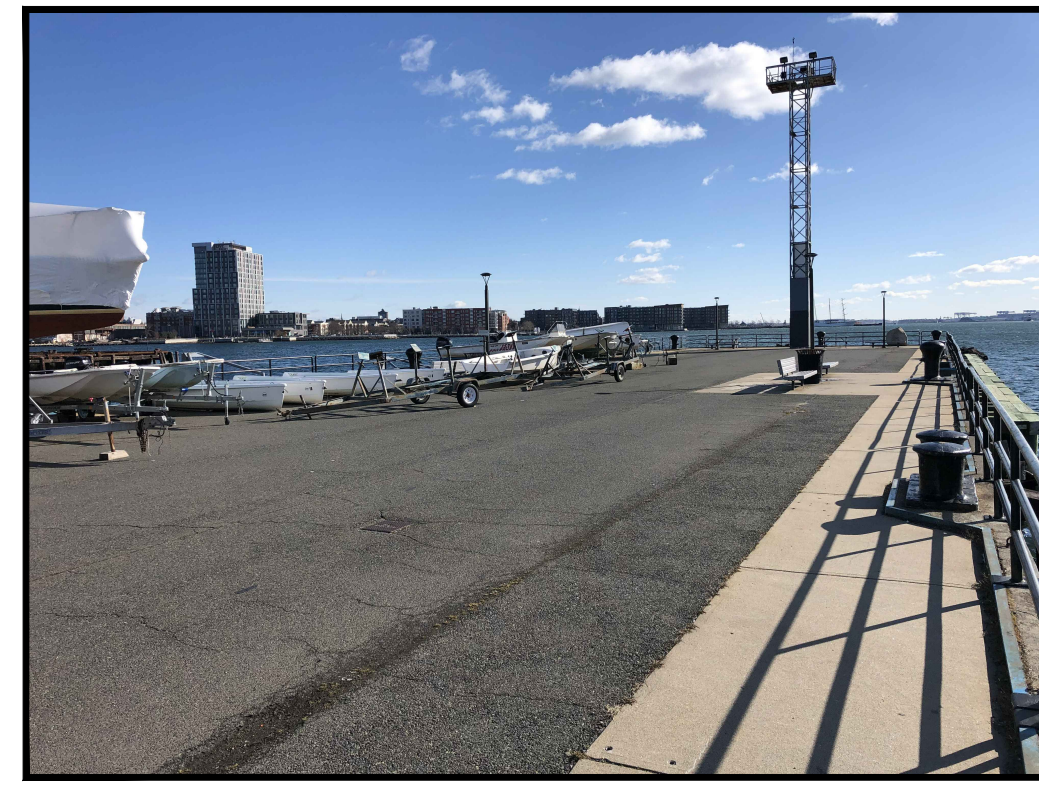
PHOTO 8 - SOUTH END OF PIER - TOPSIDE
