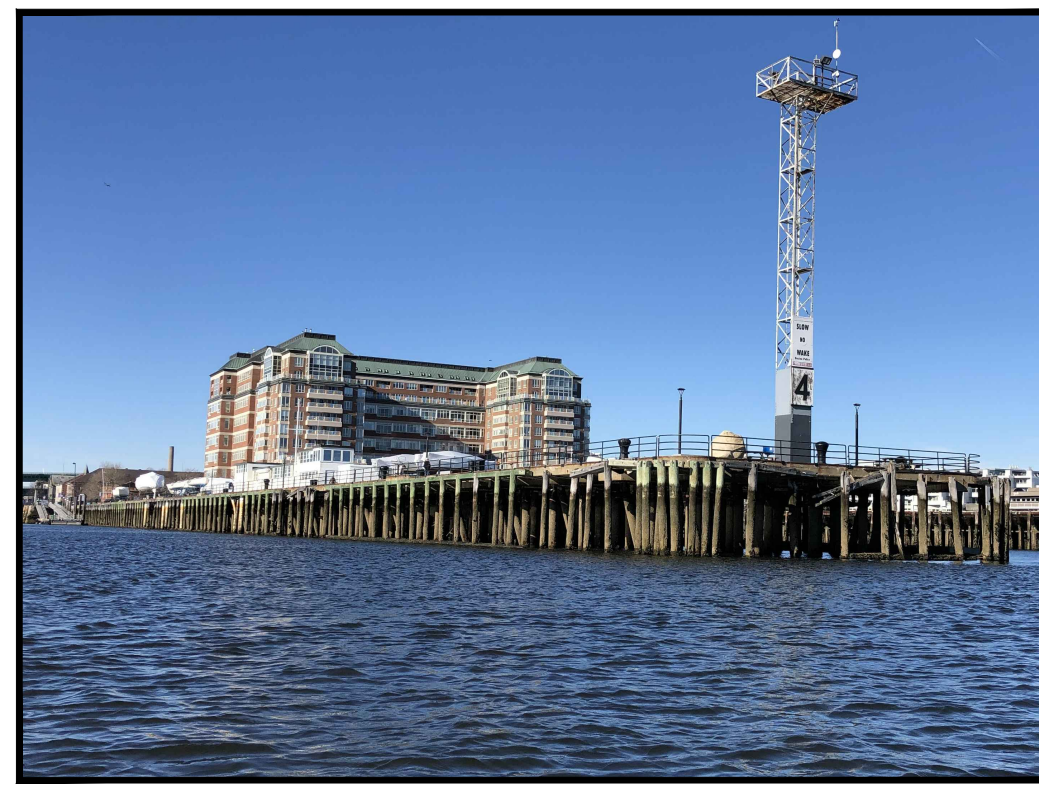
PHOTO 1 - PIER 4 OVERALL LOOKING NORTH
