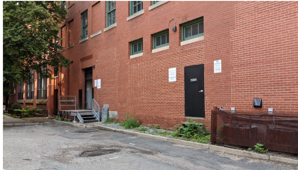
Existing Loading dock conditions
