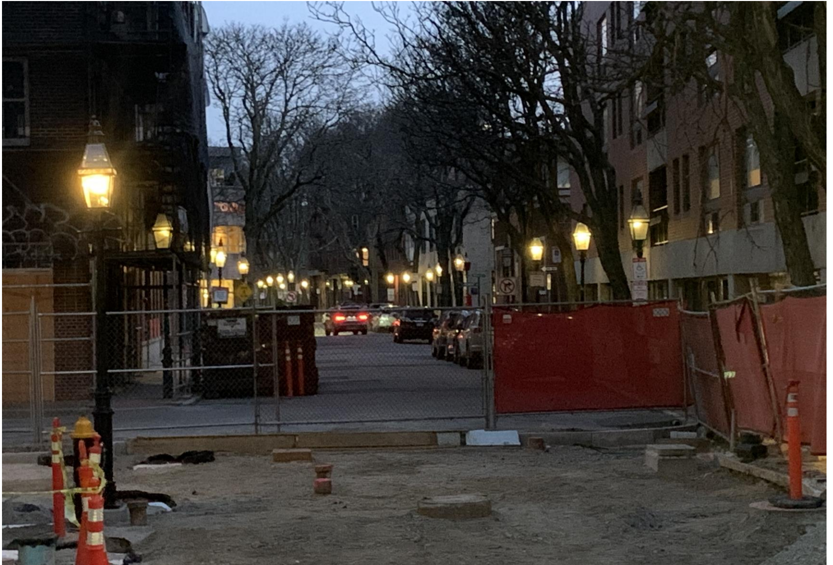
Color temperature: 3,000K Comparison to existing gas lamp fixtures
