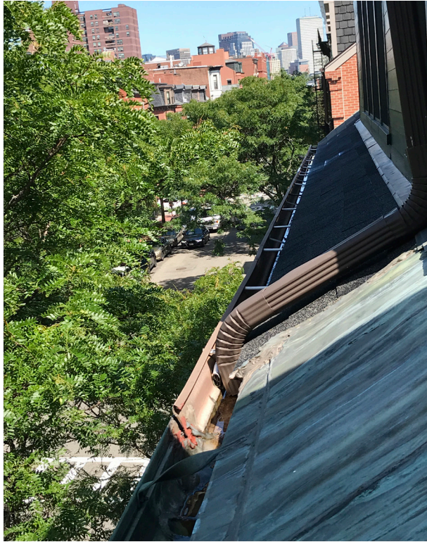
TRANSITION BETWEEN SLATE (456 SHAWMUT) AND ASPHALT SHINGLES
