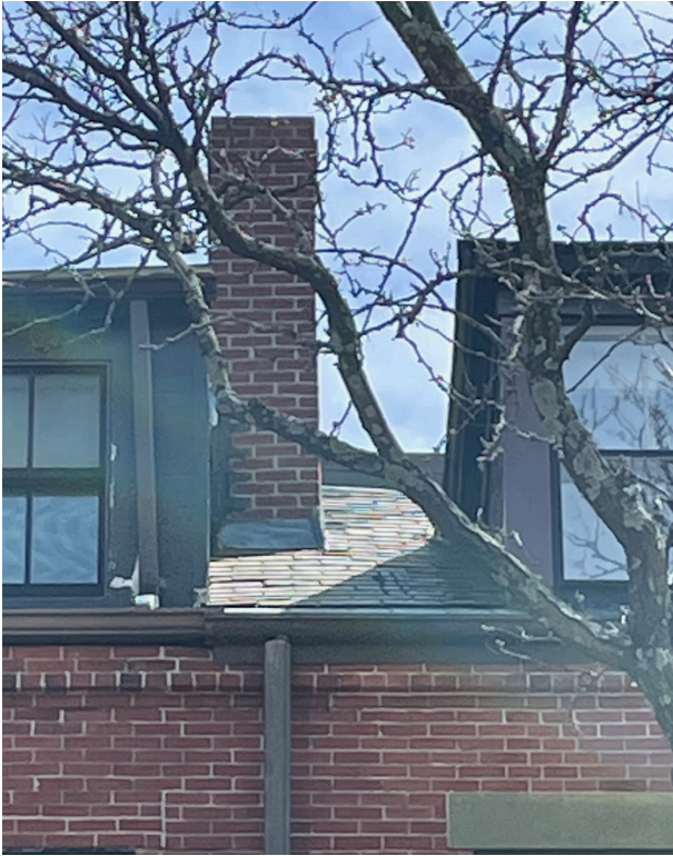
ROOF LINE BETWEEN 24 RUTLAND STREET (LEFT) AND 456 SHAWMUT
