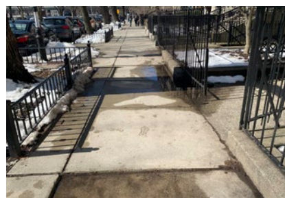
Replace/Regrade Existing Concrete Sidewalk
