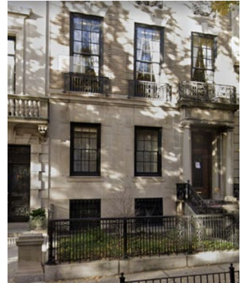
New Cast Iron Fence to match balcony railings (precedent below)
