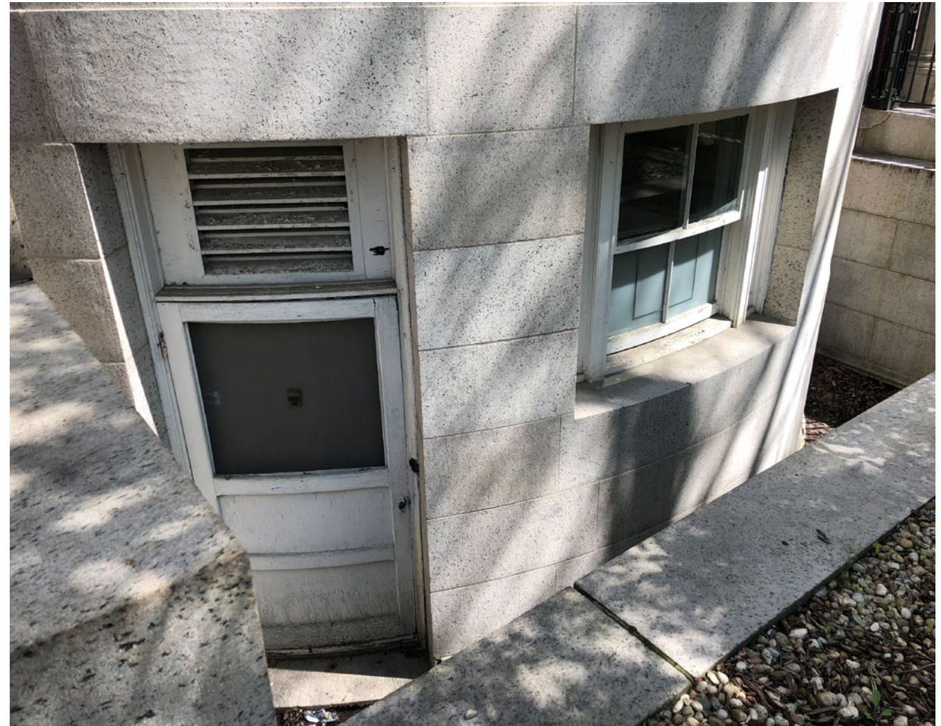
Basement wood door and windows, to be retained and refurbished.
