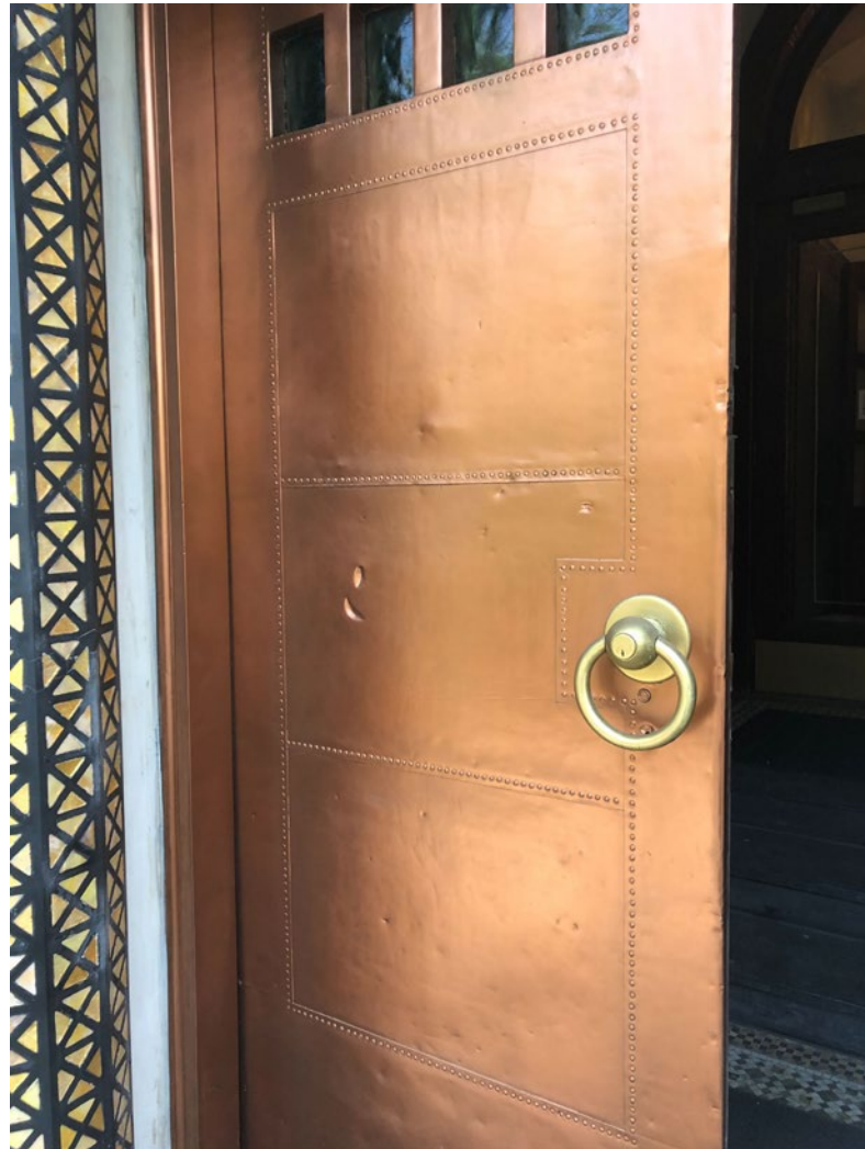
Copper clad entry door, dents cannot be repaired, copper is not punctured
