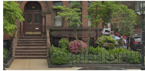
12-18" Ornamental Metal Fence on Existing Granite Wall
