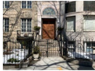
Remove Existing Gate at Main Entrance
