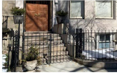
Keep Existing Handrails at Main Entrance
