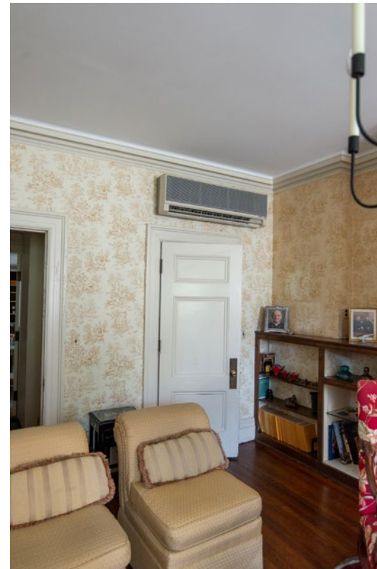
North wall, door trim detail
