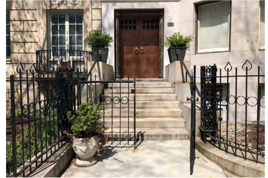
Existing Fence and Gate
