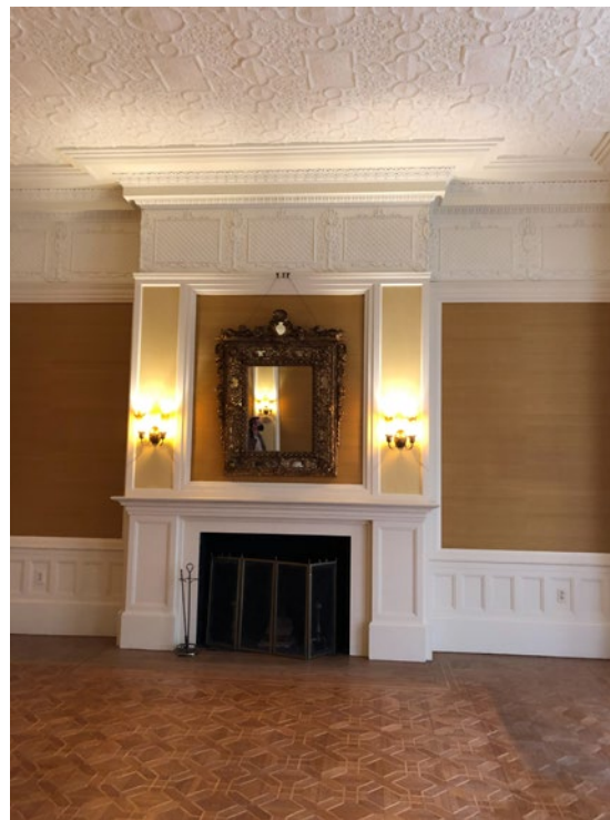
East wall - fireplace
