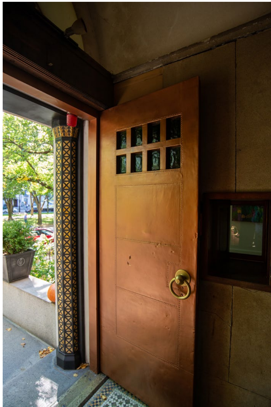
Copper clad entry doors
