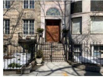
Remove Existing Gate at Main Entrance
