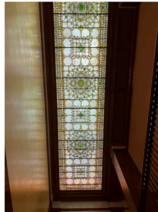
Stained glass lay light over stair
