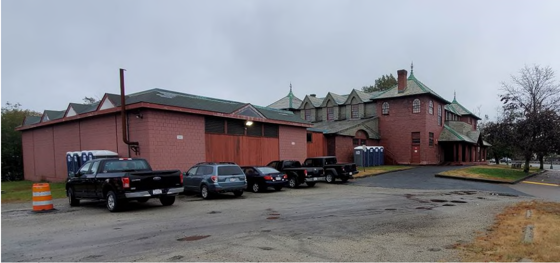
Image 1 - Existing Building next to Boathouse
