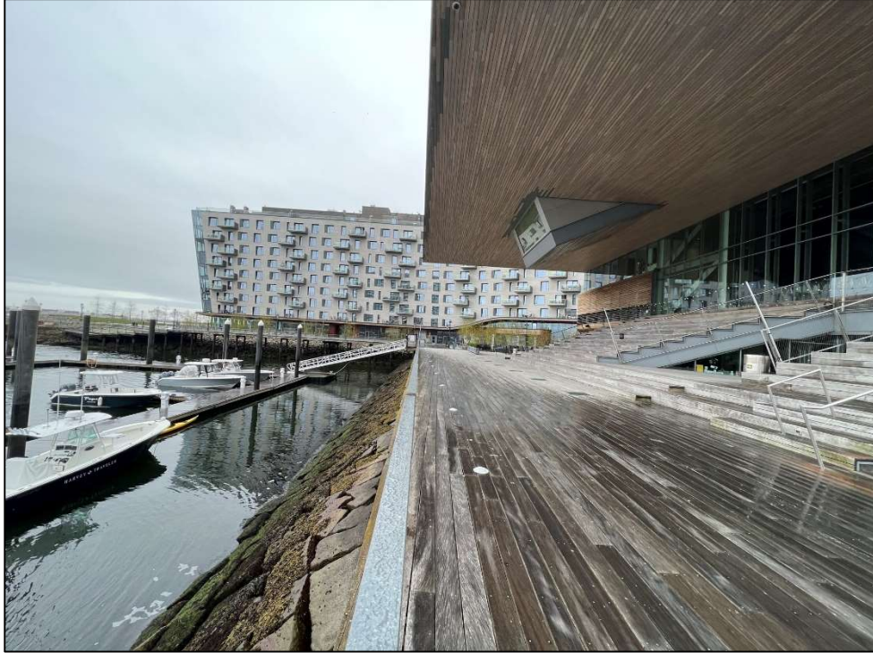
Photo 4 – Coastal Bank at ICA Building 2
