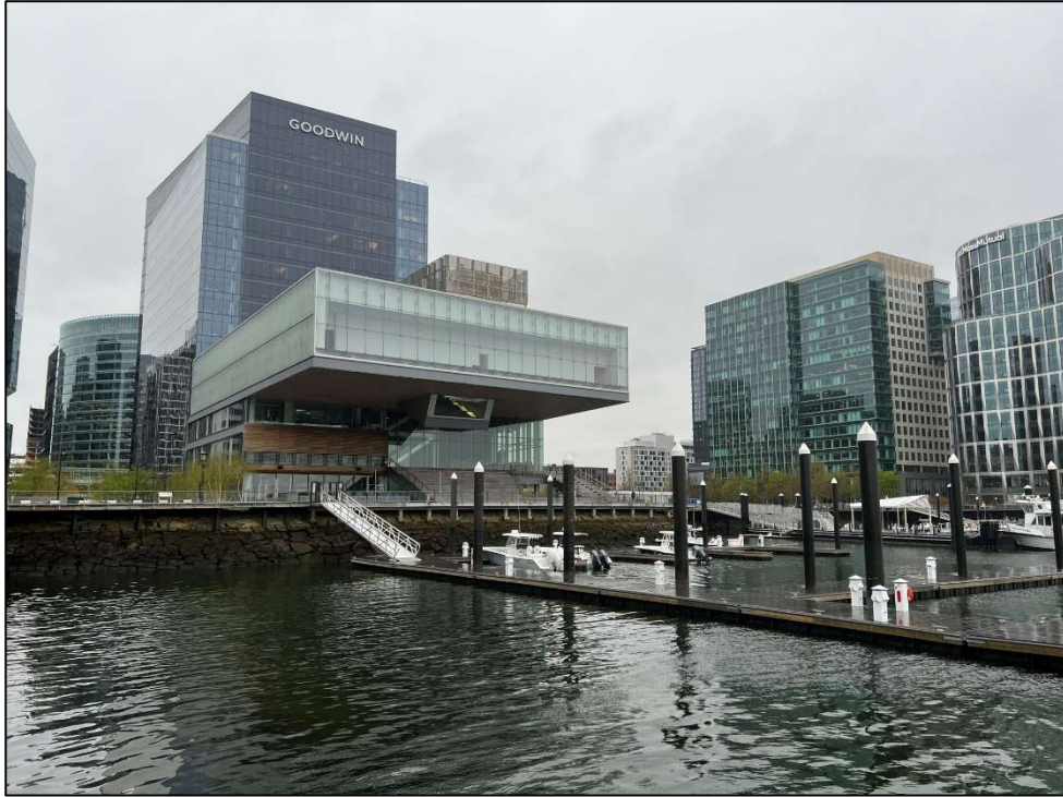
Photo 2 – ICA Building Elevation
