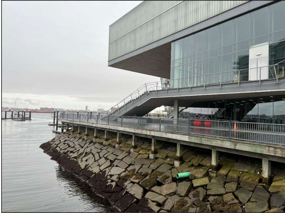
Photo 6 – Typical Deck Footings at ICA Building
