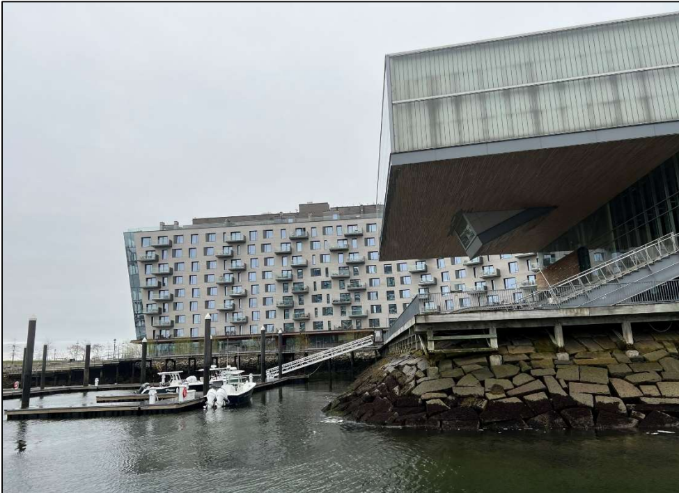
Photo 5 – Coastal Bank at ICA Building 3
