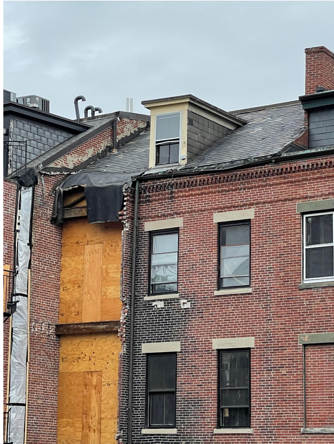
REAR DORMER AT 10 UNION PARK (ORIGINAL DORMER)
