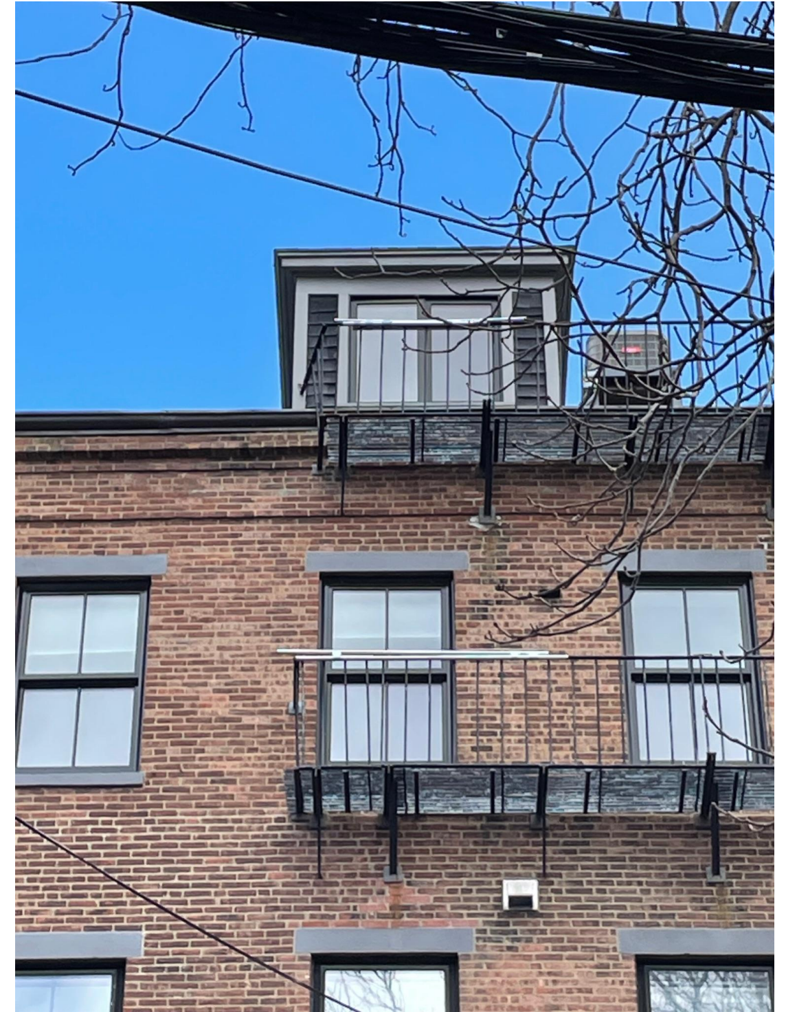
REAR DORMER AT 40 UNION PARK
