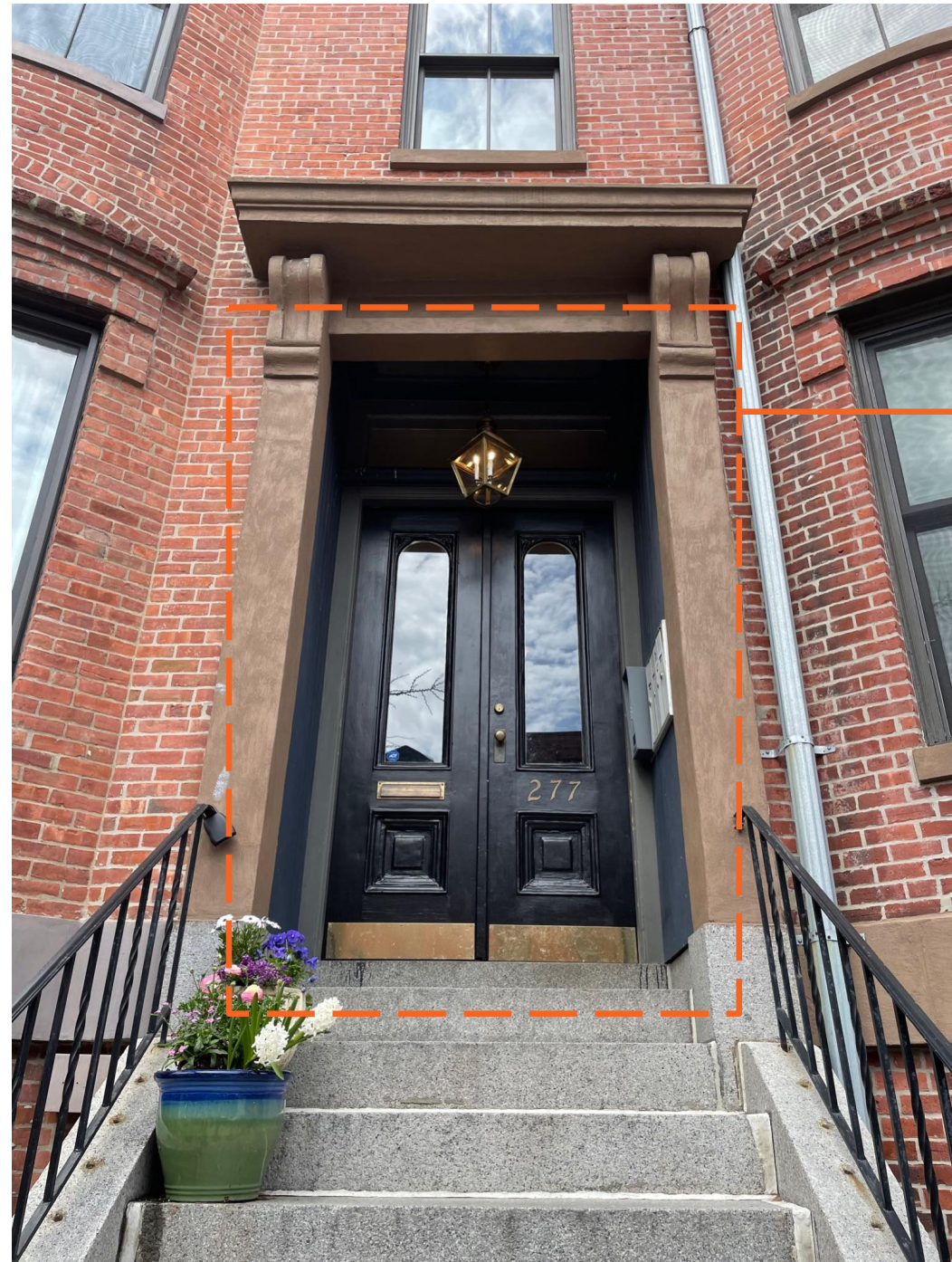
ENTRY DOOR AT 277 SHAWMUT AVENUE
