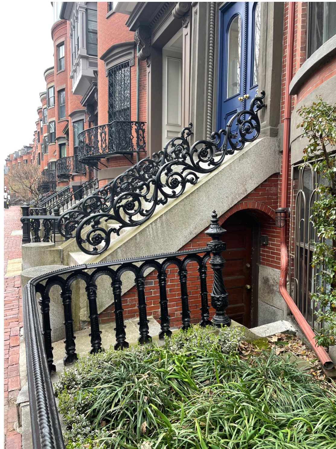
STOOP DOOR AT 38 UNION PARK (NEIGHBORING)
