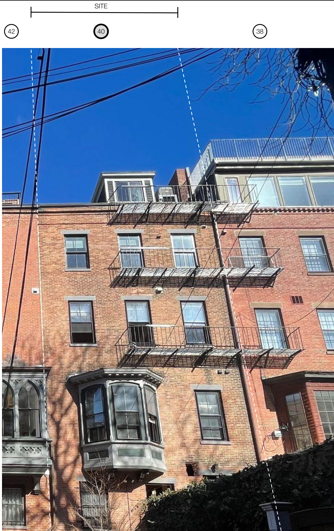
VIEW LOOKING EAST FROM PUBLIC ALLEY 701 (REAR ELEVATION)
