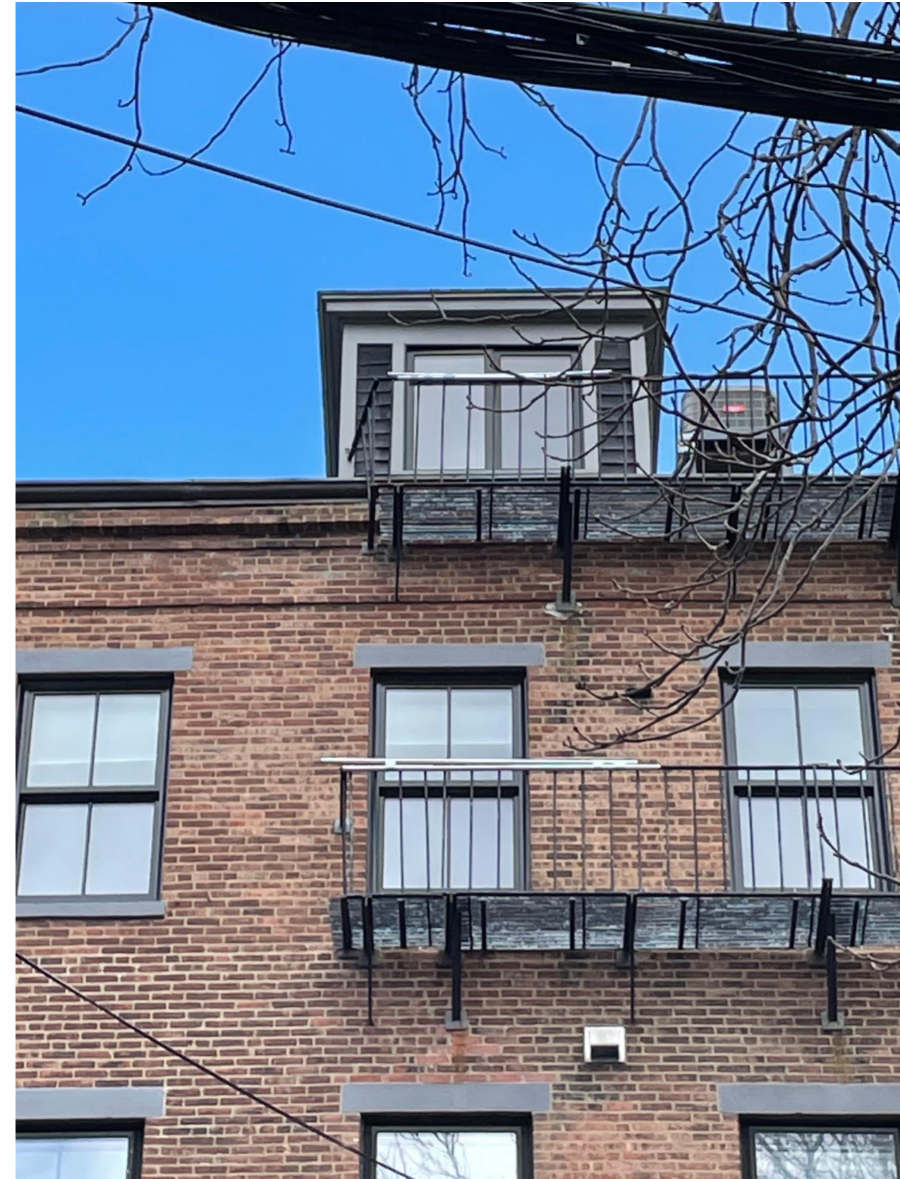
DETAIL VIEW - CORNICE LINE & REAR DORMER (REAR ELEVATION)
