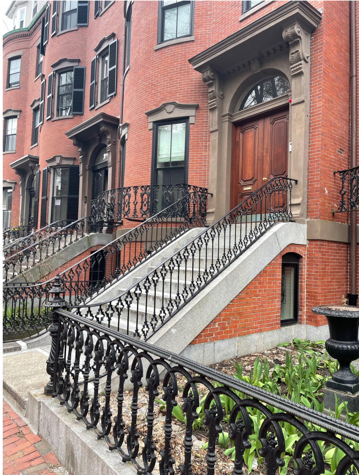
STOOP WINDOWS IN BRICK AT 4 & 6 UNION PARK
