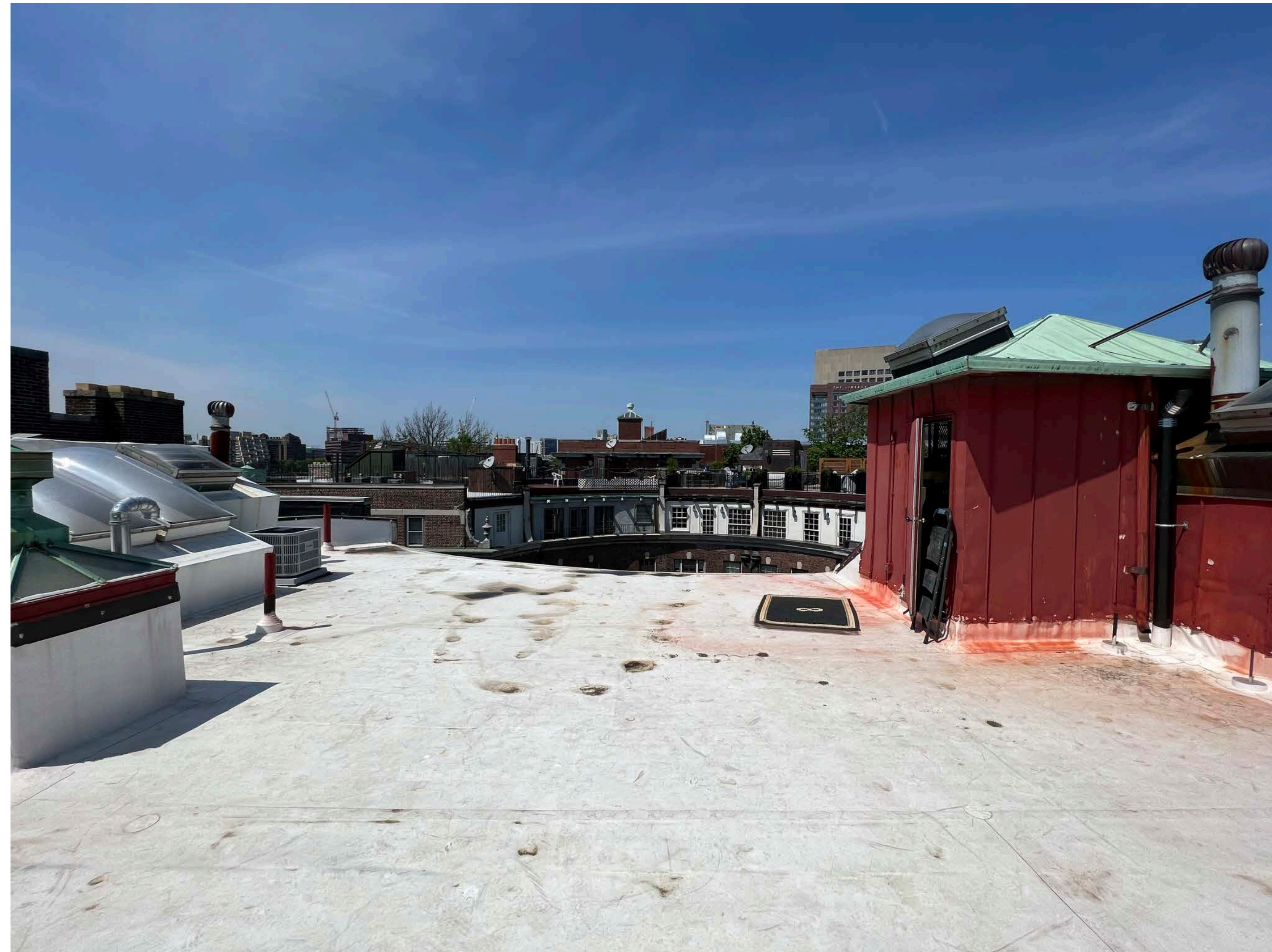
EXISTING ROOF DECK AT 8 WEST HILL PLACE
