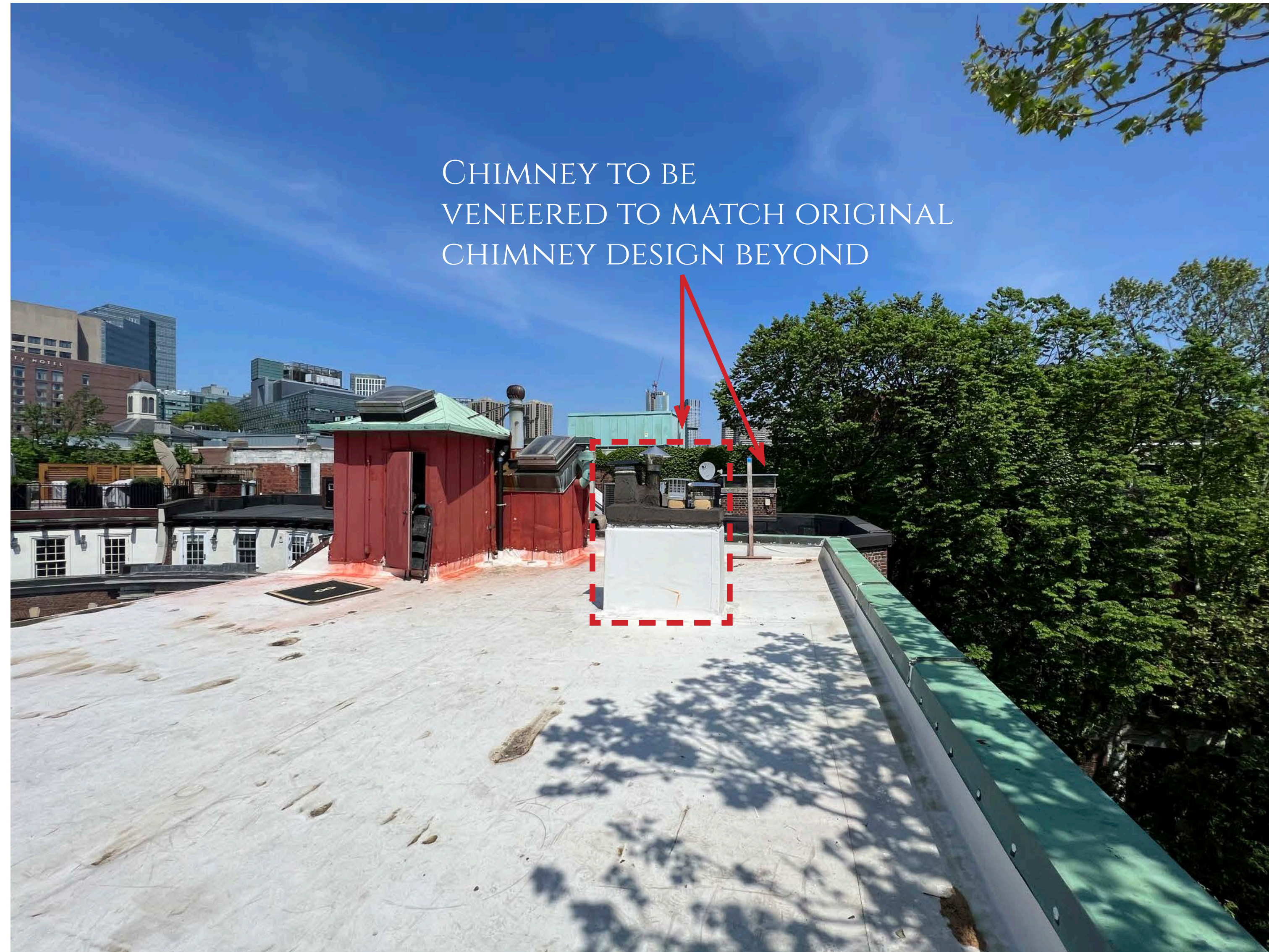
EXISTING ROOF DECK AT 8 WEST HILL PLACE
