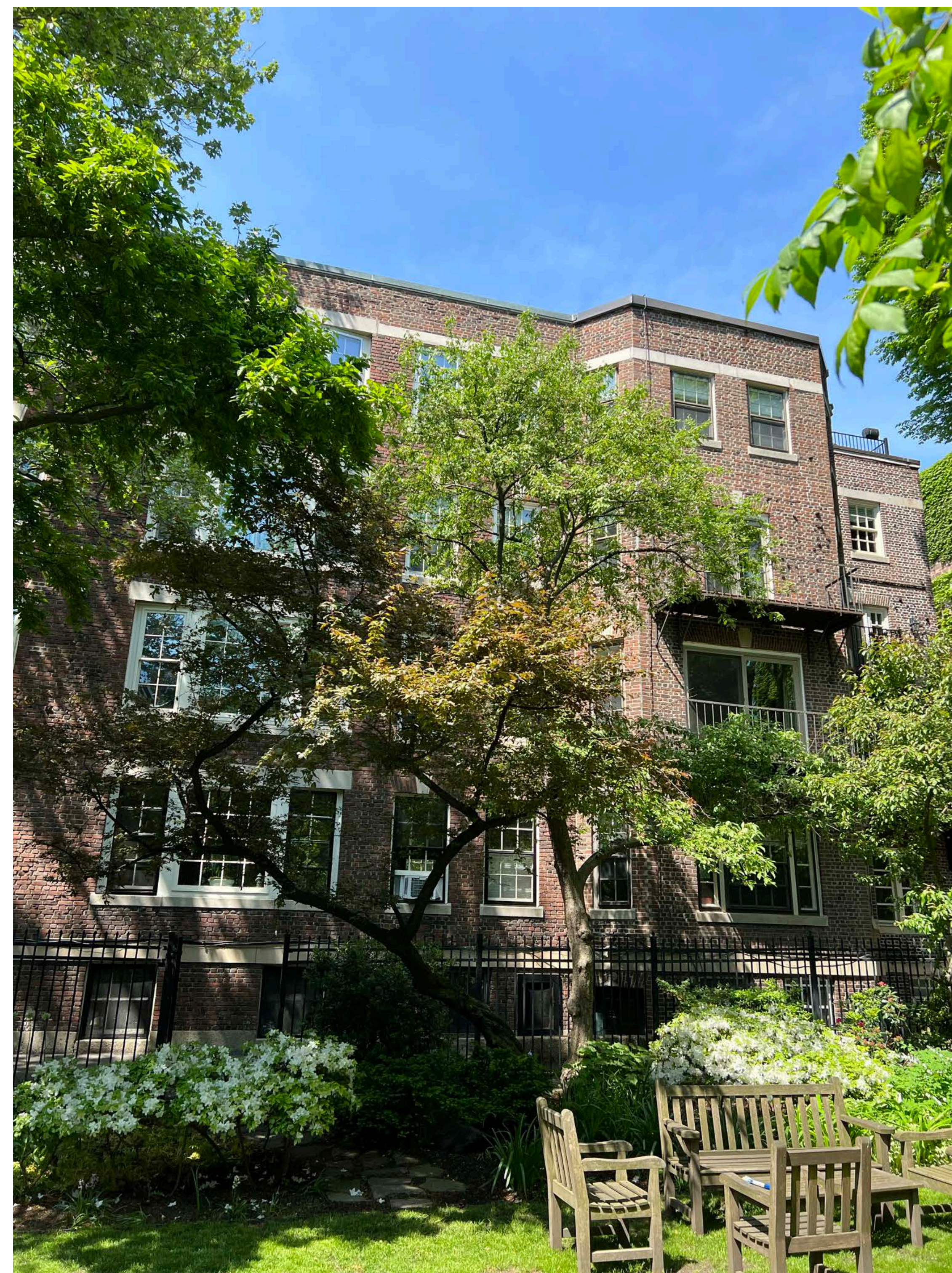
REAR ELEVATION OF 8 WEST HILL PLACE 5/23/2022
