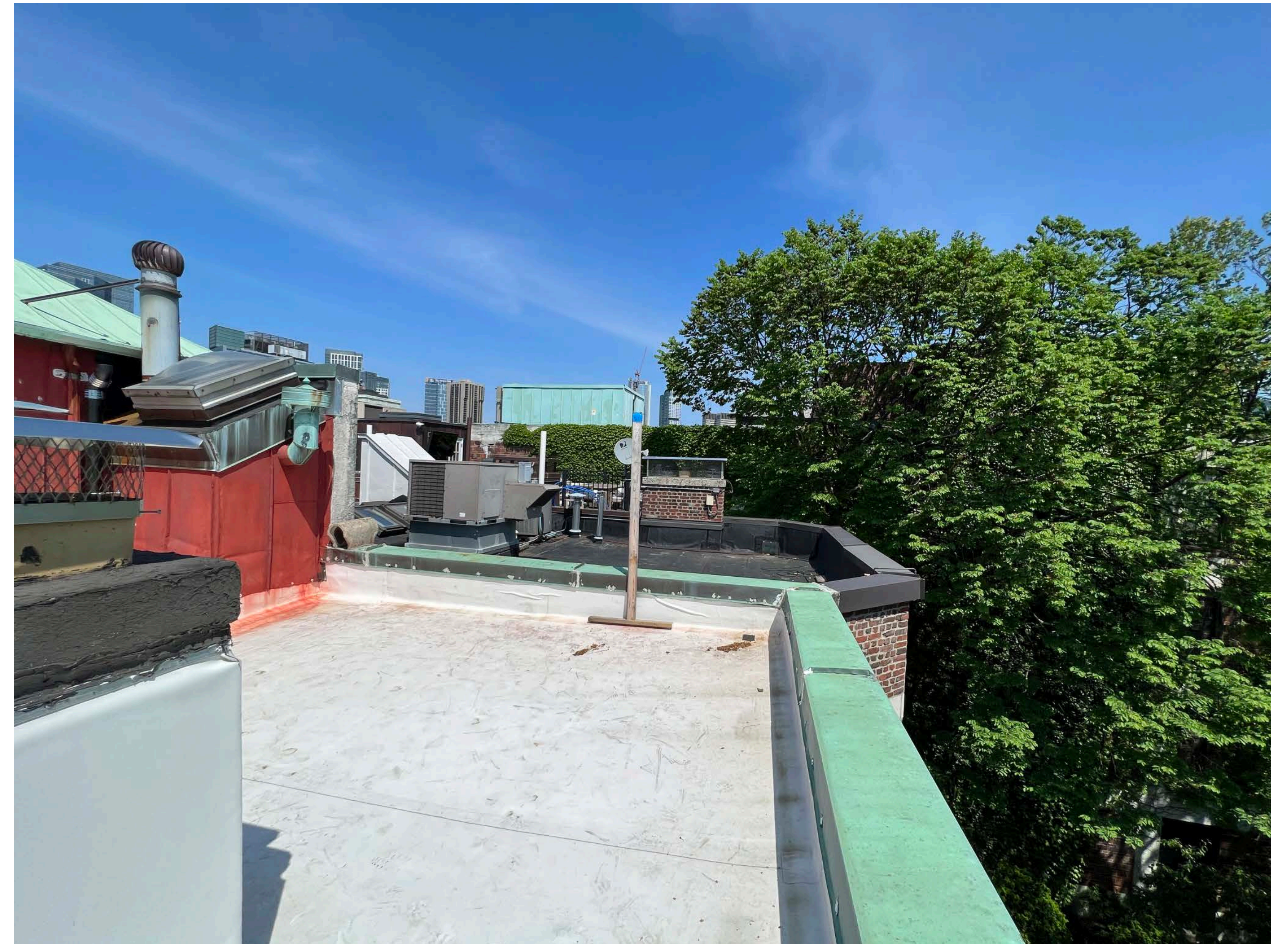
EXISTING ROOF DECK AT 8 WEST HILL PLACE
