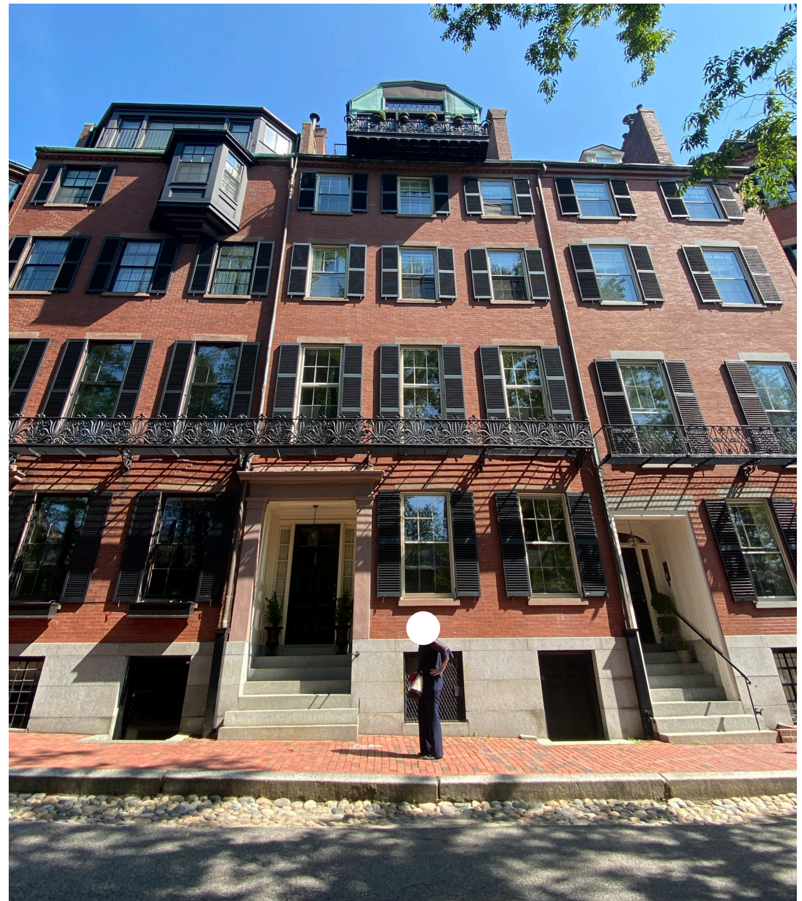
Existing sidewalk at 7 Louisburg - all existing bricks are to be re-laid after snowmelt installation
