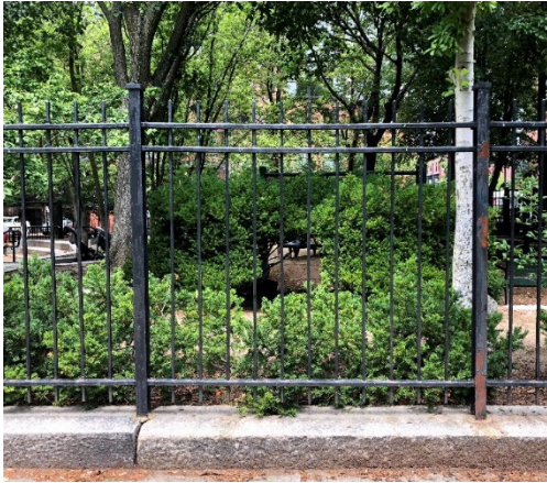
Existing Perimeter Fence
