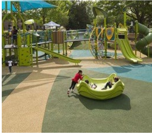
Poured-in-place (PIP) Rubber Surfacing
