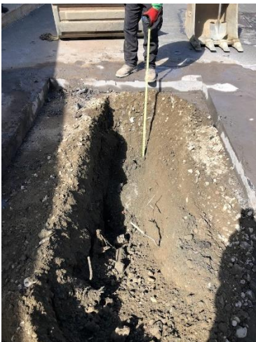
Excavated test pit
