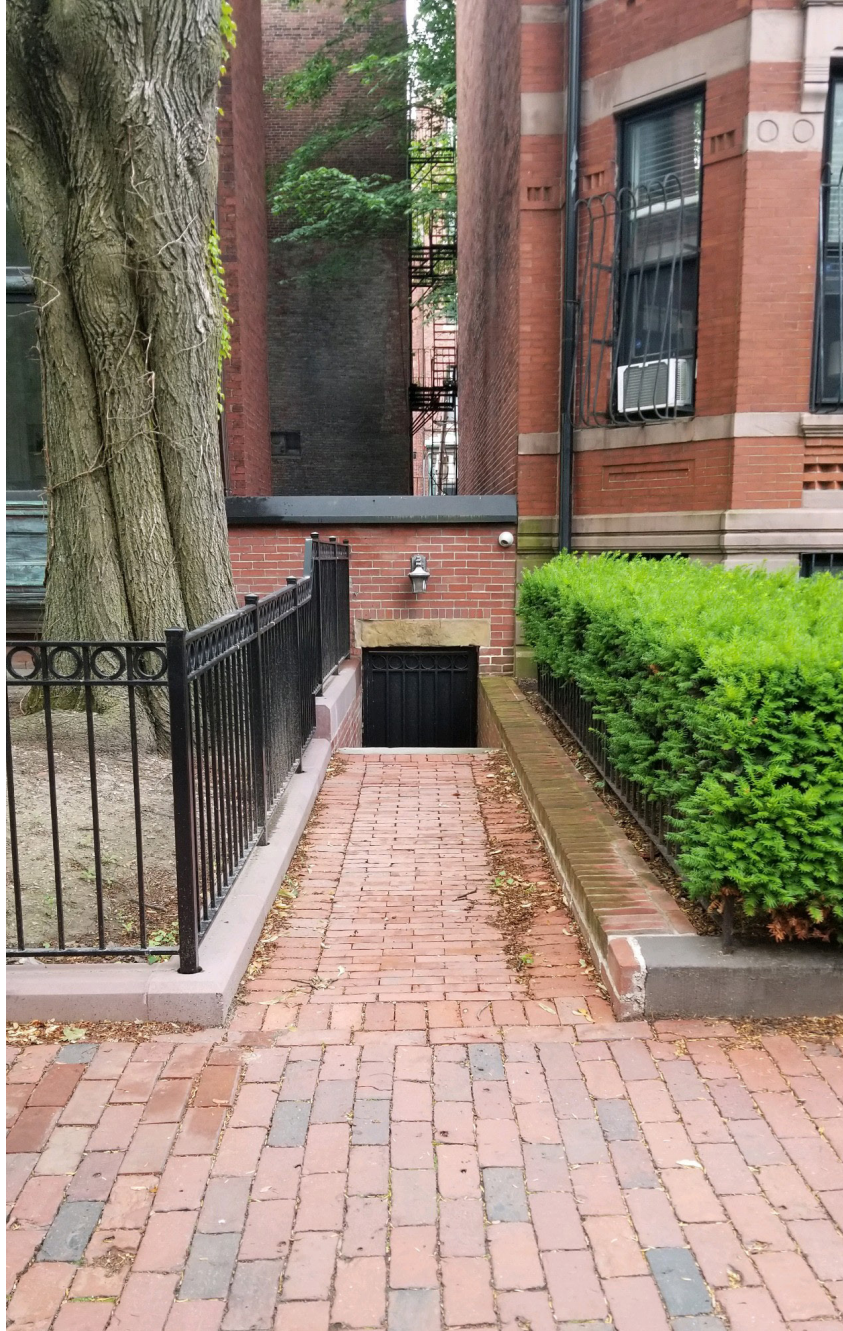
Gate Location at Side Entrance
