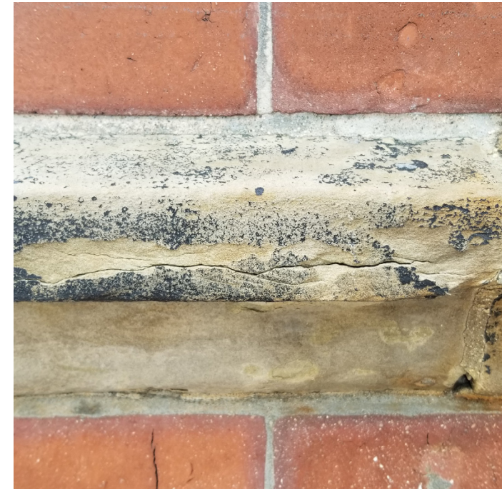
Existing Architrave Detail
