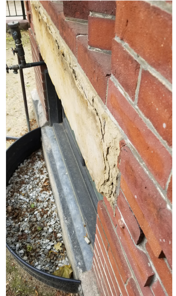
Existing Trim Detail
