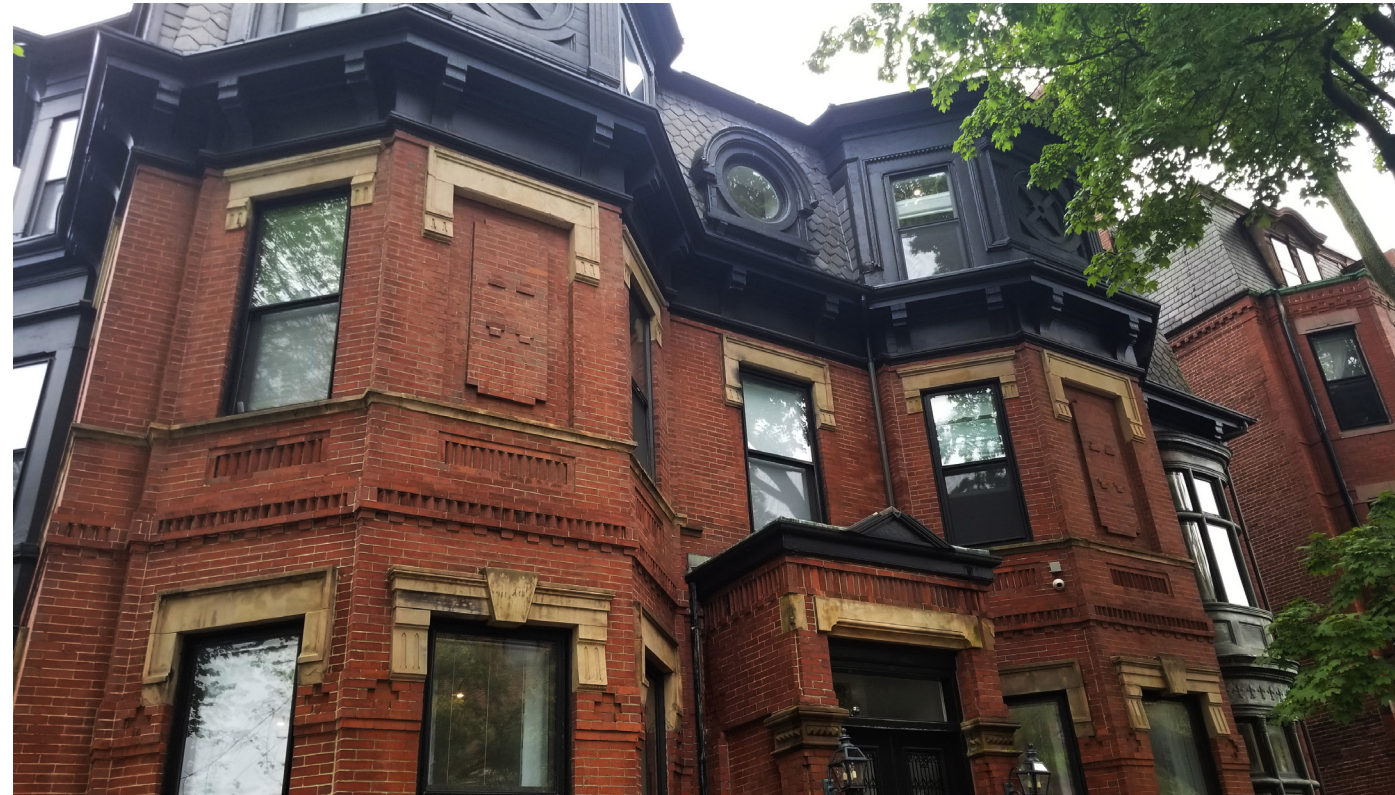
Existing Architraves and Trim on House Facade
