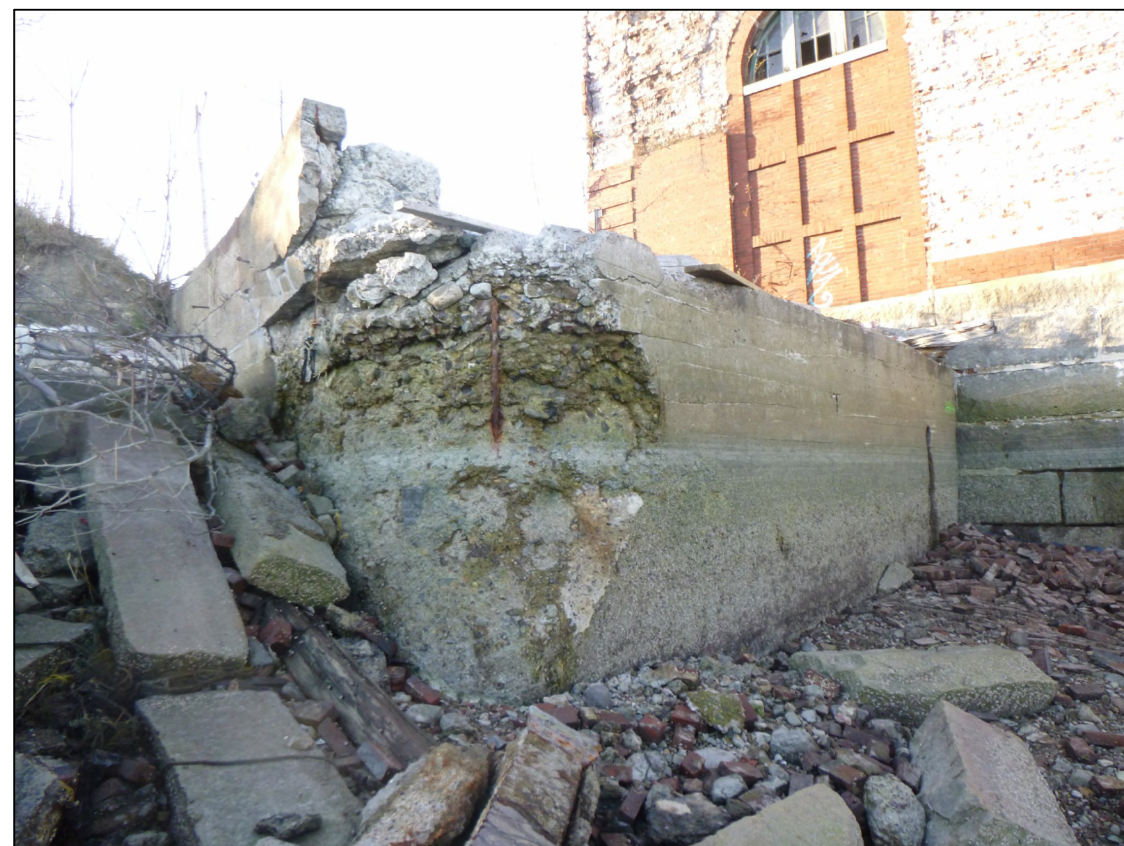
PHOTO 11: CONCRETE RETAINING WALL ON THE EAST SIDE OF THE BUILDING
