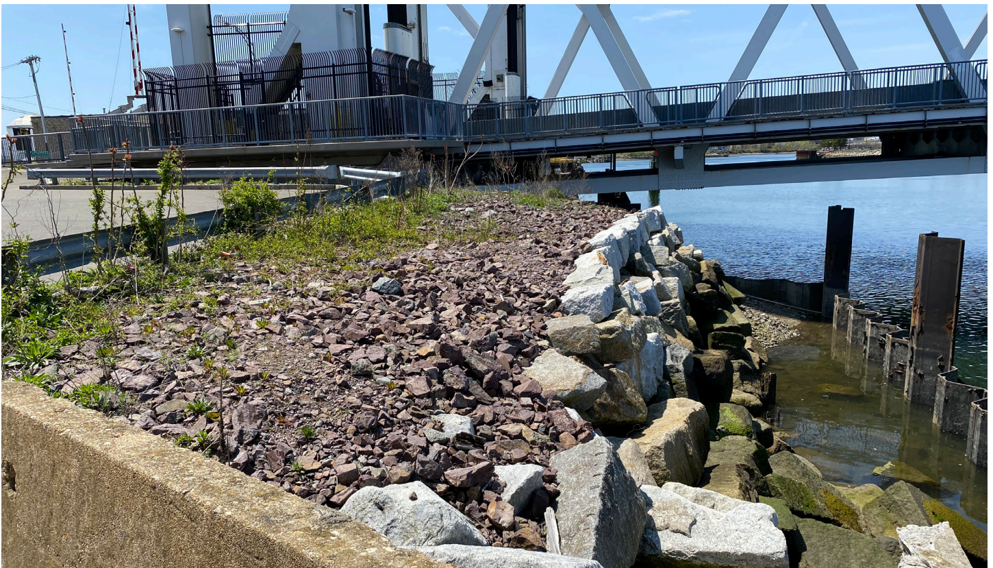
Photograph 4: Looking west towards Chelsea Street Bridge at sheetpile and seawall
