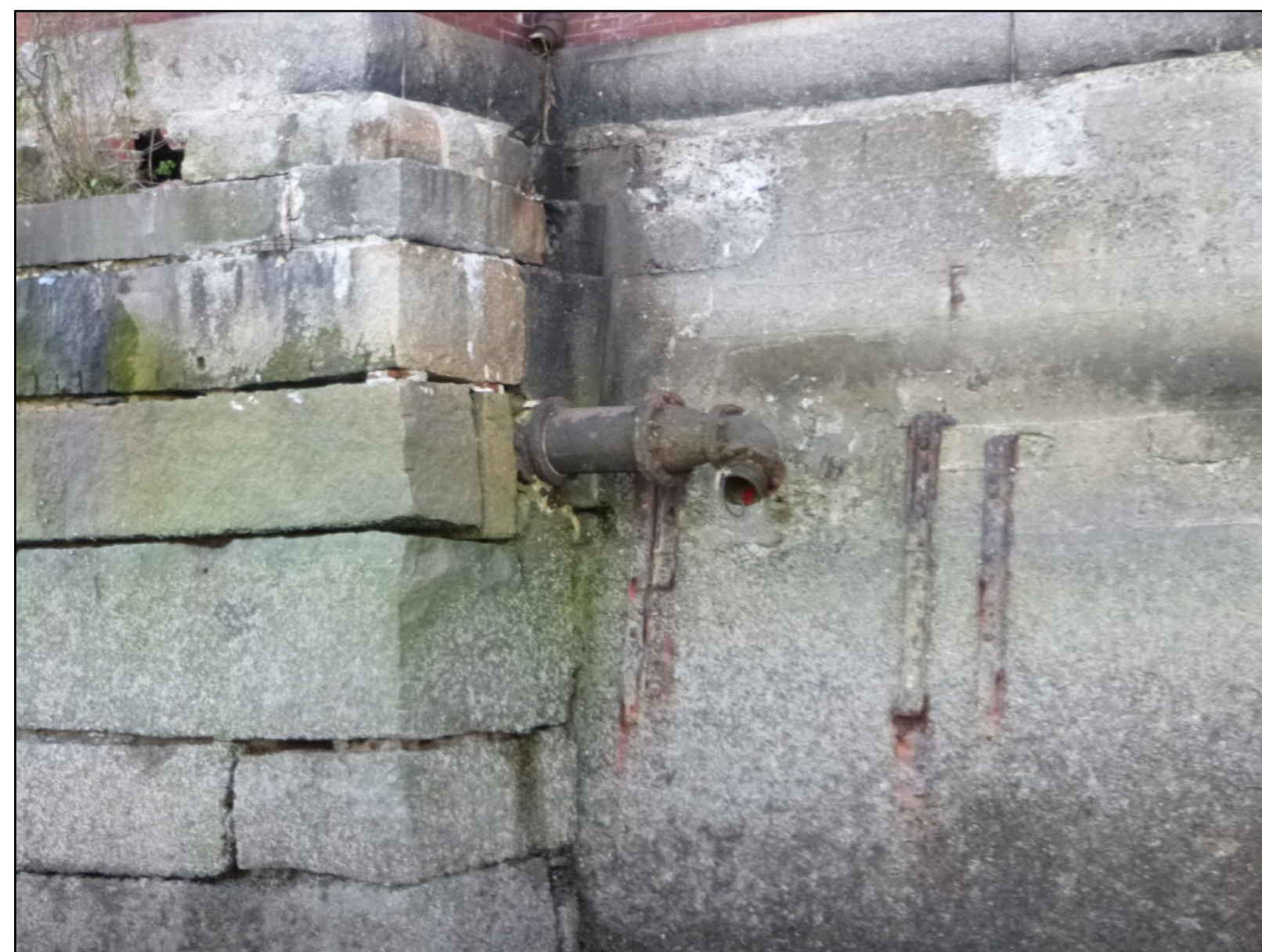
PHOTO 10: DRAINPIPE EXTENDING OUT OF SEAWALL
