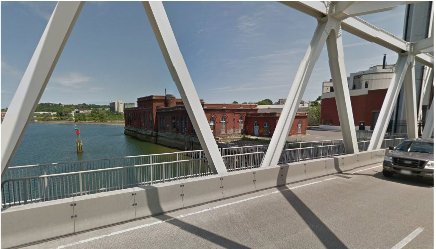
Photograph 3: Looking east at the Project Site from Chelsea Street Bridge
