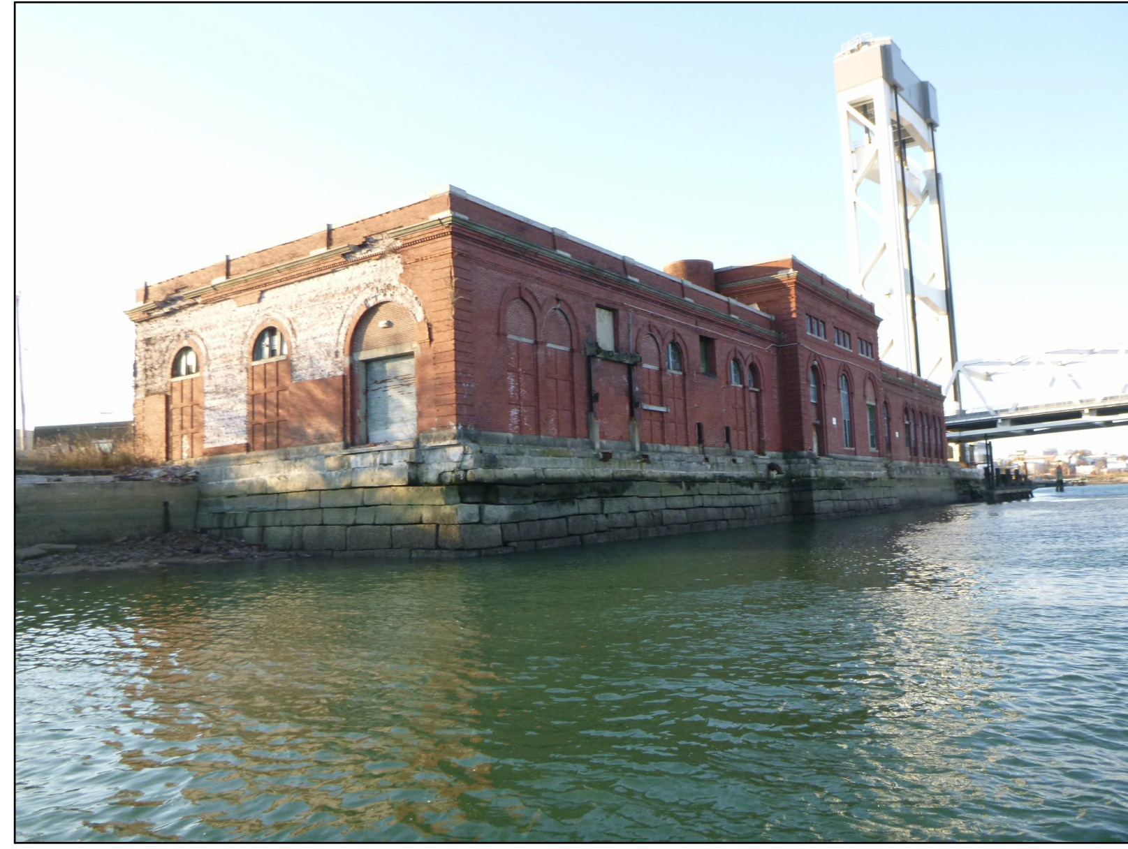
PHOTO 1: OUTSHORE VIEW OF THE NORTHEAST CORNER
