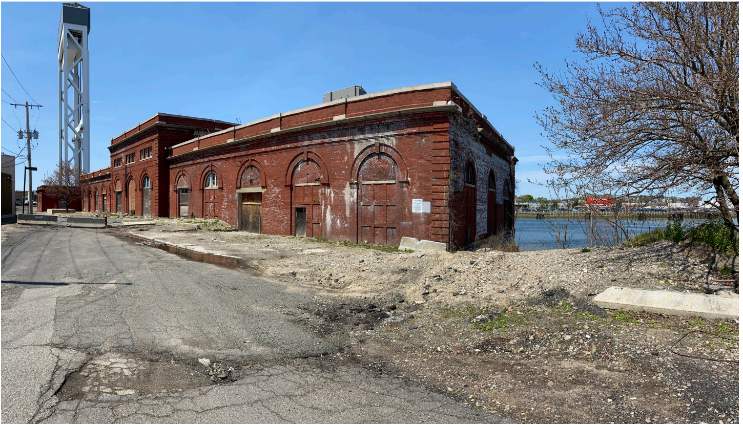
Photograph 1: Looking west at the Pump Station
