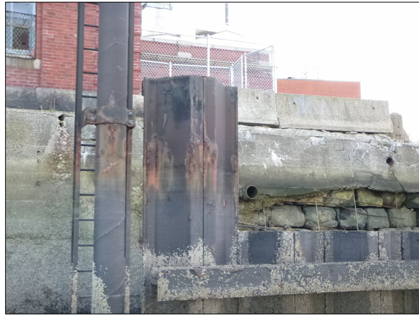
PHOTO 5: BRIDGE NAVIGATIONAL AID STRUCTURE
