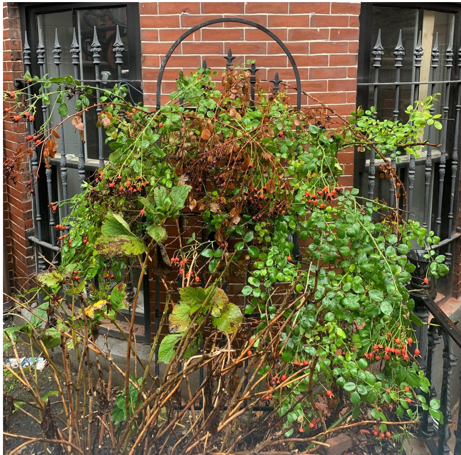
Existing Conditon- At lower level in bay
