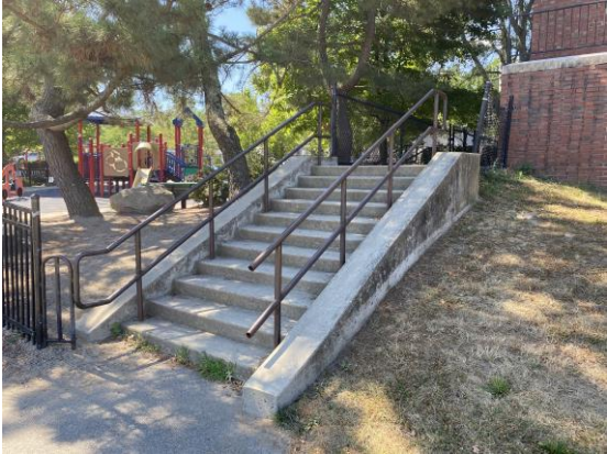
Stairs to Existing Building
