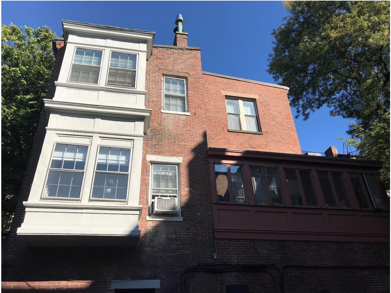
9.) View of rear elevation of 44 Chestnut Street from Branch Street
