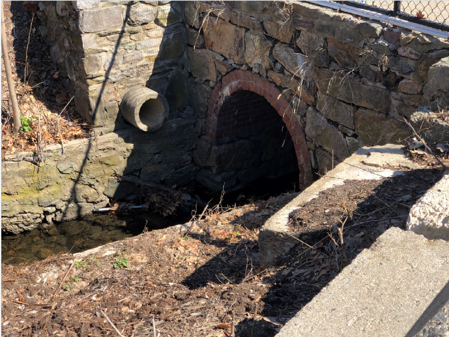
Photo 3. Bussey Brook Culvert (West Side)
