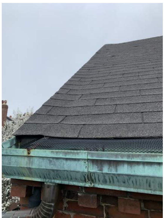
EXISTING COPPER GUTTER
