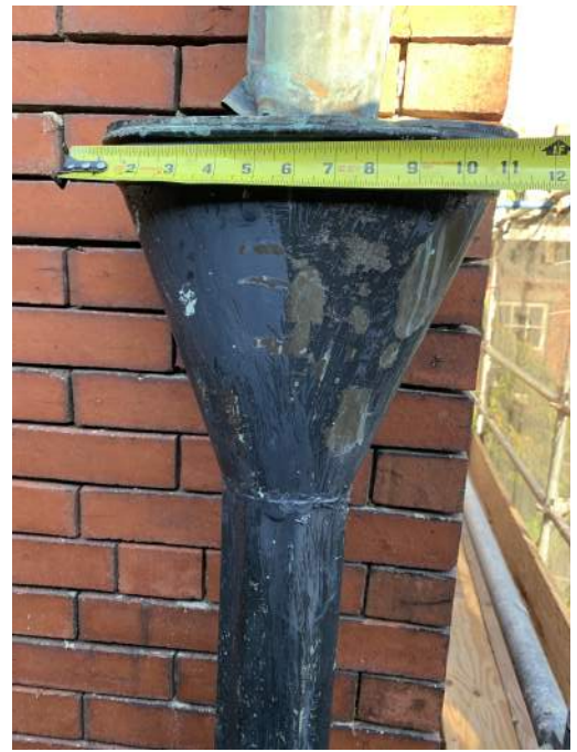
EXISTING GUTTER CONDUCTOR
