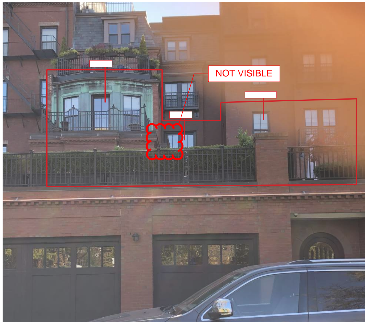
B. NORTH FACADE - PROPOSED WORK TO UNIT G (SECOND FLOOR LEVEL, BACK STREET SIDE)
