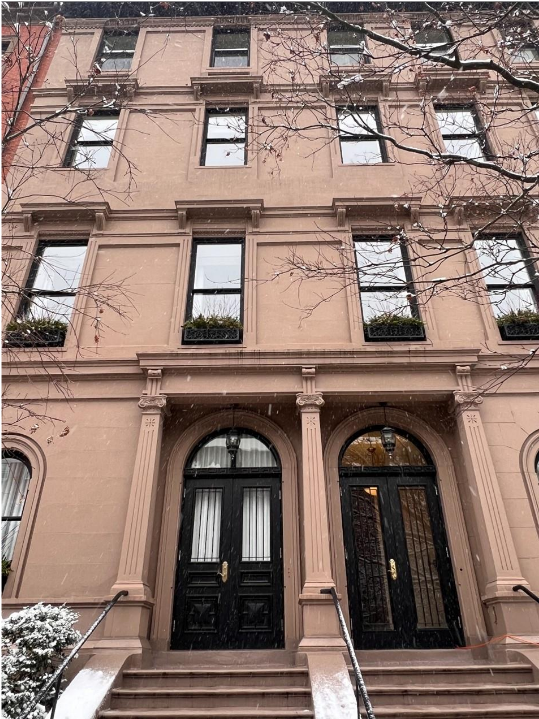
Across the Street from 122 Beacon Street
