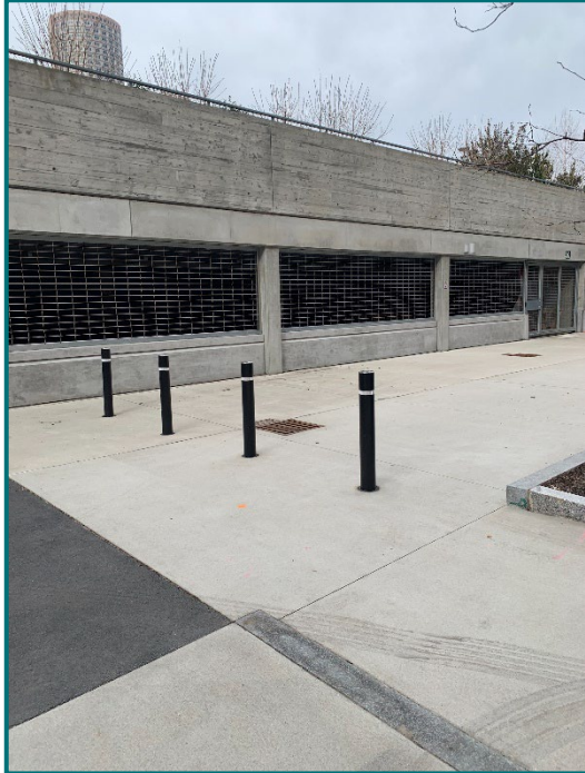
Representative bollards within public ROW on Sleeper Street.
