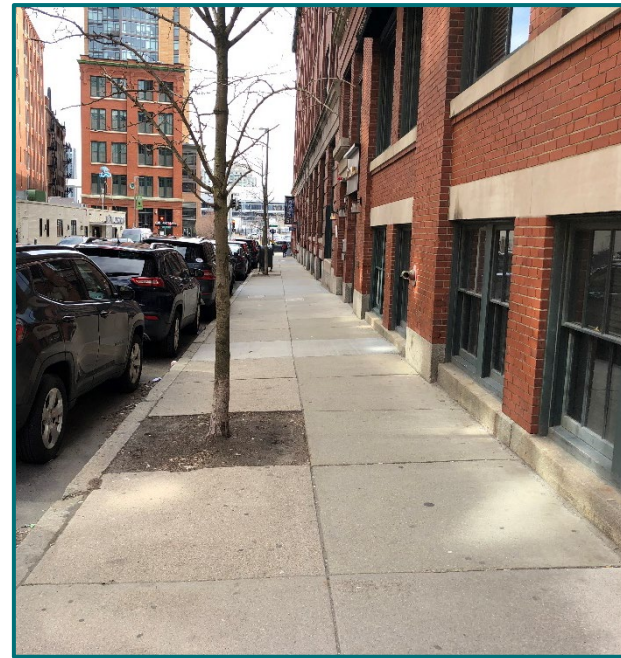
Existing Melcher Street tree pits.
