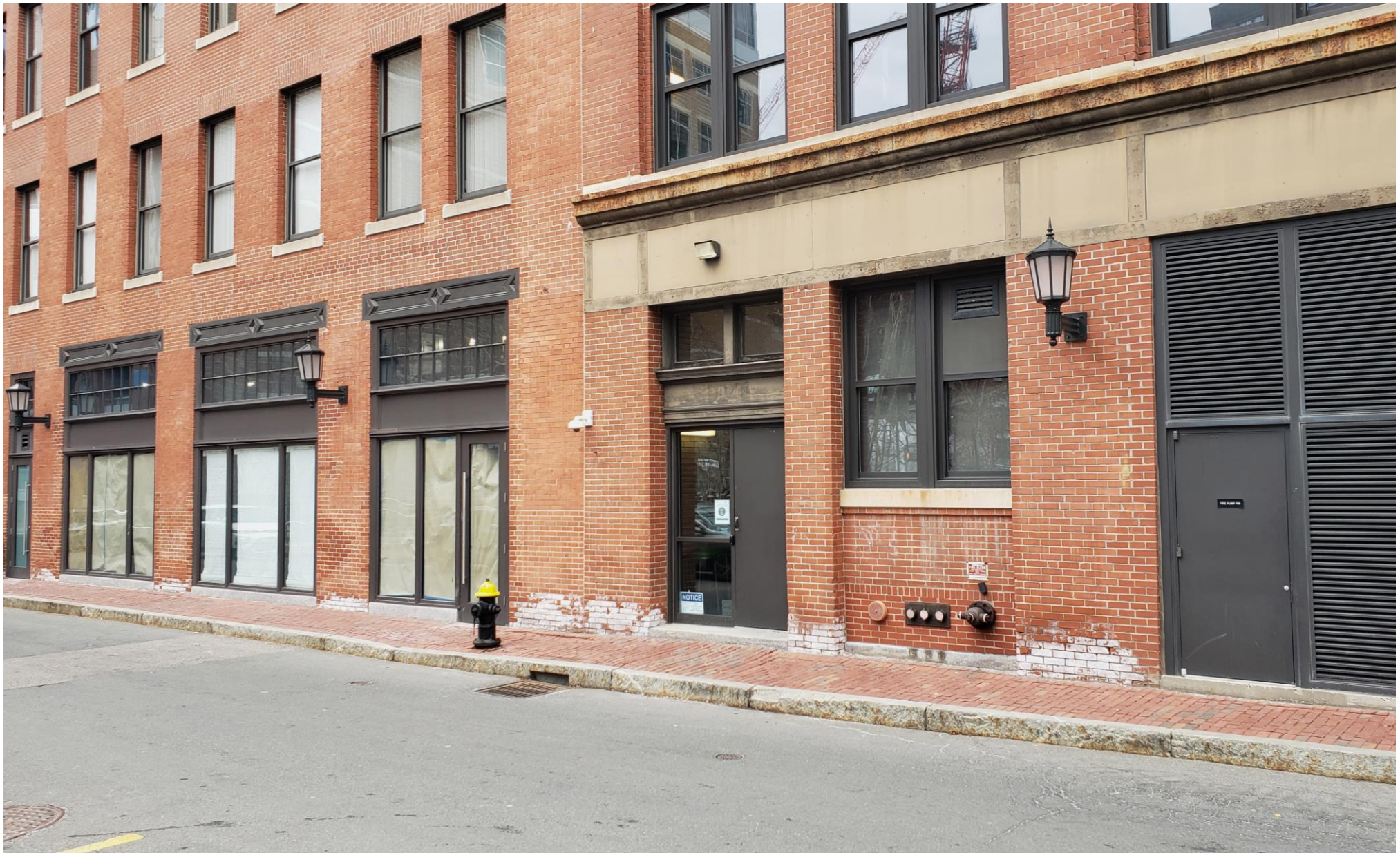
EXISTING CONDITION PHOTO
