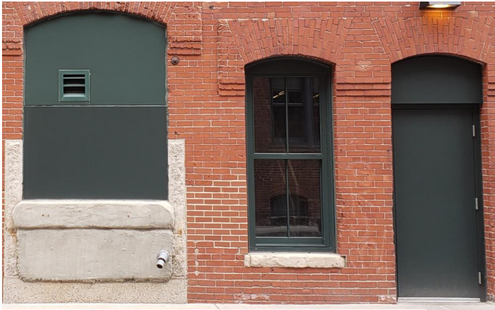
RESIDENCE INN - VENT DETAIL ON THOMSON PLACE
