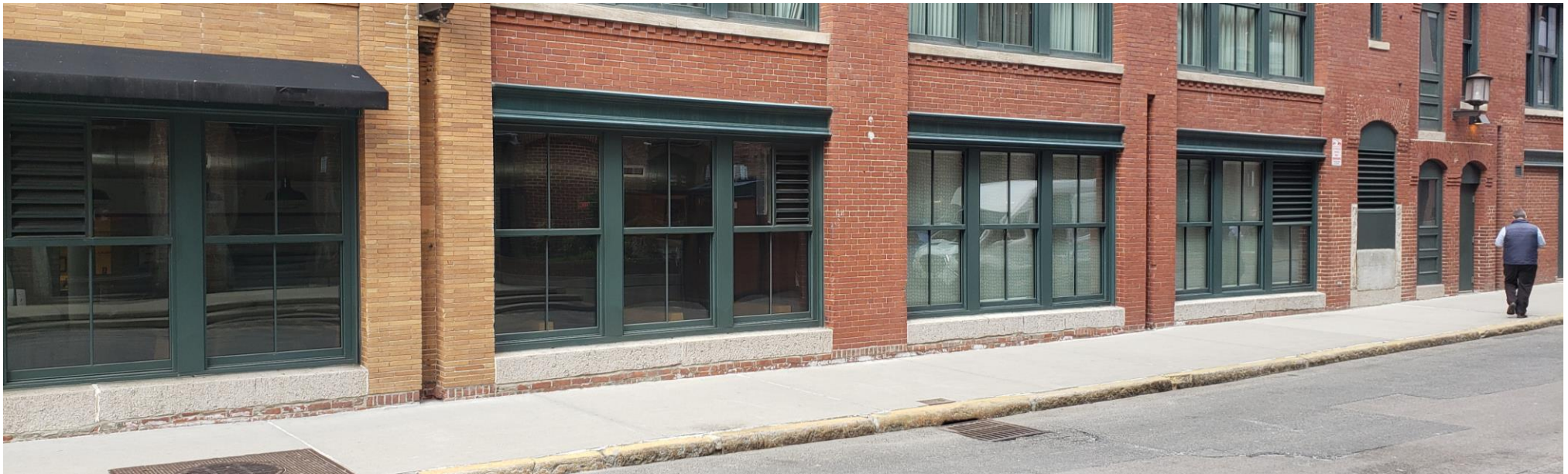
RESIDENCE INN - VENT DETAIL ON STILLINGS STREET
