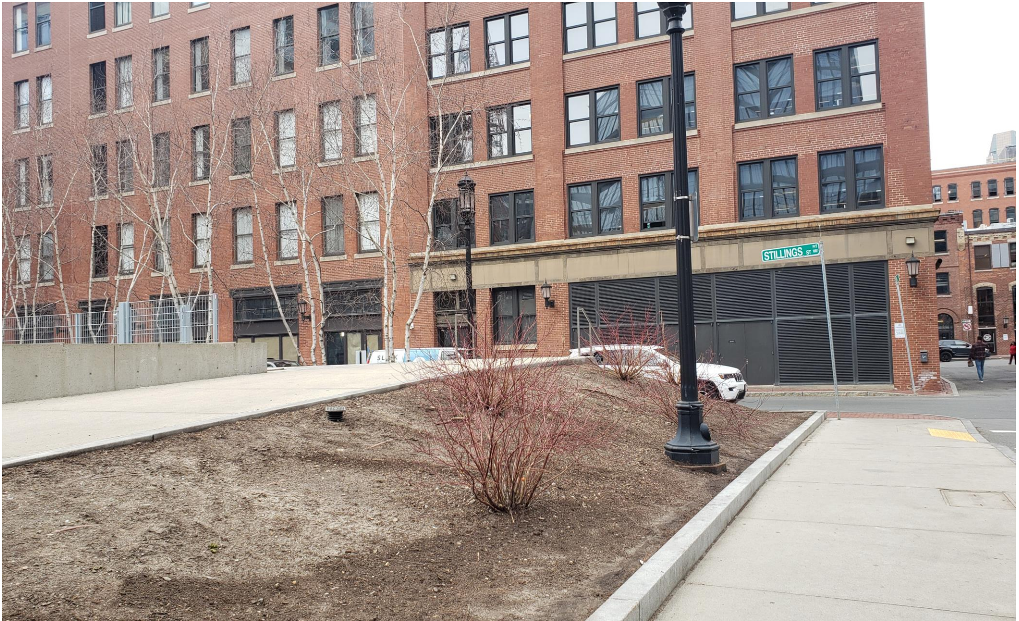
EXISTING CONDITION PHOTO
