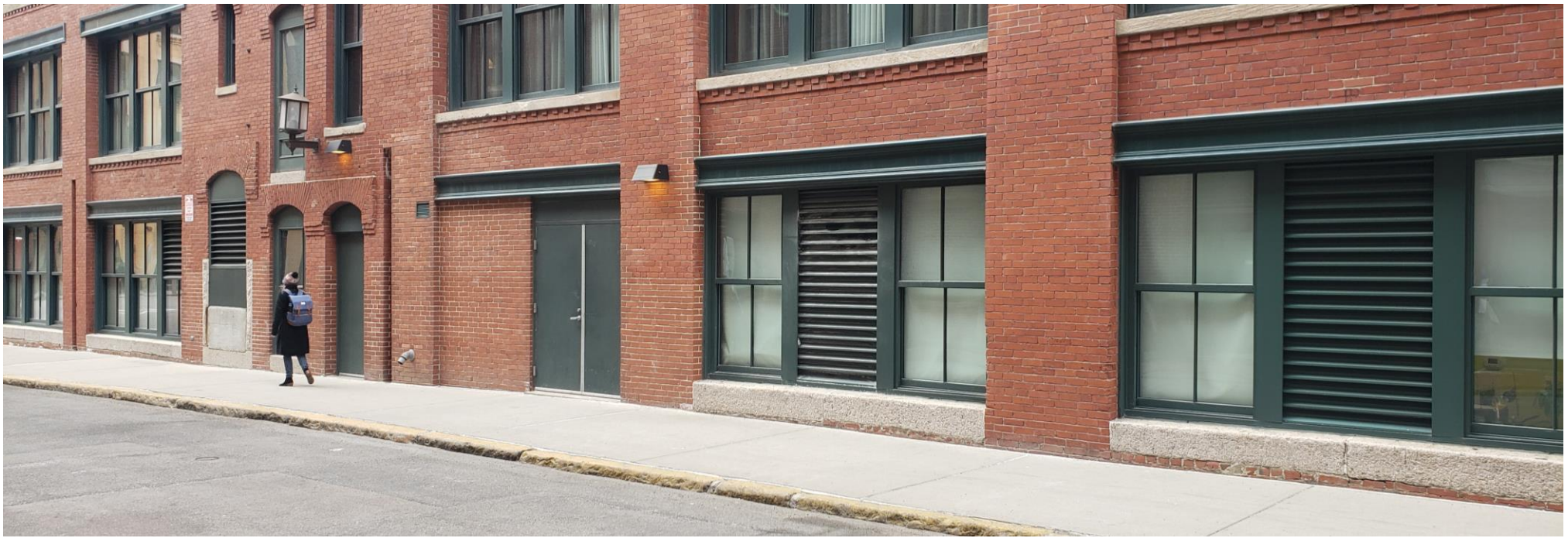
RESIDENCE INN - VENT DETAIL ON STILLINGS STREET
