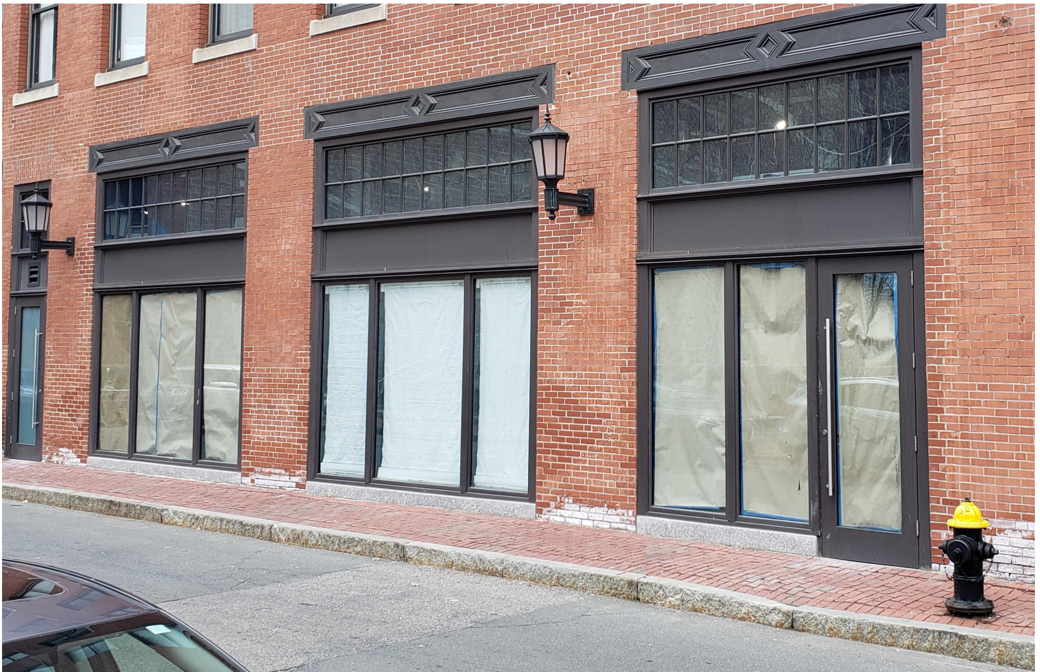
EXISTING CONDITION PHOTO
