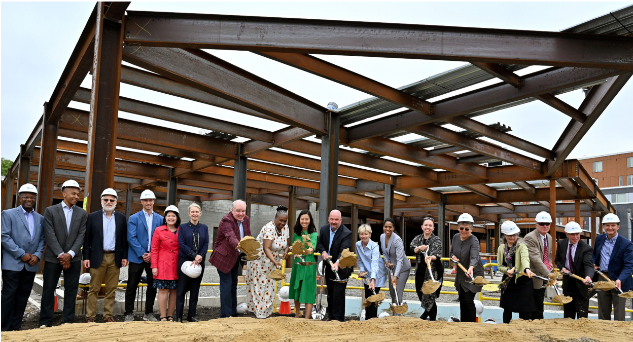
The groundbreaking event for J.J. Carroll Redevelopment in Brighton, a 142-unit affordable housing community for seniors.
