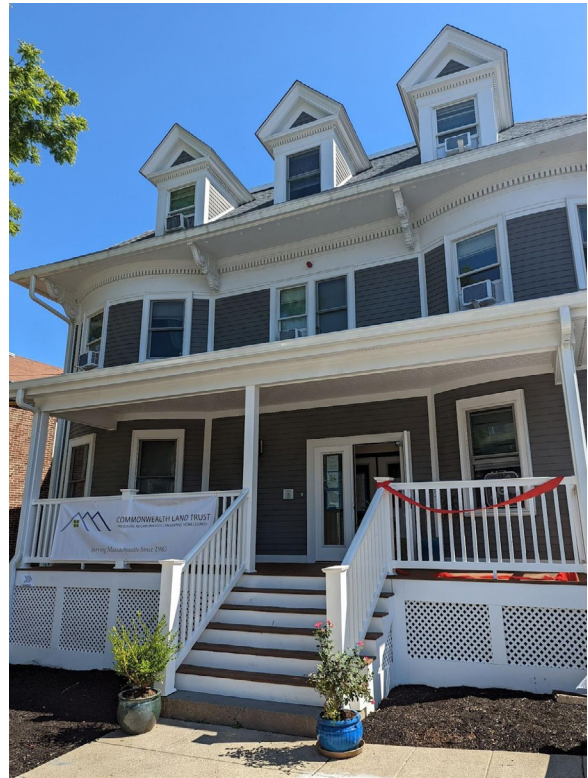
123 Crawford Street in Roxbury is a Single Room Occupancy (SRO) building that provides housing to low- and very low-income individuals who benefit most from onsite case management support and a live-in staff person.
